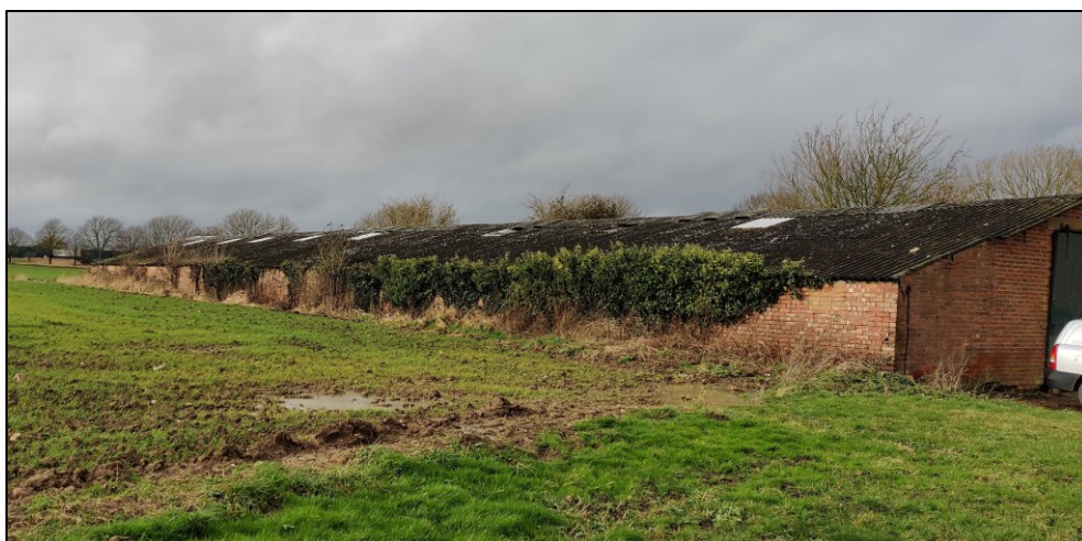
Figure 3.1 - Existing Barn View from South
