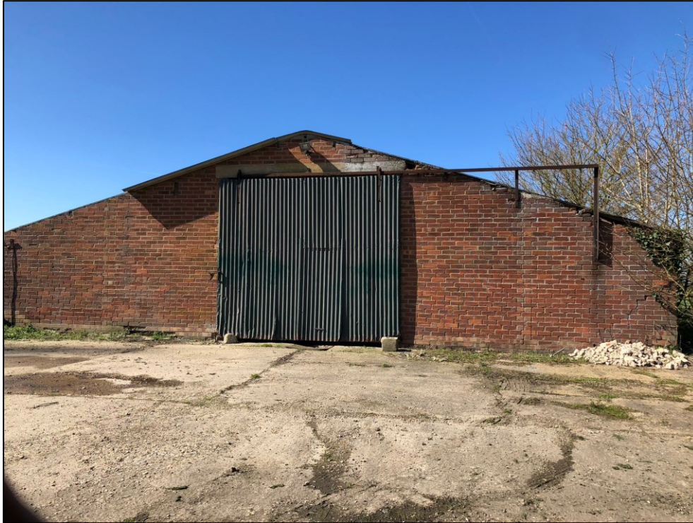
Figure 2.2 - Existing Barn East (Front) Elevation
