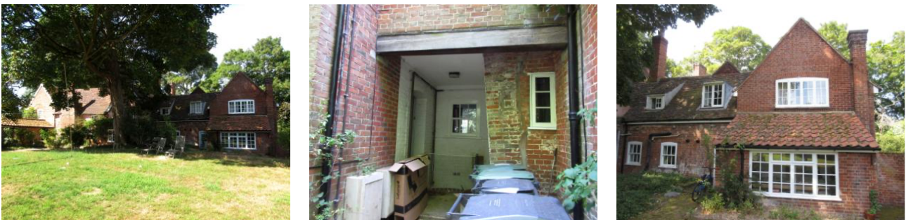
Left: East (rear) elevation; Centre: West elevation showing recess on West side of cottage with 20th century timber lintel and brickwork, West wall of cottage (white render) visible inside recess; Right: North elements of east elevation showing cottage with cat-slide and flat roofed dormers, and 20th century red brick annexe.
