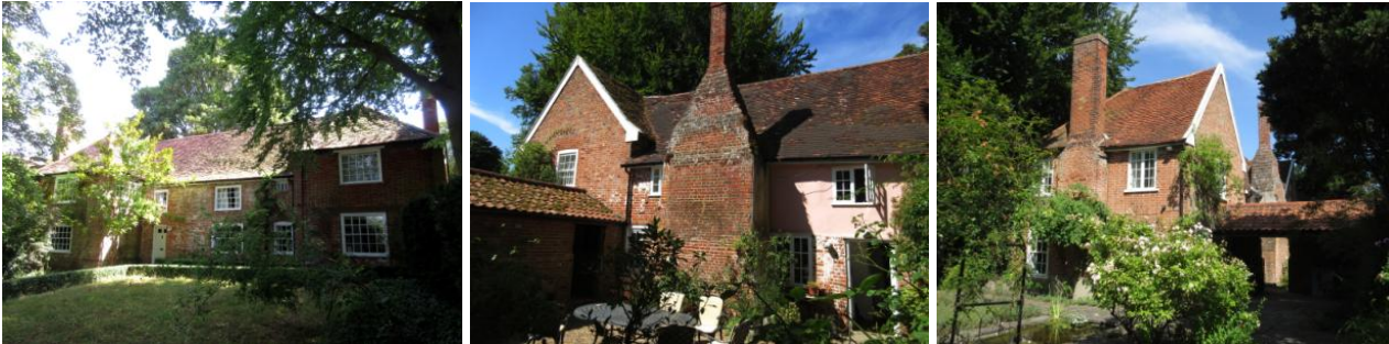
Left: principal West elevation showing hipped cross wings; Centre: East elevation of South cross wing and hall with 16th century external stack; Right: looking NW, showing stack against South wall.
