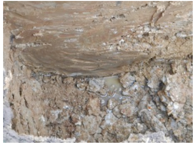
photo to right: flinty pocket giving rise to water ingress
