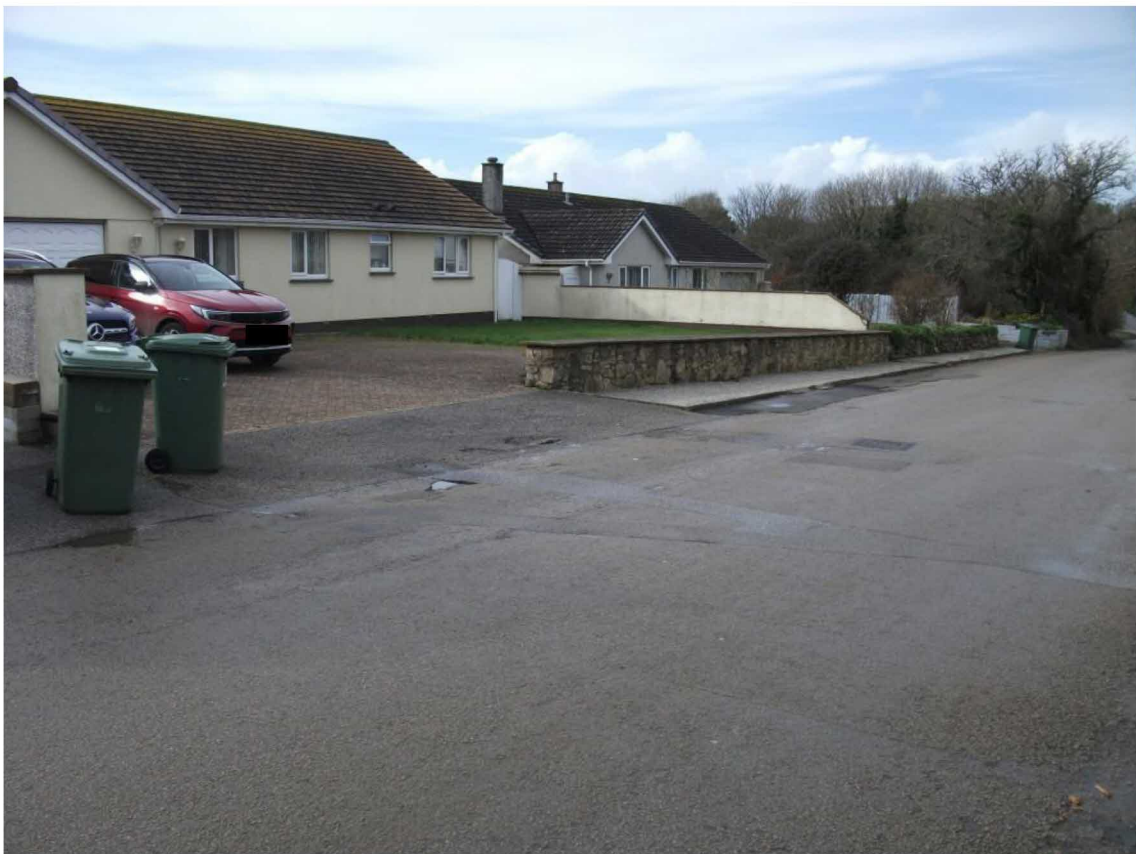
Photo # 4 – Access facing NW view of Bungalow
