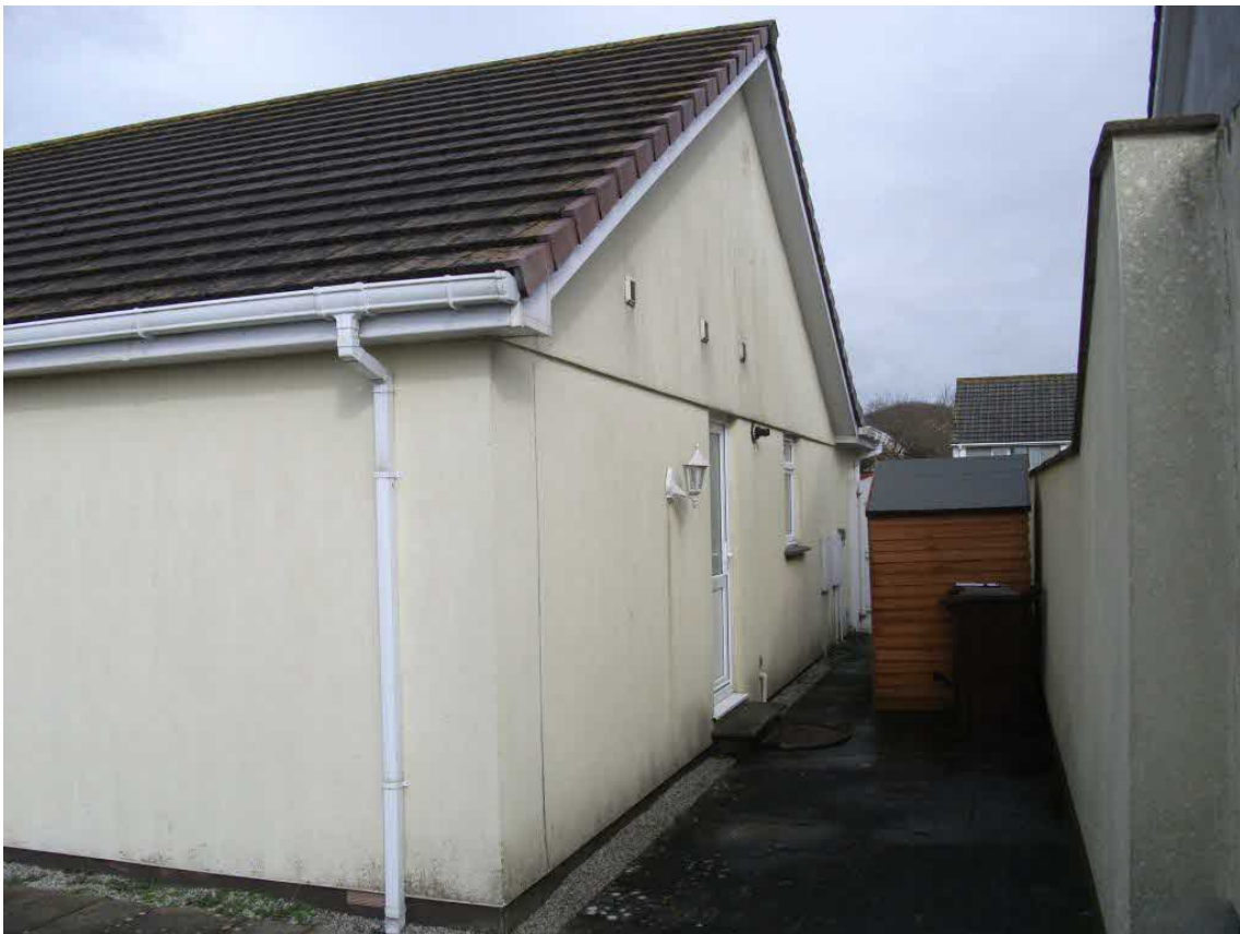
Photo # 16 – Side view of Bungalow (adjacent to No. 7)
