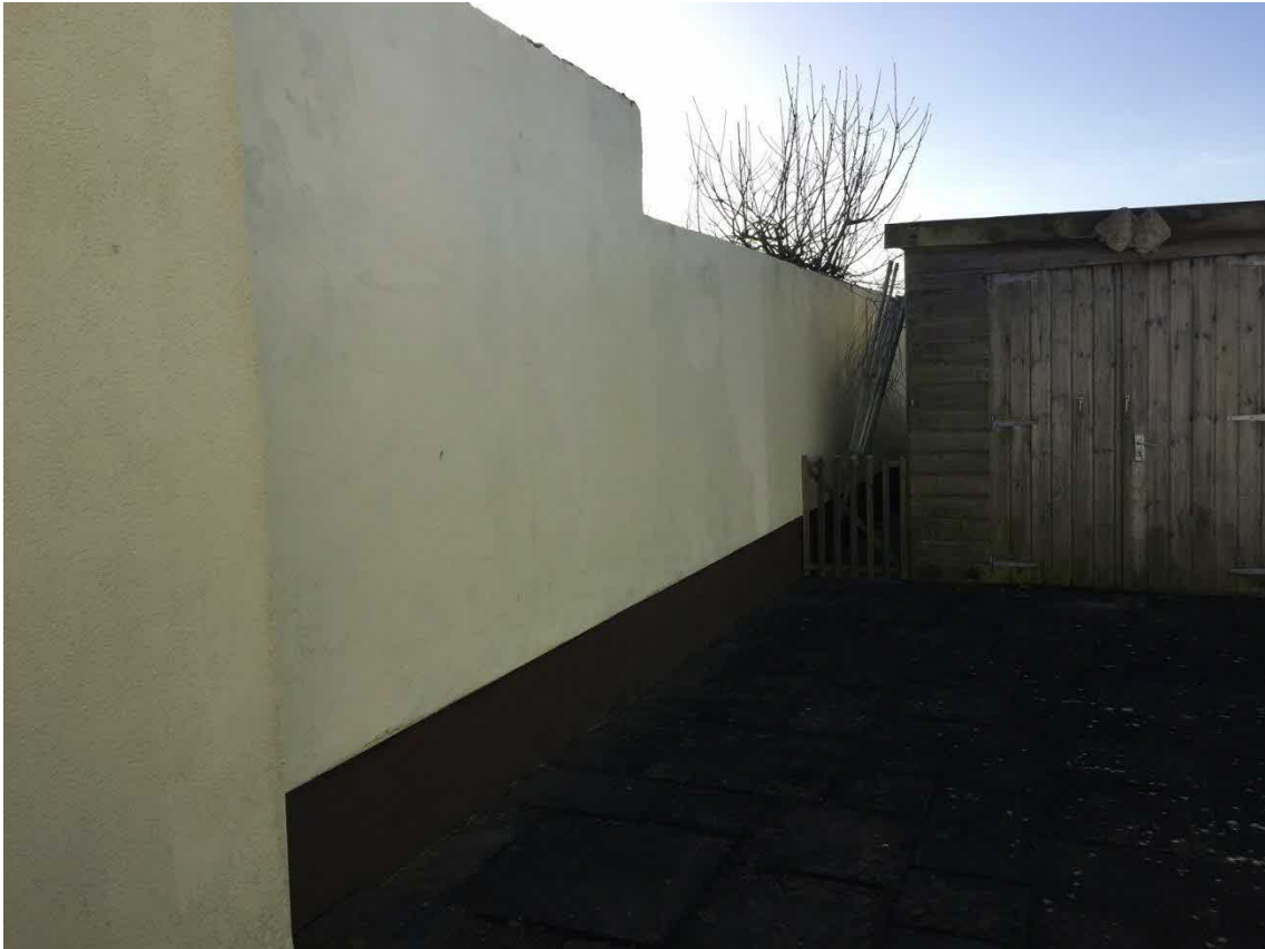
Photo # 13– Rear SE Boundary (adjacent to neighbour at No. 7)
