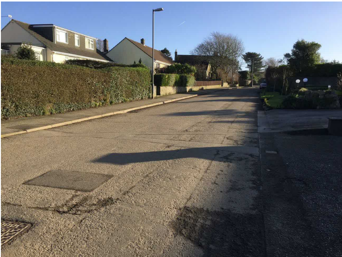
Photo # 2 – South Facing View on Relistian Lane
