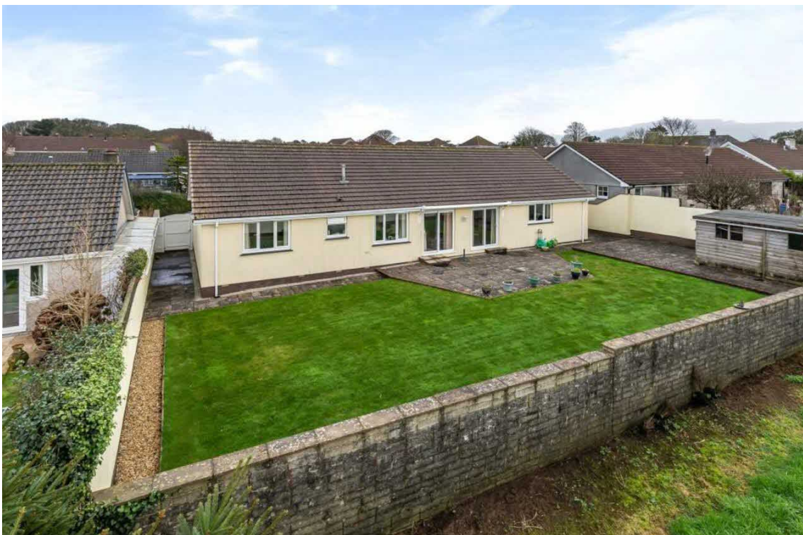
Photo # 8 – Rear of Bungalow
