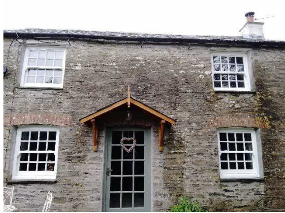
Photograph 2 – View of the south aspect of the cottage.
