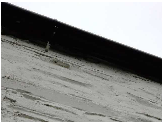
Photograph 5 – View of the sealed eaves of the cottage roof.
