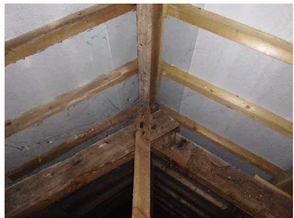
Photograph 6 – View of the void roof structure.
