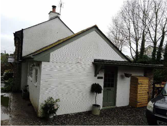
Photograph 1 – View of the east aspect.
