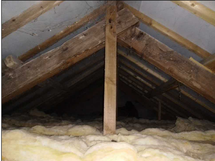
Photograph 2 – View of the internal void.
