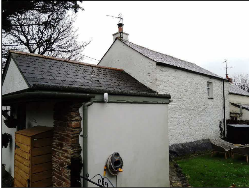
Photograph 1 – View of the north aspect.
