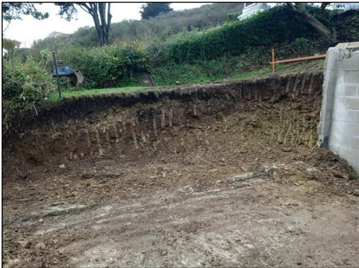
Excavation for new garage 09/02/2024
