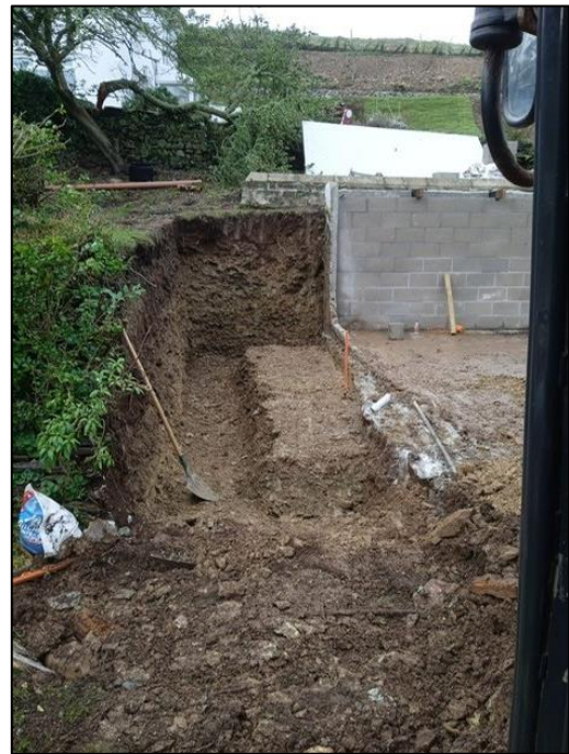
Footings for new garage 10/02/2024
