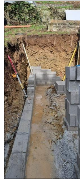
First blockwork for new garage under construction – 01/03/2024
