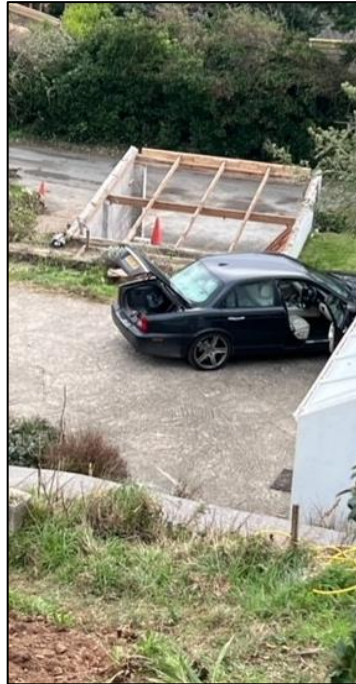
Asbestos roof removed – 17/01/2024
