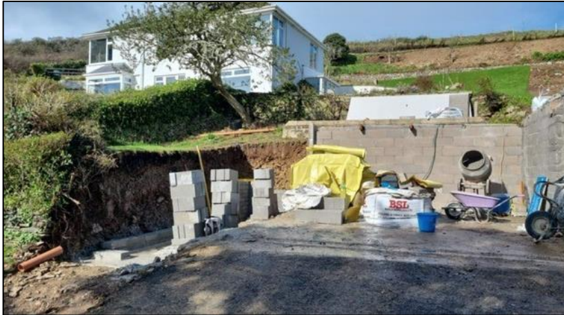
First blockwork for new garage under construction – 01/03/2024
