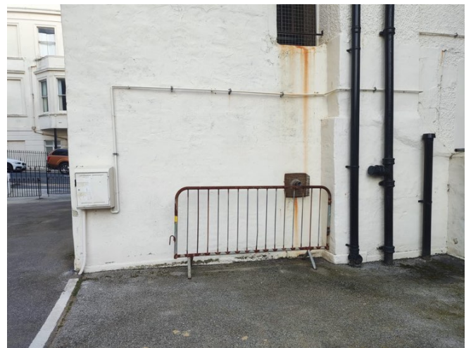
4 Existing gas meter and pipework
