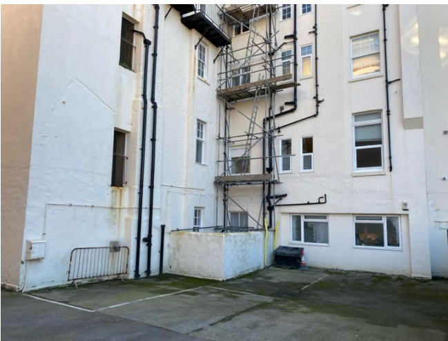
3 Rear elevations with existing gas meter and pipework
