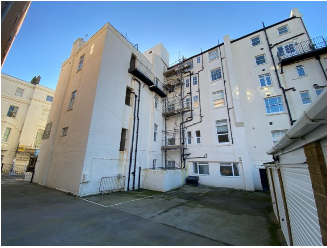
1 Rear elevations to Bristol Court across carpark
