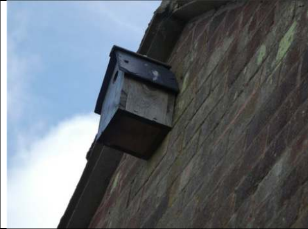
Photograph 19. Example of a nesting box on the garage
