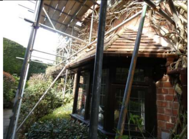
Photograph 2. The lower part of the south elevation of the house
