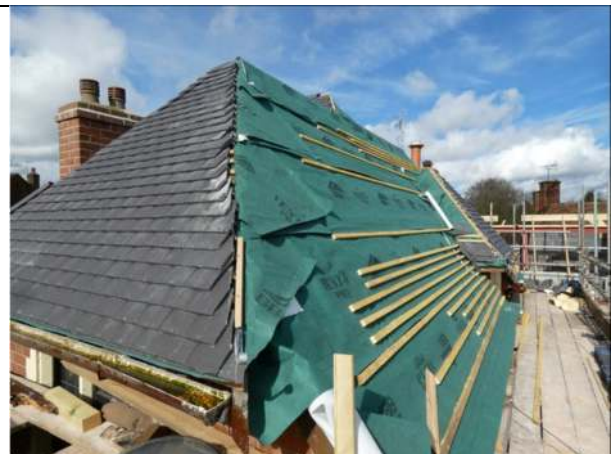
Photograph 6. Example of the south roof (re-roofing in progress)
