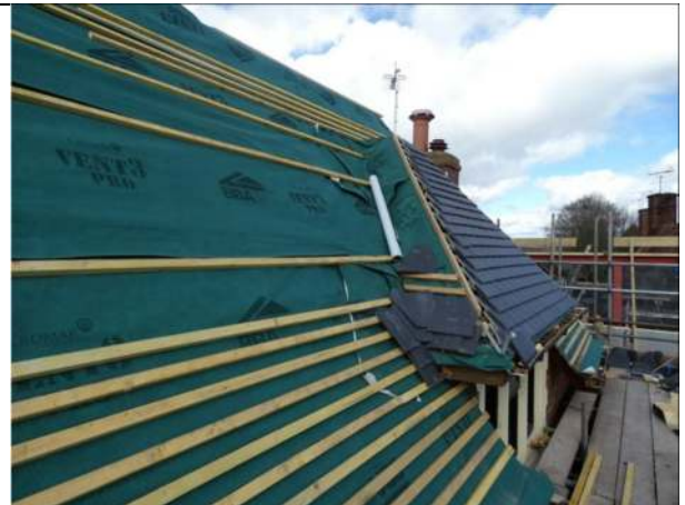
Photograph 4. Example of the east roof (re-roofing in progress)
