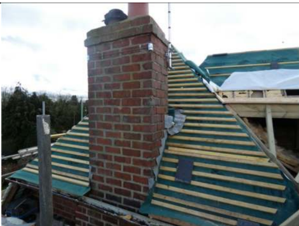
Photograph 5. Example of the north roof (re-roofing in progress)
