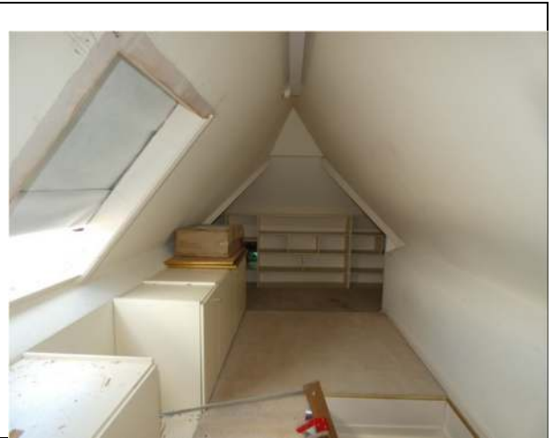
Photograph 8. The enclosed roof void the house (east-west orientated section)
