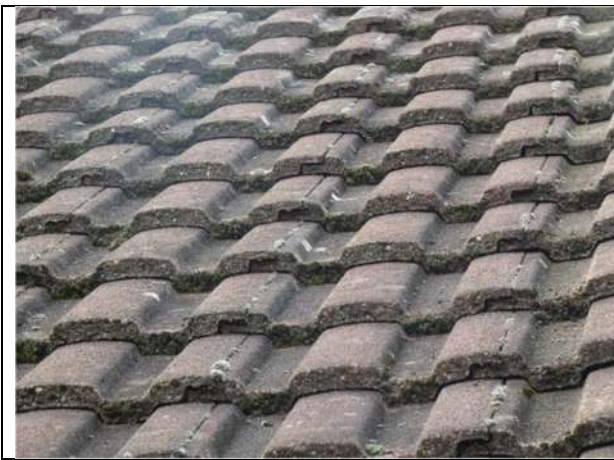
Photograph 15. Example of the tiles on the roof of the garage
