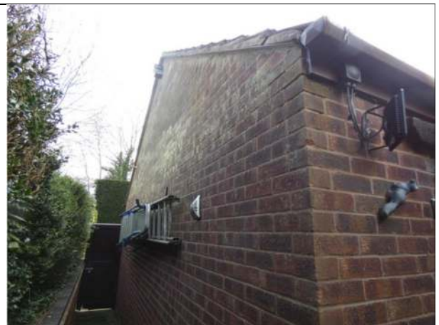
Photograph 12. The north elevation of the garage
