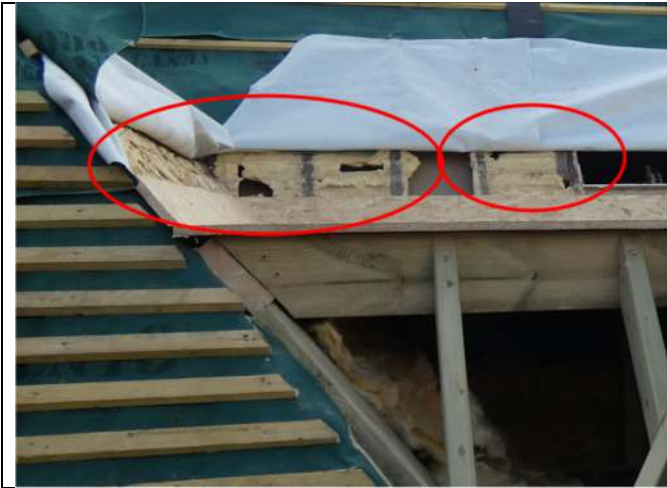
Photograph 7. Expanding foam between rafters on the previous roof on the house
