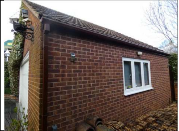
Photograph 14. The east elevation of the garage
