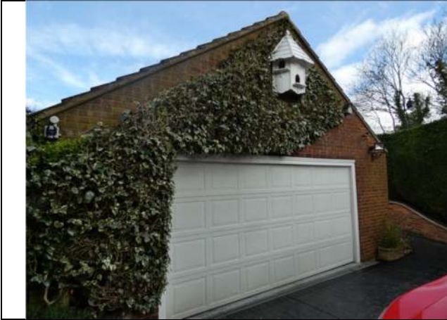
Photograph 13. The south elevation of the garage
