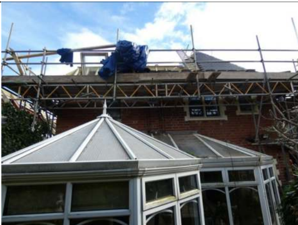
Photograph 3. The west elevation of the house
