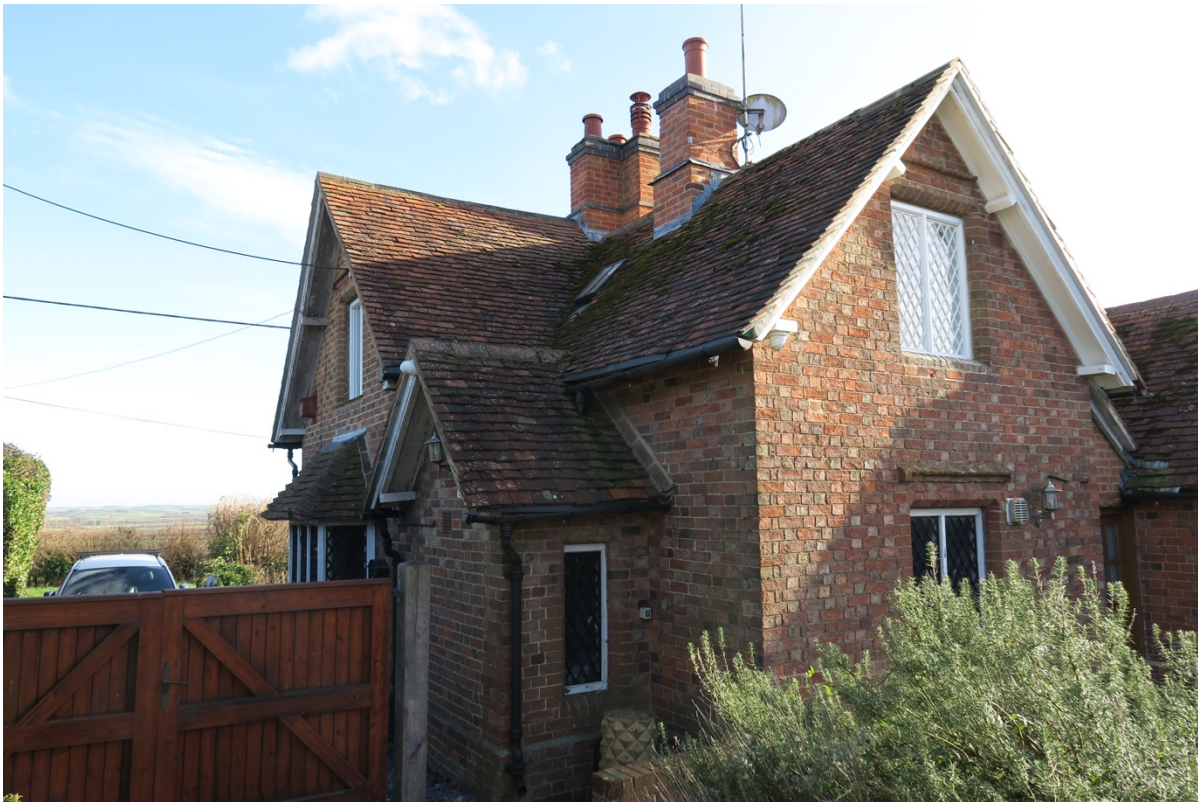
Northwest corner of the cottage showing plain clay tiles
