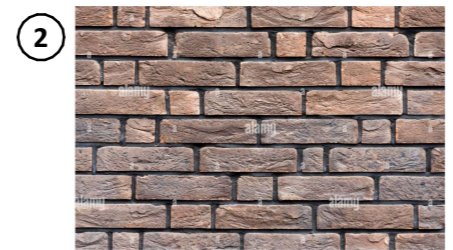
External Walls - Brown Brick Wall.
