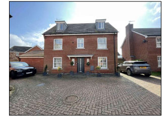
Existing frontage showing block paving
