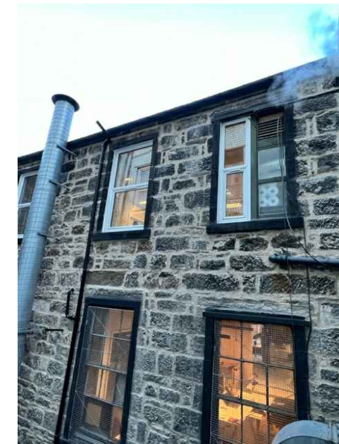
Existing Photo - Rear Elevation
