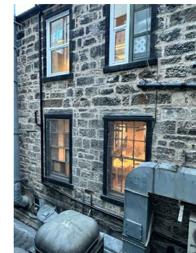
Existing Photo - Rear Elevation
