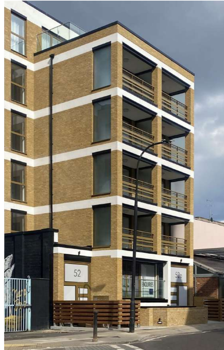
Metal Balustrade, GML Architects, Kentish Town
