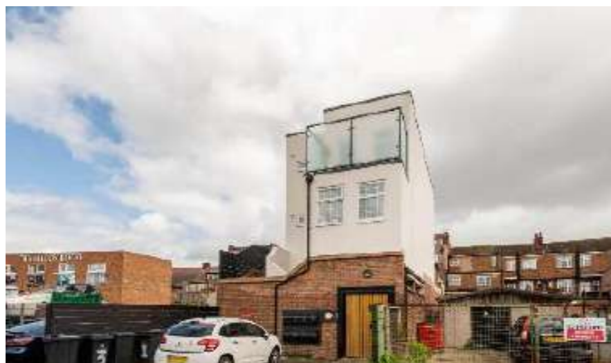
View of the new building extension, at the Burwood Close
