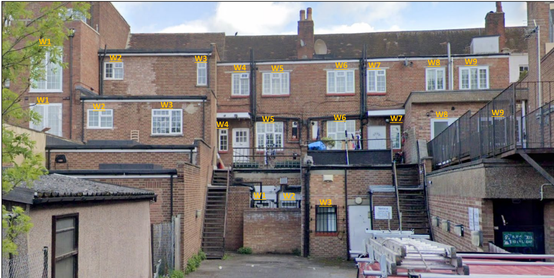
Figure 7:Rear View of 12-18 Tolworth Broadway
