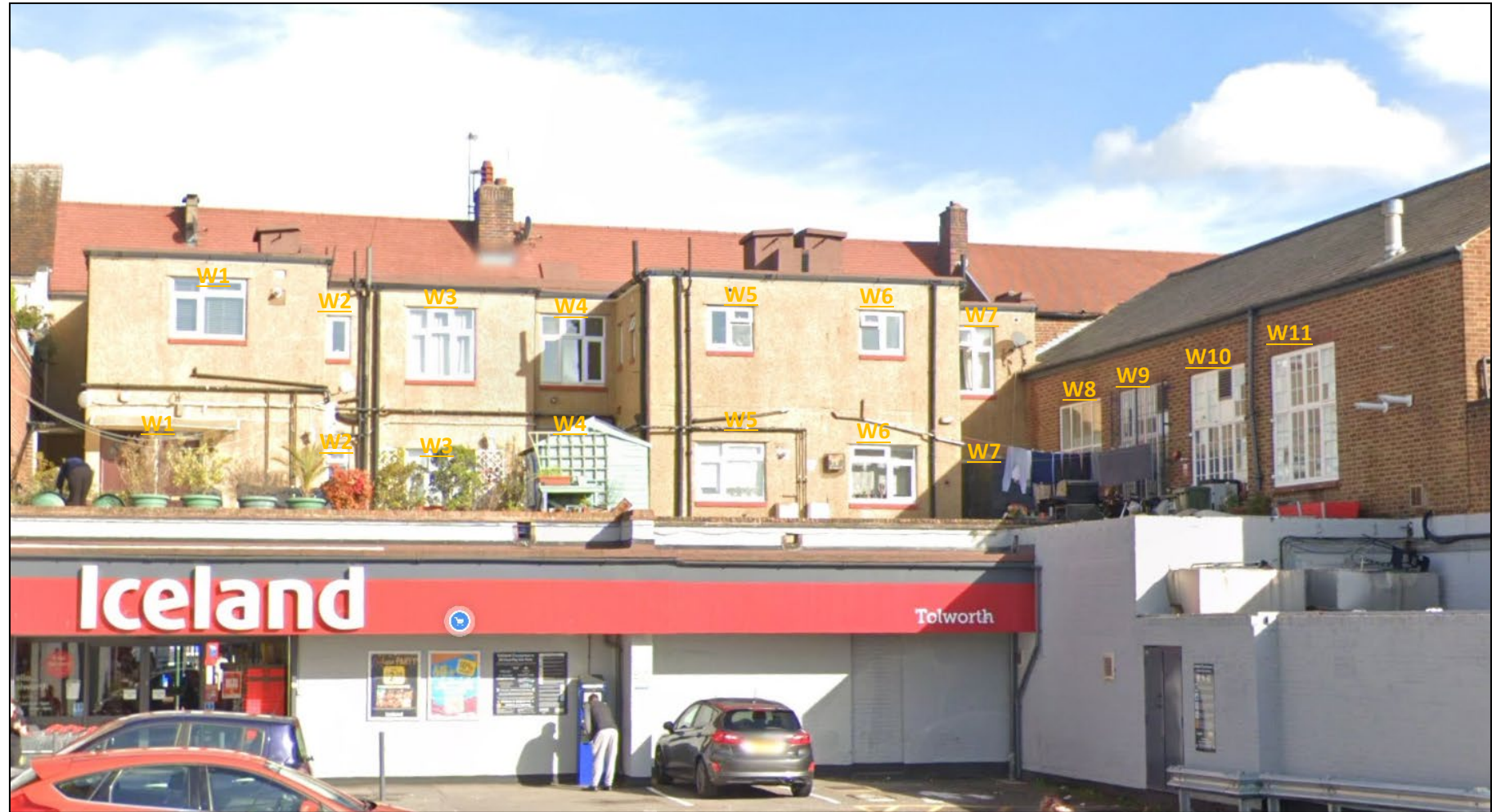
Figure 8: Rear View of 12-18 Tolworth Broadway
