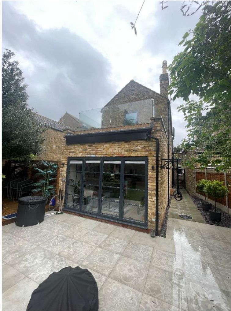
Fig 1. – Flat D, 48 Fassett Road. Adjacent flat's roof terrace.
