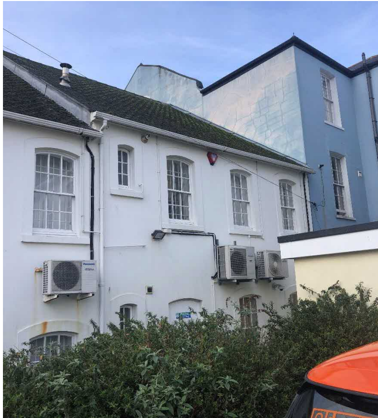
Rear elevation of property
