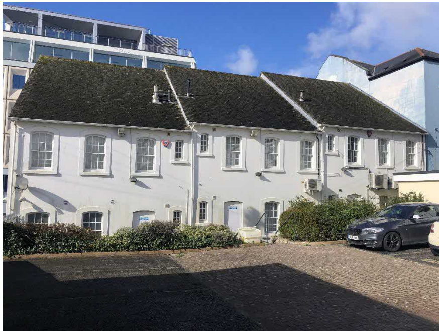
Rear elevation of the property with off-street parking area in the foreground. Unit 3 is to the right hand side.
