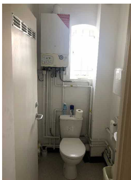
First Floor WC
