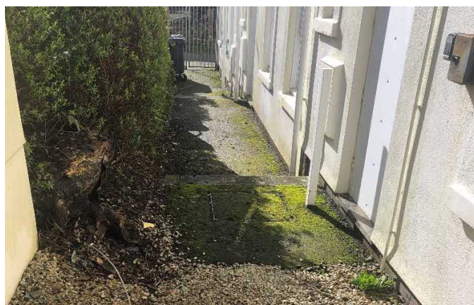
External manhole chamber
