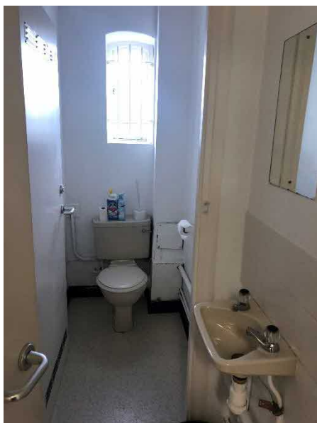
Ground floor WC
