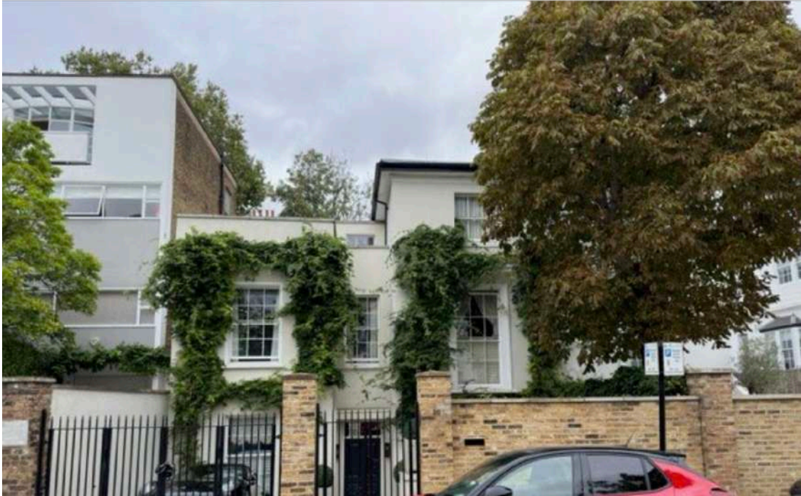
Above: This shows the relationship between nos. 32 and 30 Newton Road and the varied roof form. The eaves and ridge of the main part of the villa at no. 30 are taller than the application property.
