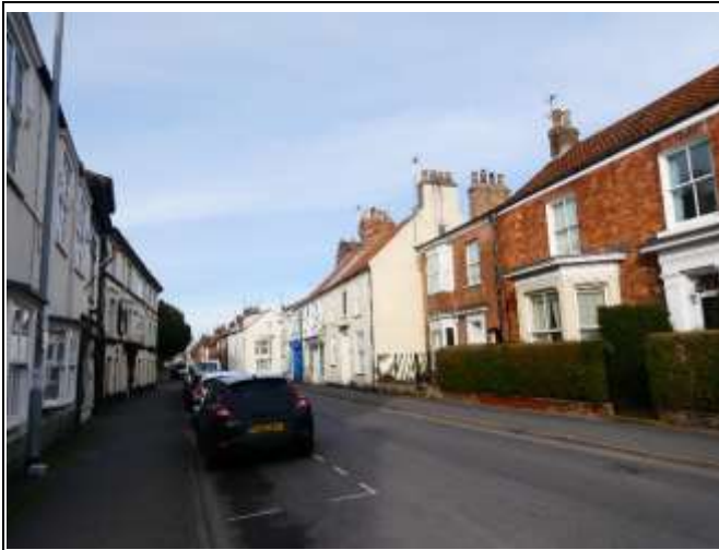
Looking North Towards All Saints Church Along Middle Street North
