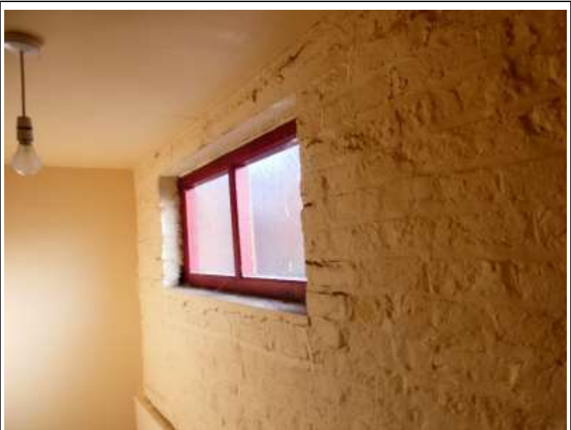
Window at the South Elevation
