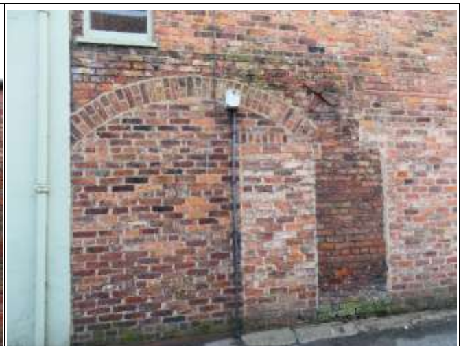
Infilled Sections – Former Archway and Iron Cross Shaped Wall Tie
