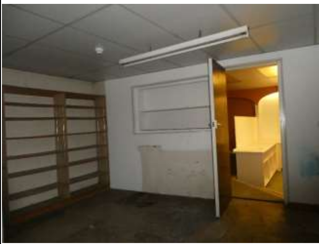
Doorway Leading into Rear Gable Section
