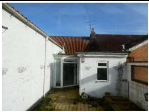
Looking East Towards the Flat Roof Extension and Glazed Link
