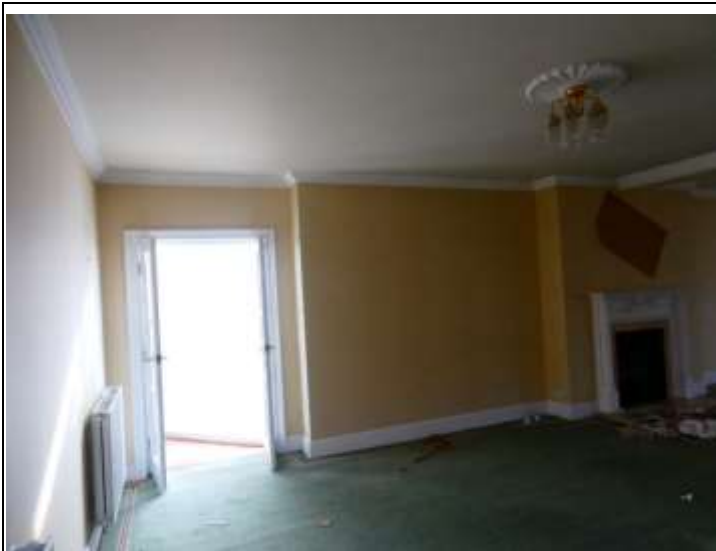
Doors Leading to the Glazed Link
