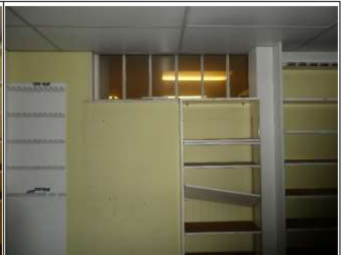
Section of Wall to the Northwest of South Side
