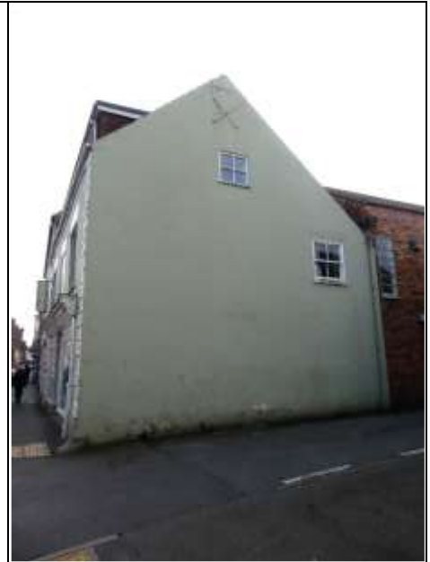
Rendered Section with Cross Shaped Wall Tie
