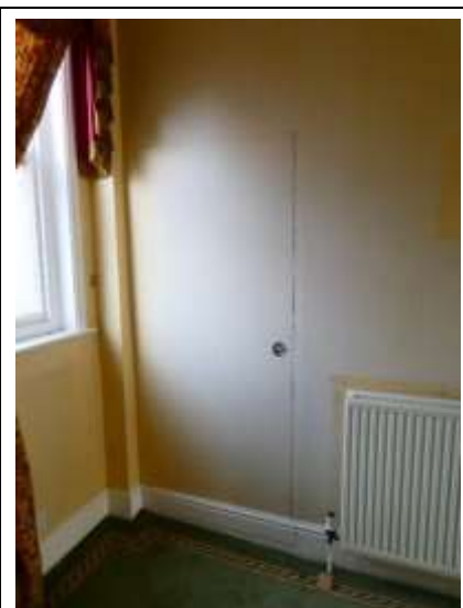
Doorway to the North Staircase
