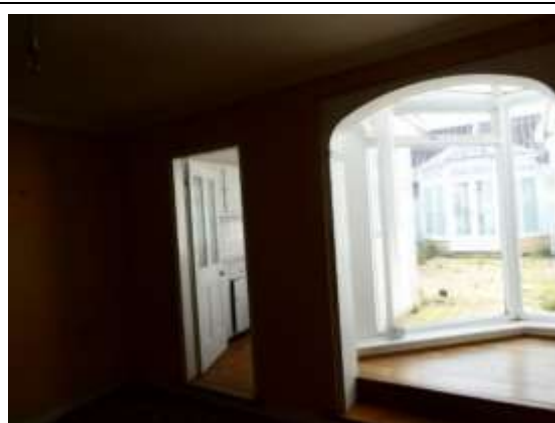
Doorway Leading to Flat Roof Extension
