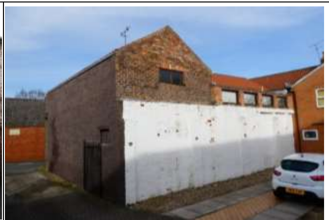
Southern Boundary – Adjacent to Rear Car Park
