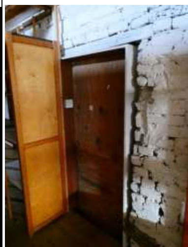
Former Opening Leading to the Living Room
