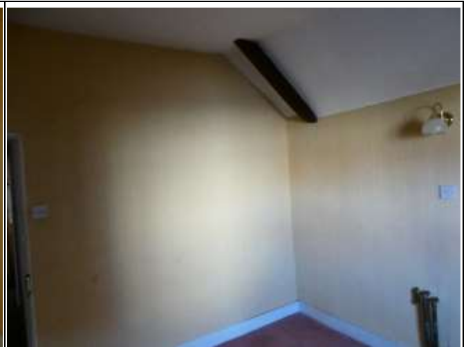
Ceiling Beam – Slanted Ceiling
