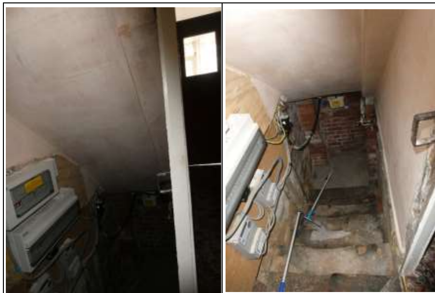
Area Under the Central Stairs
