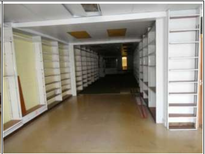
Looking Towards the Rear Along the South Side
