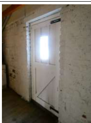
Loading Door at the North Elevation
