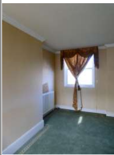
Window at the North Elevation - West End
