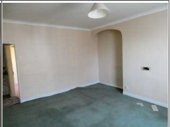
Alcove and Boarded up Fireplace
