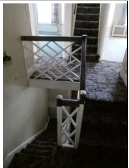
Landing and Stairs Leading to the Second Floor
