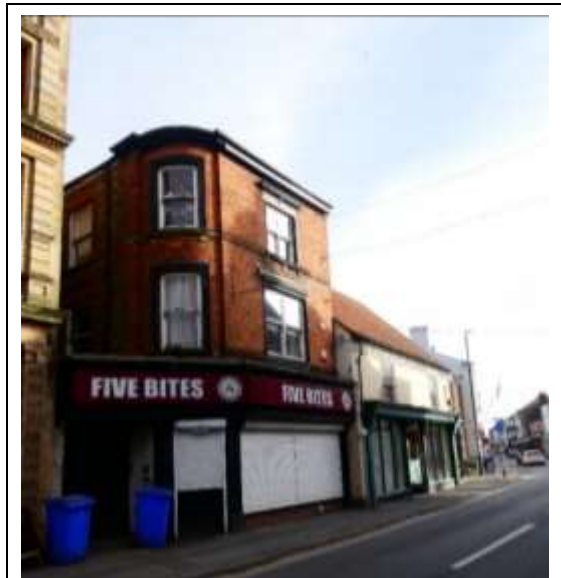
Rounded Wall at 42 & 43 Middle Street North
