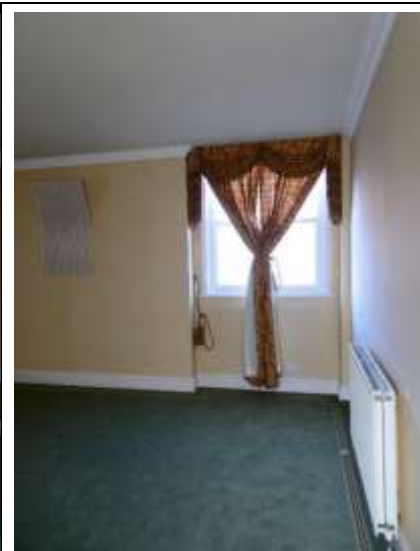
Window at the North Elevation - East End
