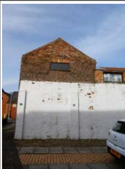
Variation in Brickwork at the Gable End
