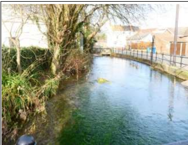
Driffield Beck Alongside Laundry Lane and Under Bridge Street
