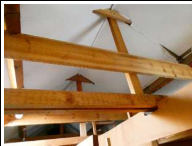
Roof Trusses
