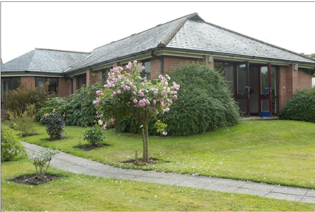
View from north-east of pool building
