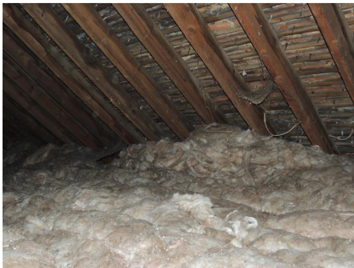
Photo 10: Note lack of evidence of bats on floor of second loft
