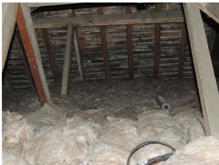
Photo 12: Note lack of evidence of bats on floor of second loft
