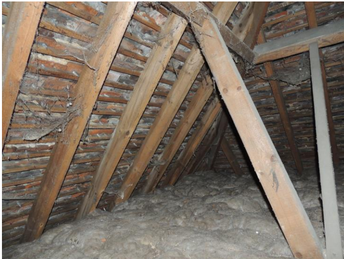
Photo 6: Note lack of evidence of bats on floor of first loft
