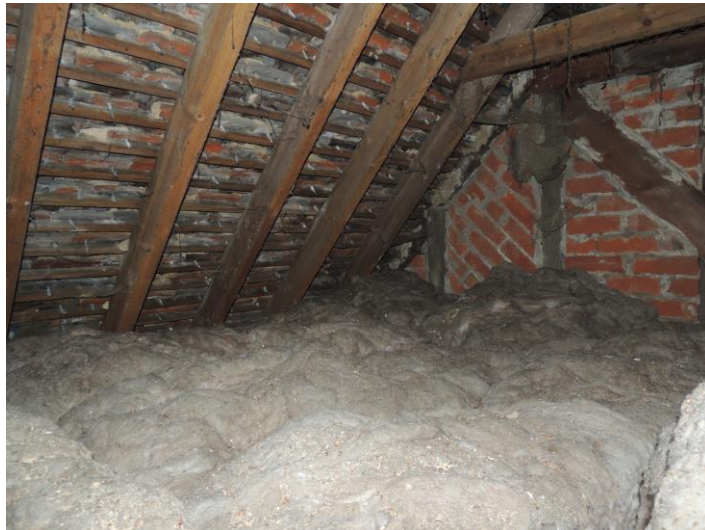
Photo 5: Note lack of evidence of bats on floor of first loft
