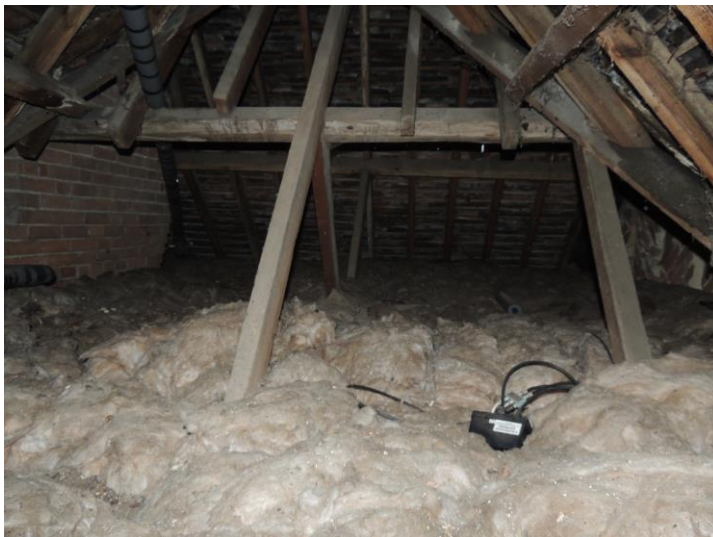
Photo 9: Note lack of evidence of bats on floor of second loft
