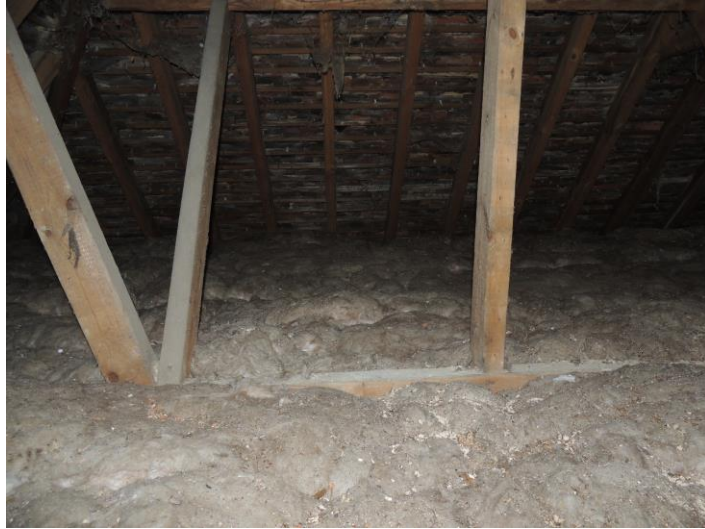
Photo 4: Note lack of evidence of bats on floor of first loft
