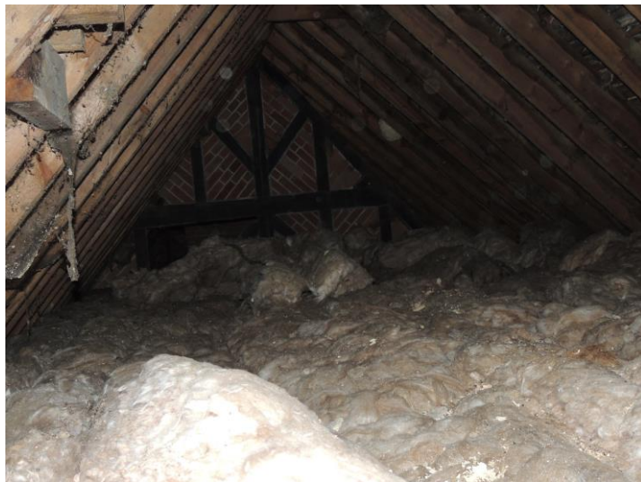
Photo 14: Note lack of evidence of bats on floor of third loft
