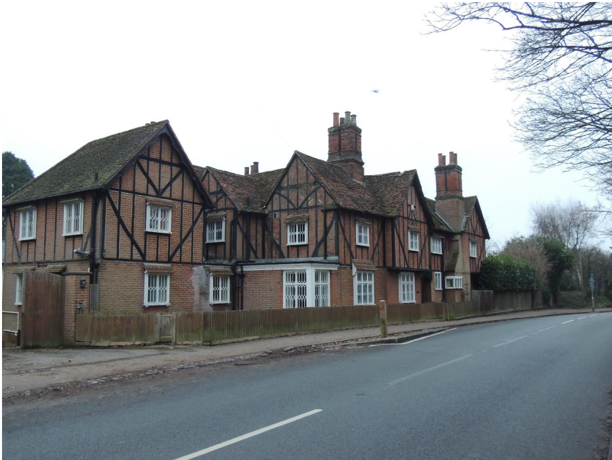
Photo 1: Front (western) elevation. The proposal is for the tiles to be taken off the unlined roof; the roof to be lined and the tiles replaced back on the roof. It is anticipated that the work will be done in sections
