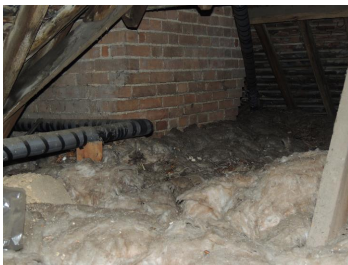
Photo 11: Note lack of evidence of bats on floor of second loft
