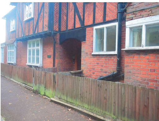
35. Existing timber fence to street boundary
