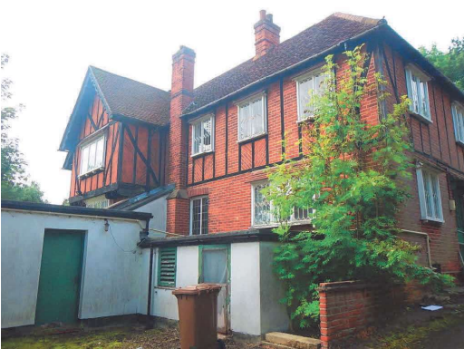
8. East elevation from north-east
