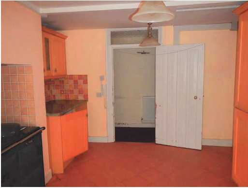
32. West facing kitchen wall (to be removed)
