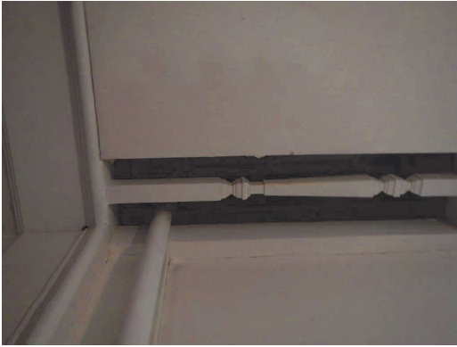
24. Plasterboard concealing stair spindles/banister
