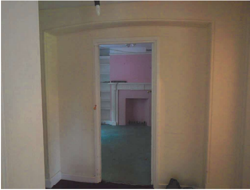
21. Timber stud and plasterboard infill to opening
