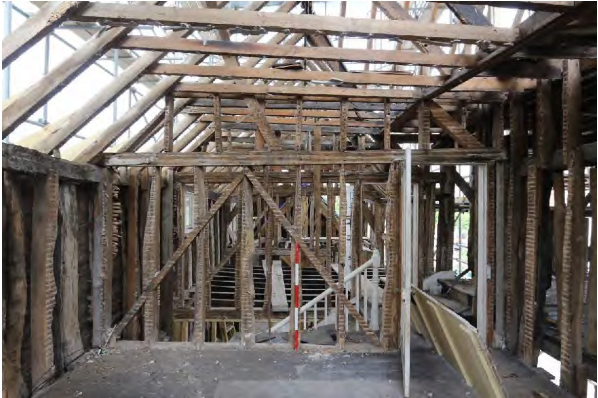
Plate 67 Northern primary braced wall of (F1)
