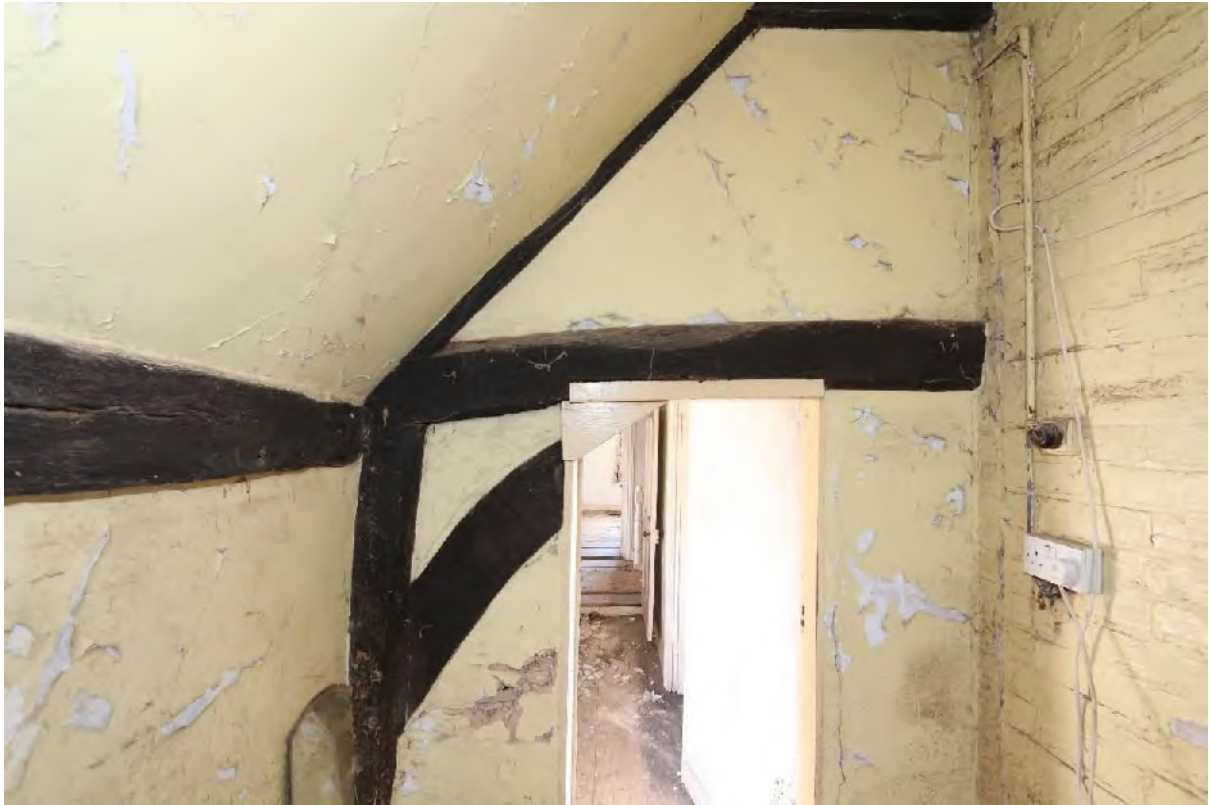
Plate 37 Bathroom (F7), showing curving arch brace, looking south
