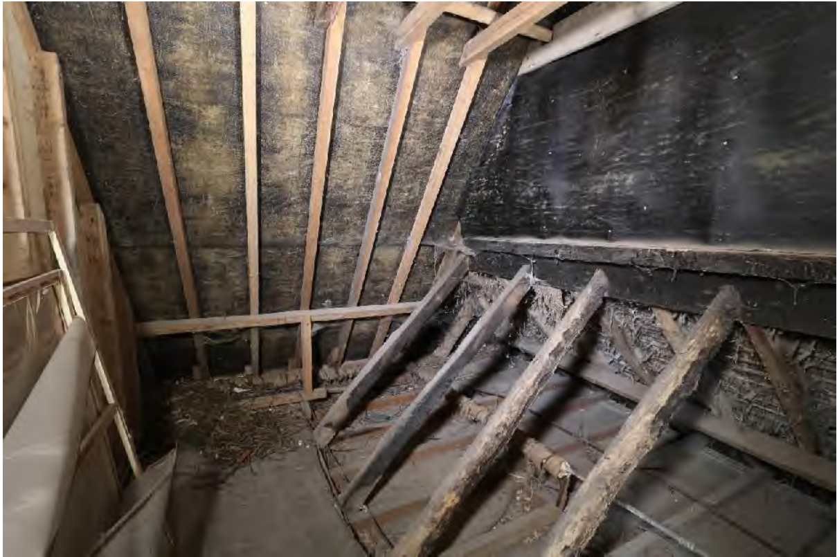
Plate 41 Rebuilt roof of 1947 and reworked roof over cross-wing (right)
