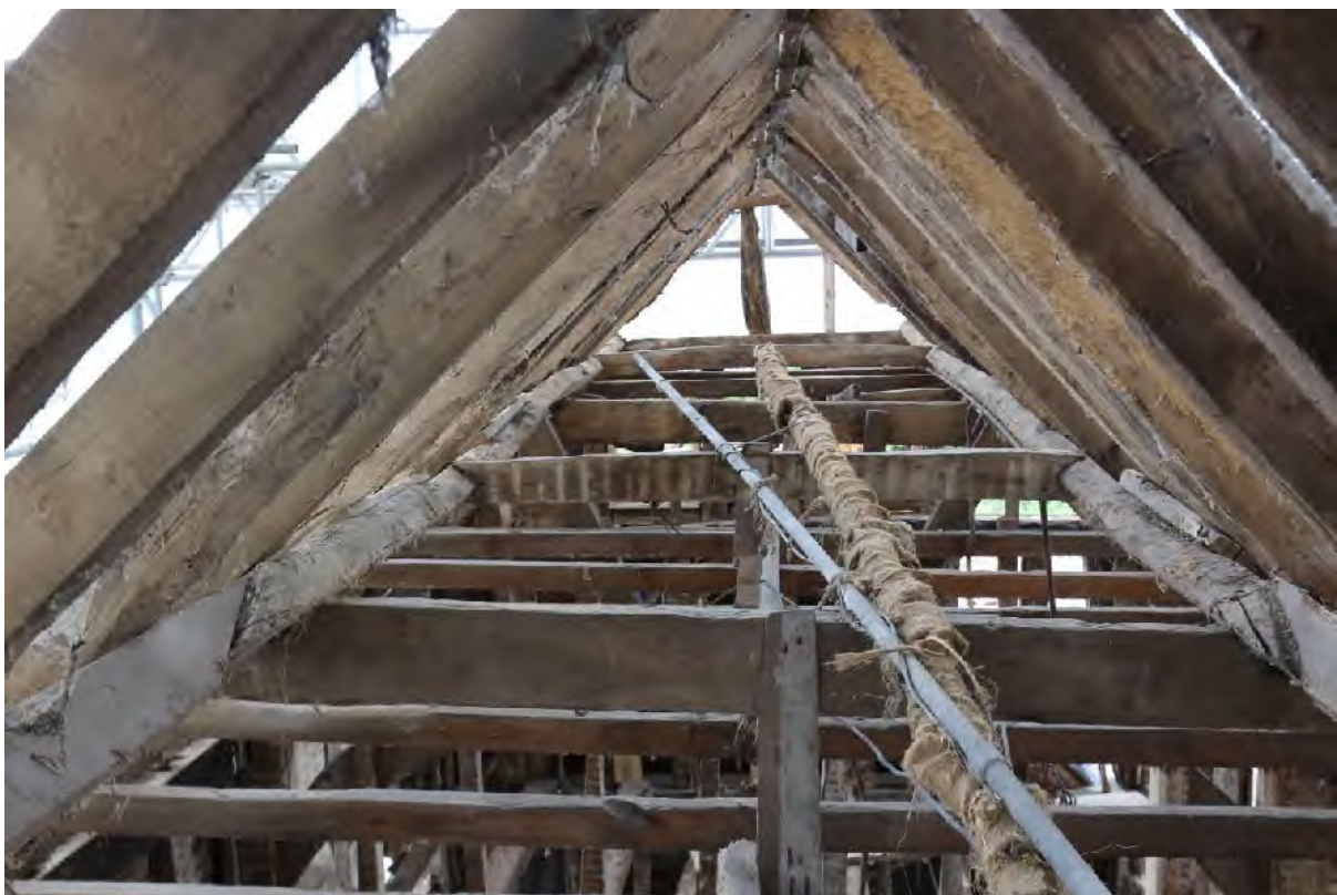
Plate 96 Roof showing clasped purlins and intermediate collars
