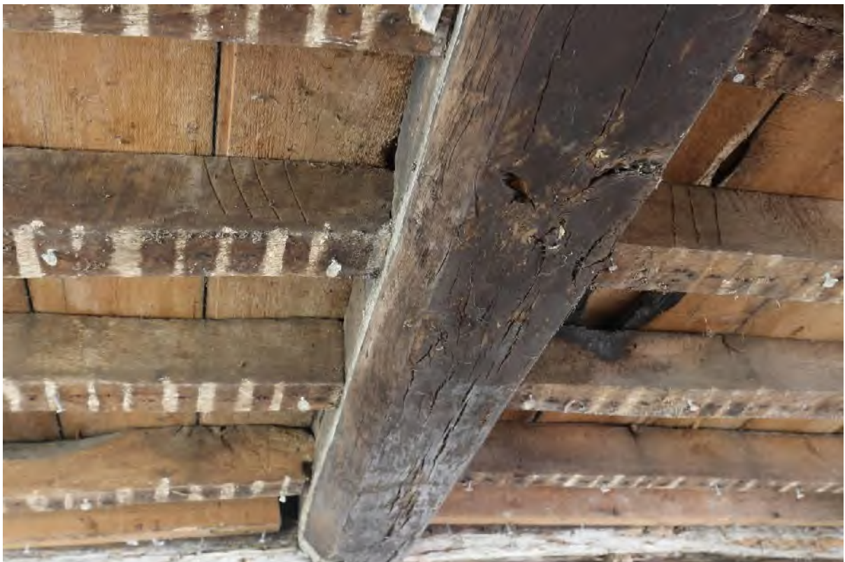
Plate 80 Scribed Roman carpentered marks on ceiling joists
