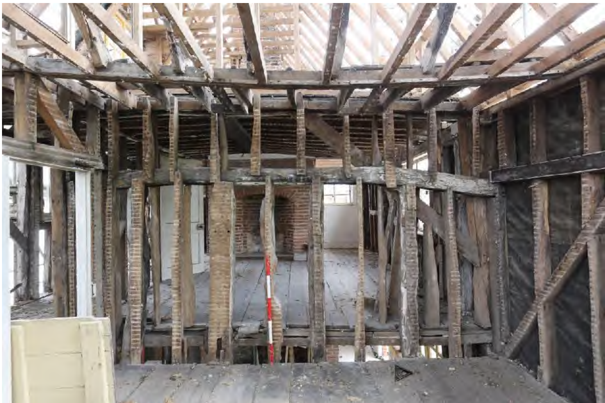
Plate 72 Eastern wall of (F1) showing original storey post and top plate, looking east
