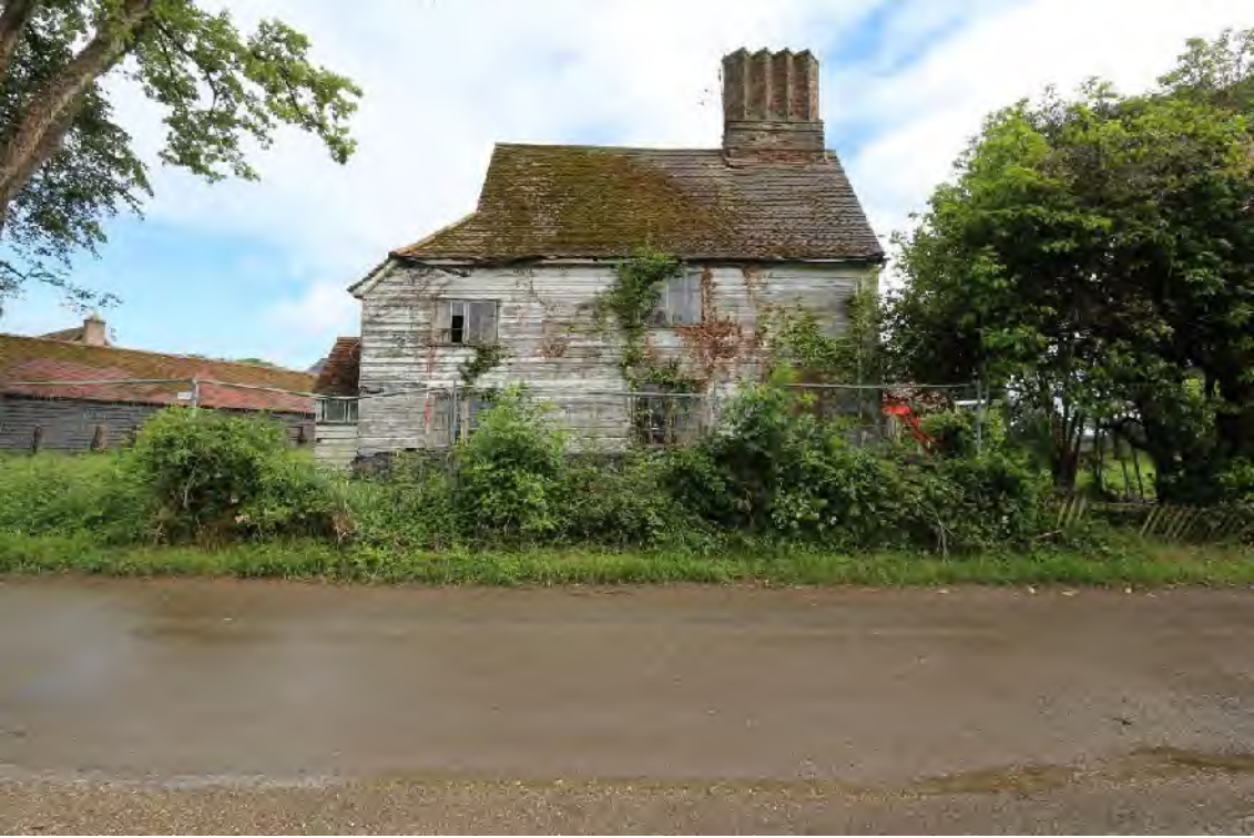
Plate 1 Principal southern elevation, looking north
