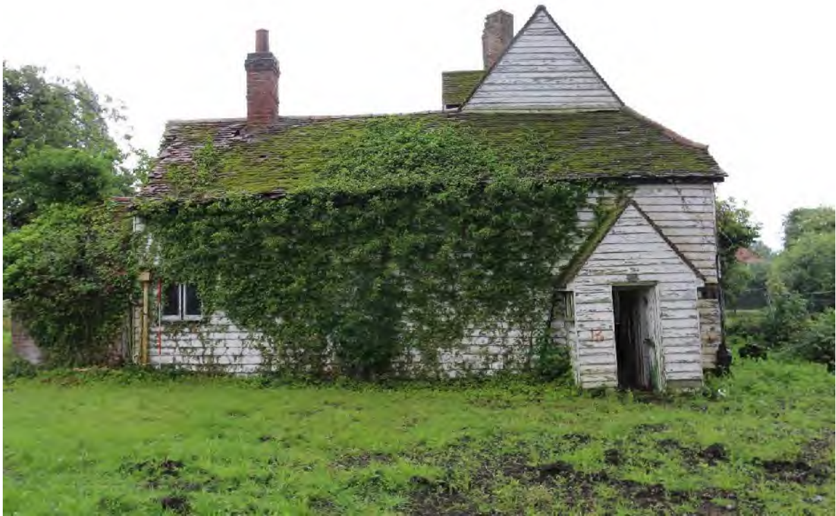
Plate 5 Western elevation, looking east
