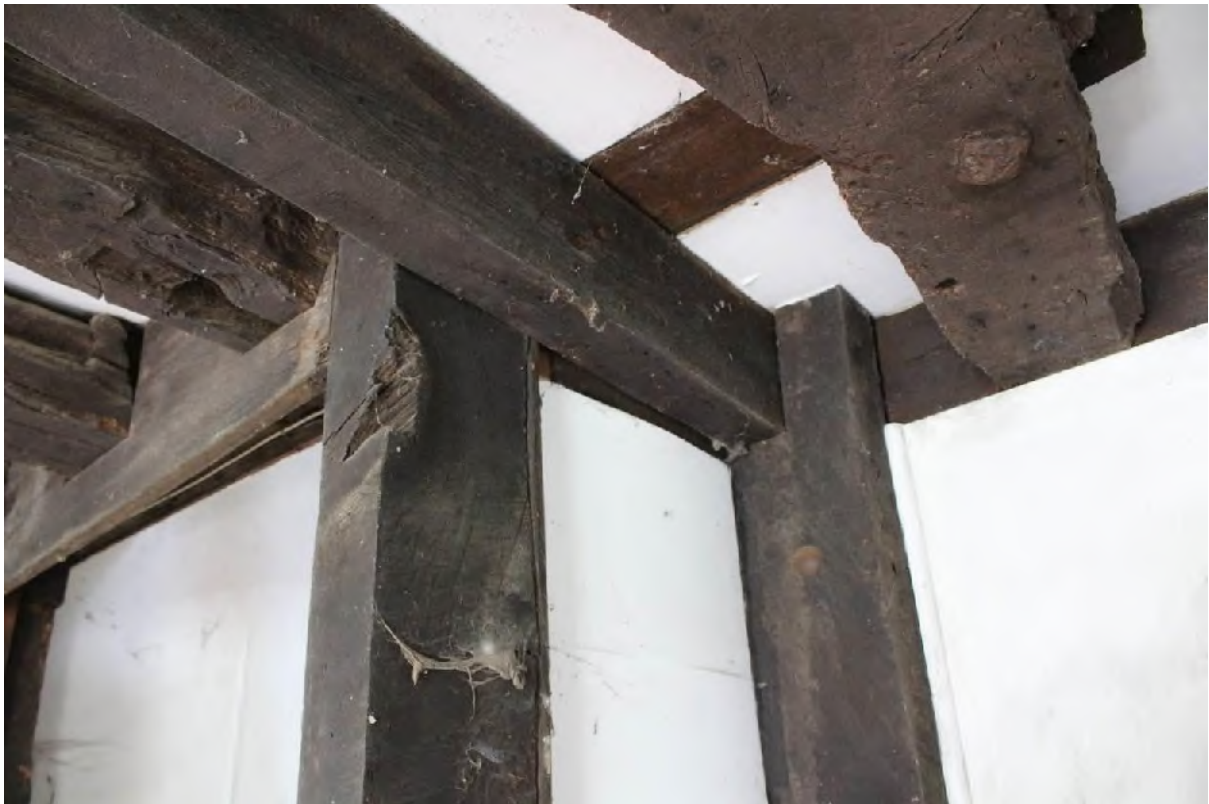
Plate 16 Detail of later structure supporting inserted stair
