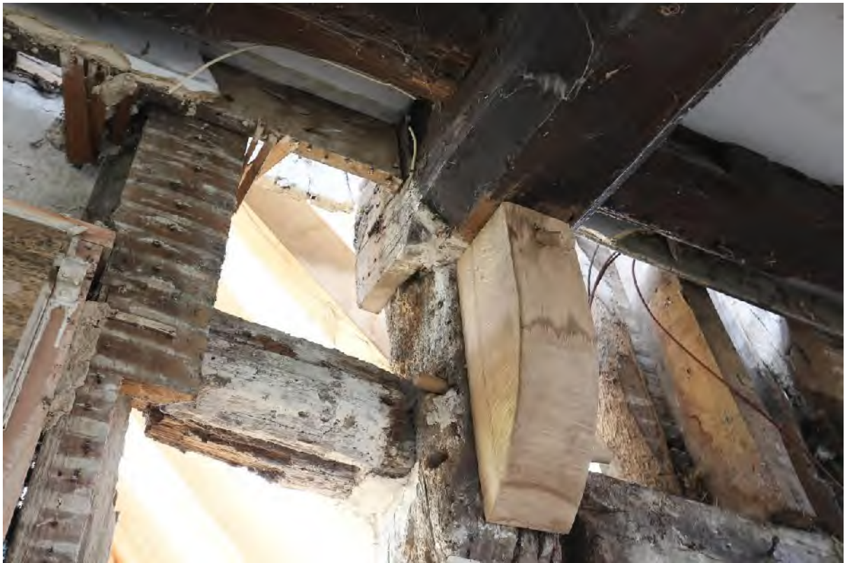
Plate 54 Stopped end to bridging beam (G1) and jowl to post
