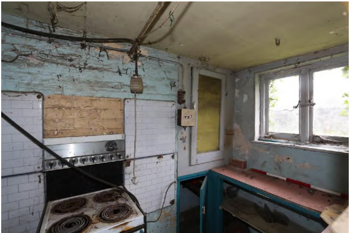
Plate 26 Kitchen (G4) showing back of chimneystack and meat safe, looking south-west
