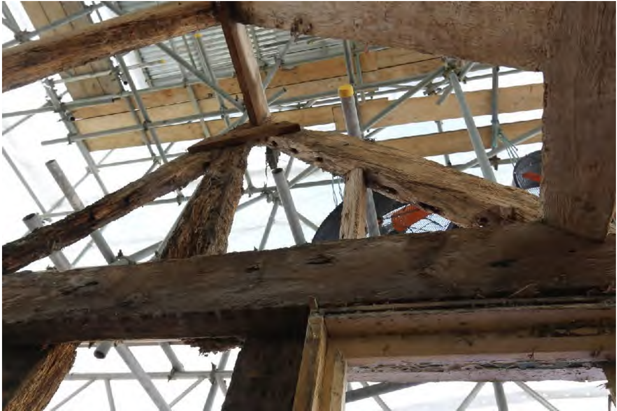
Plate 93 Stave holes in soffit of principal rafters, northern end of cross wing
