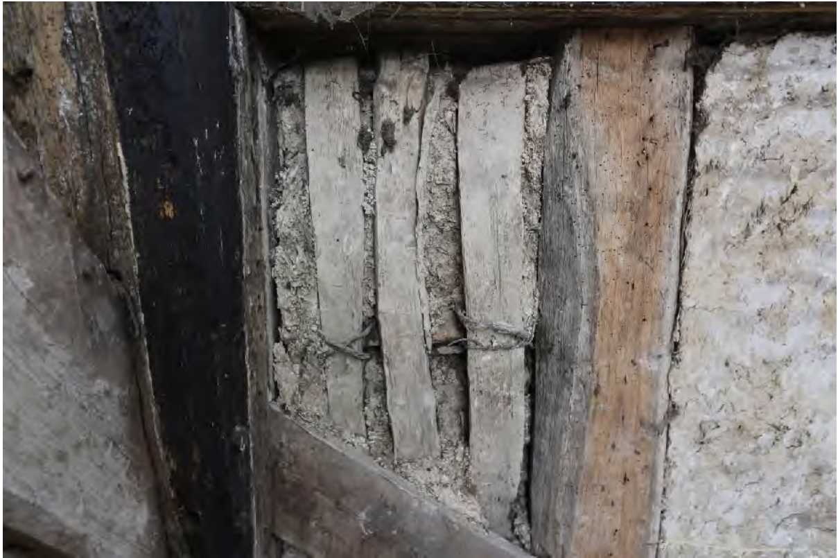
Plate 91 Detail of wattle and daub wall infill
