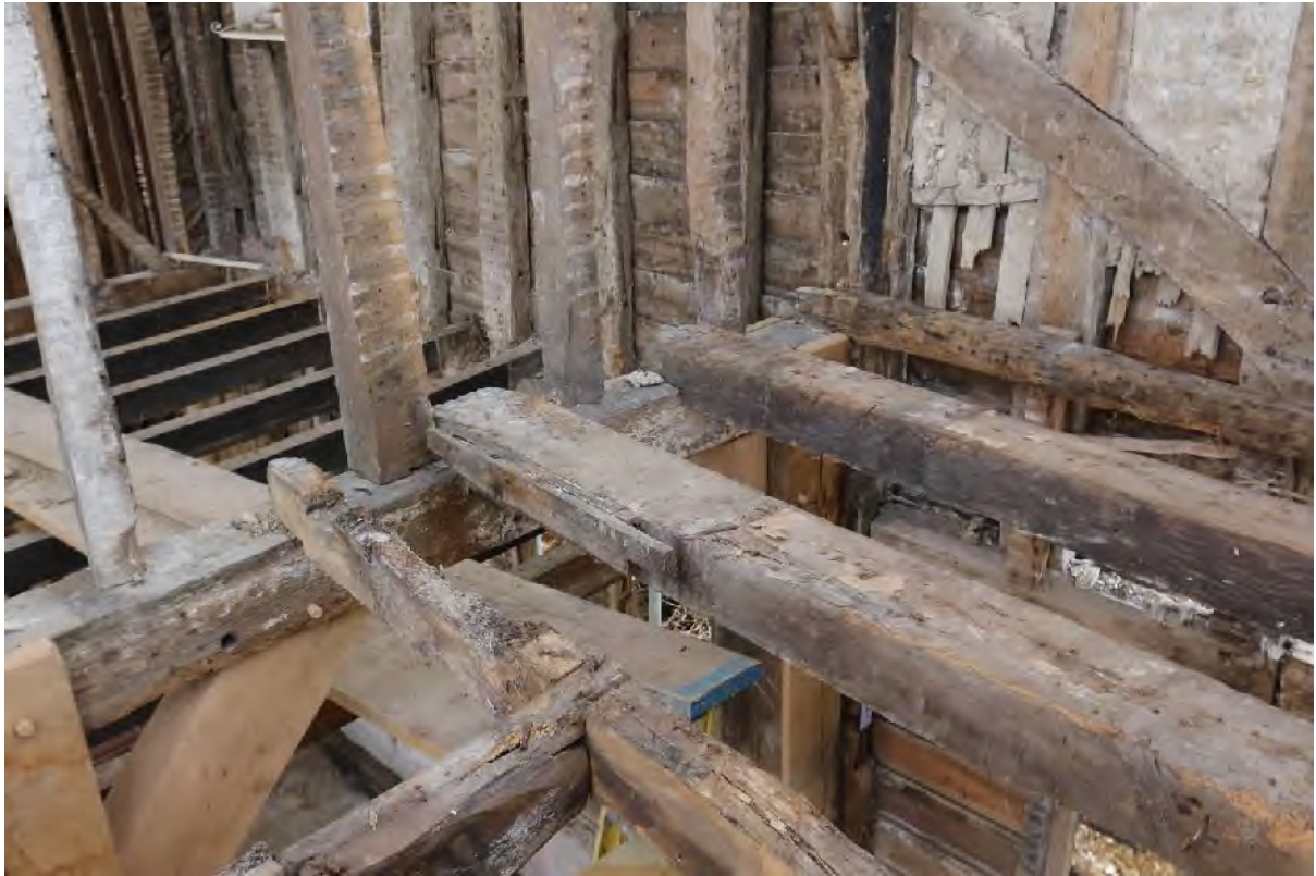
Plate 65 Stout first floor joists in (G4)
