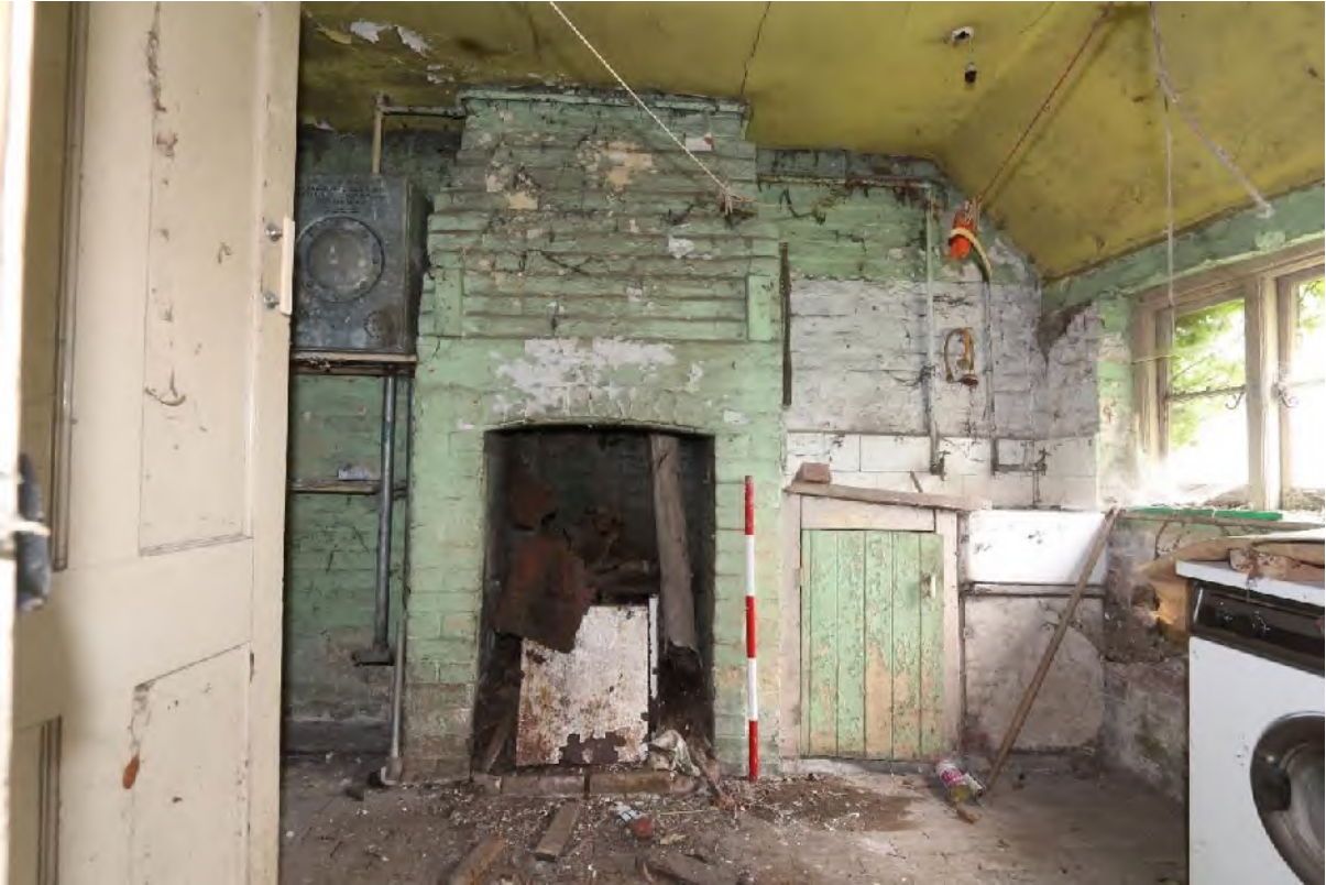
Plate 27 Utility room (G5) looking north
