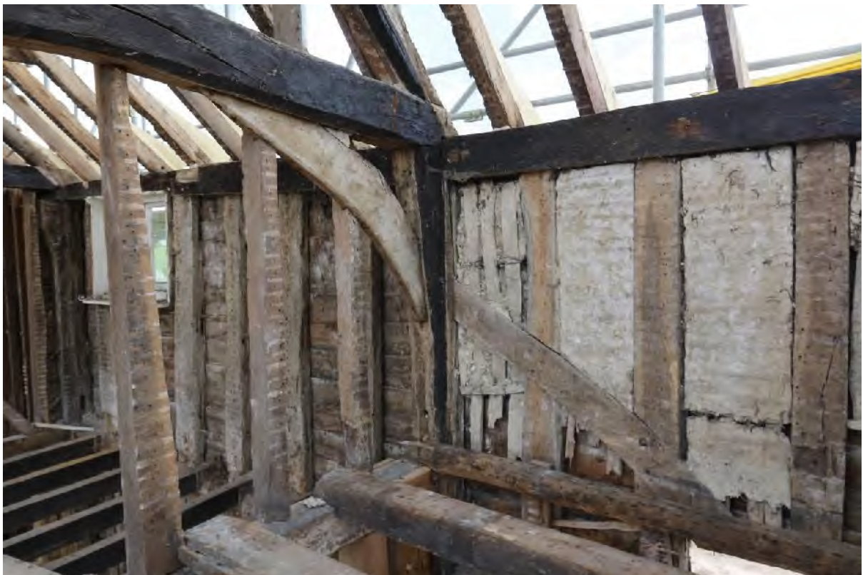
Plate 90 Original wattle and daub wall infill, west wall of (F7)
