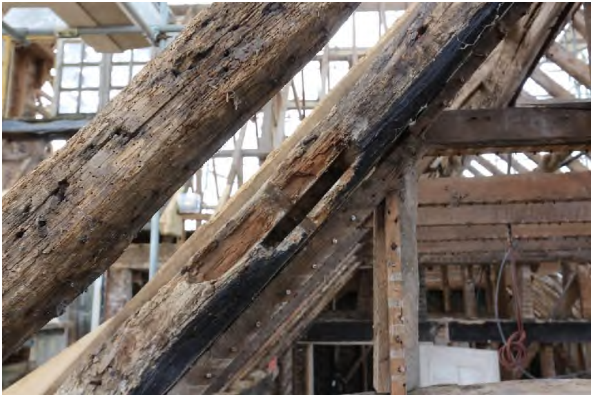
Plate 94 Narrow mortise for a wind brace cut into principal rafter
