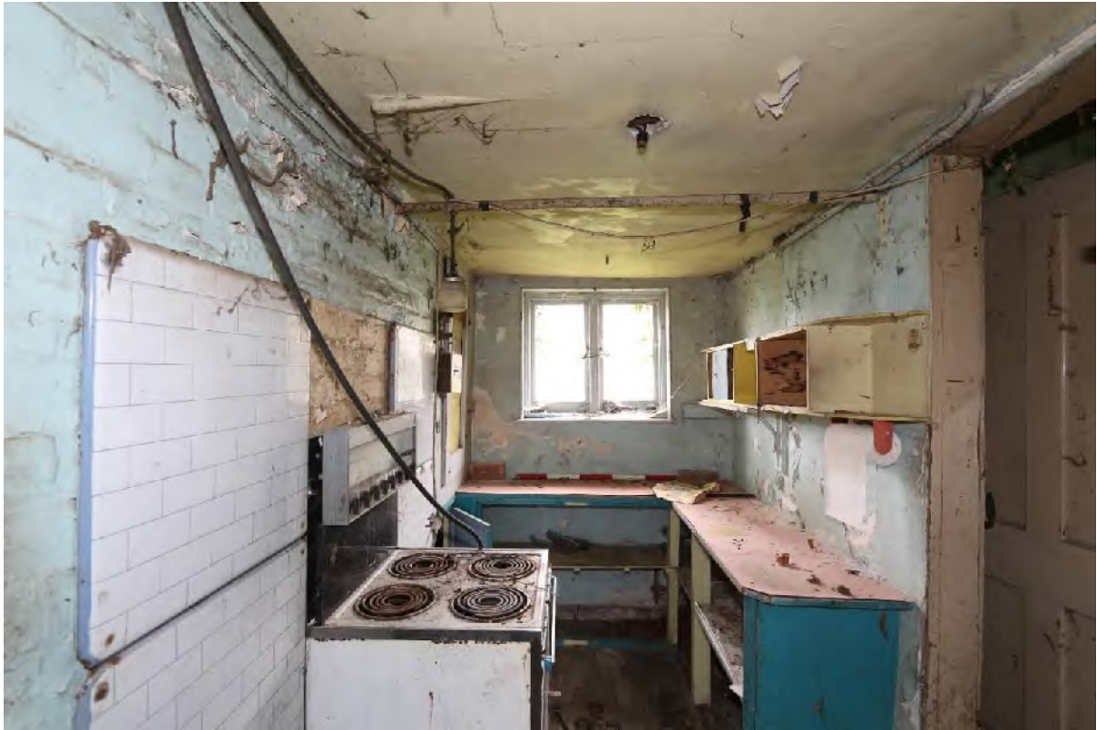
Plate 25 Kitchen (G4) looking west
