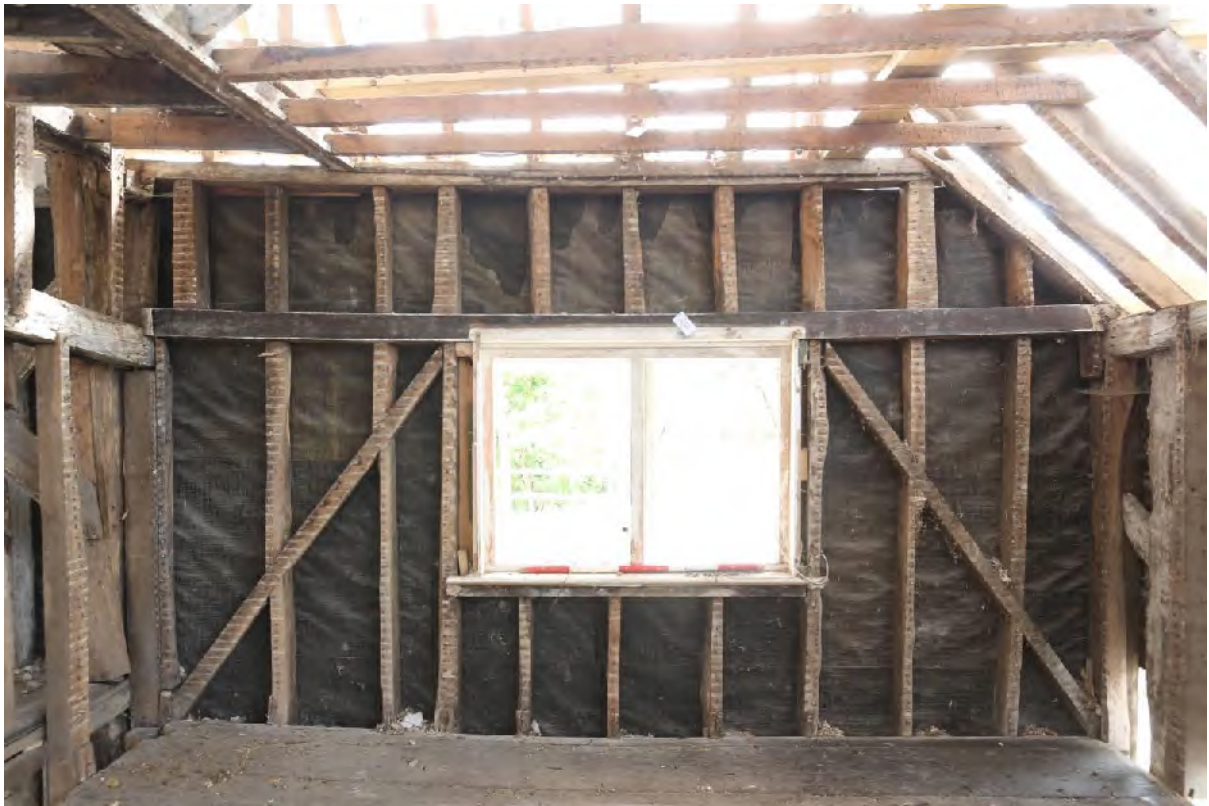
Plate 68 Southern primary braced wall of (F1)
