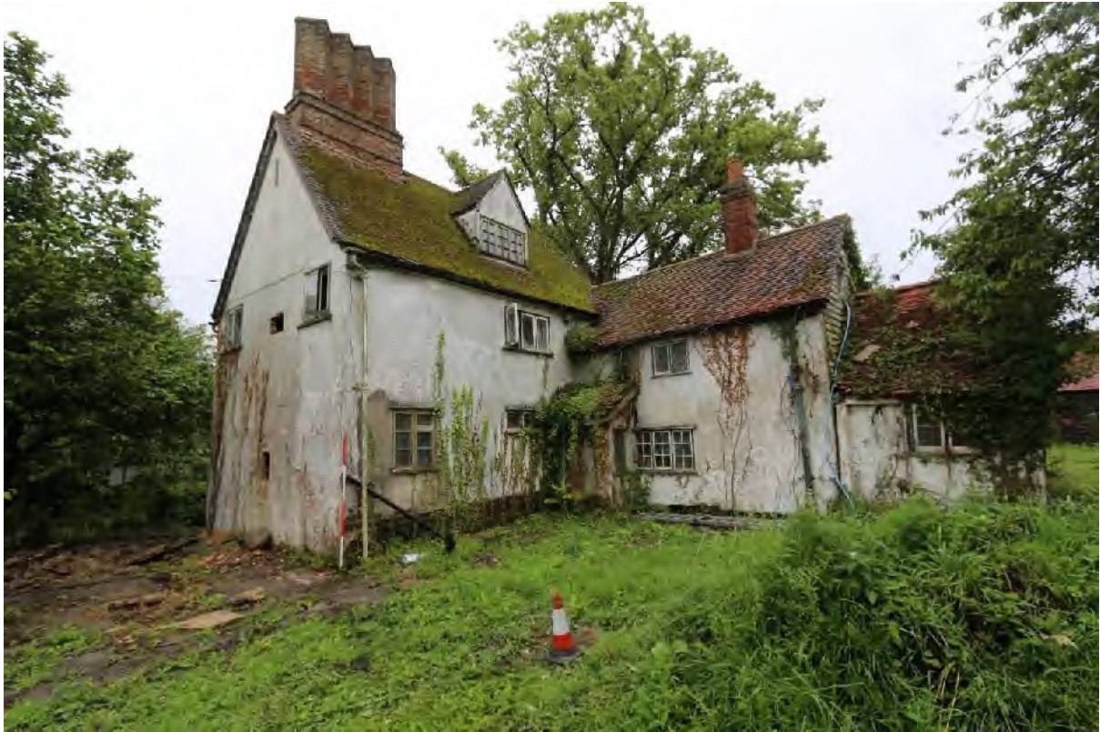
Plate 3 Eastern and northern elevations, looking south-west
