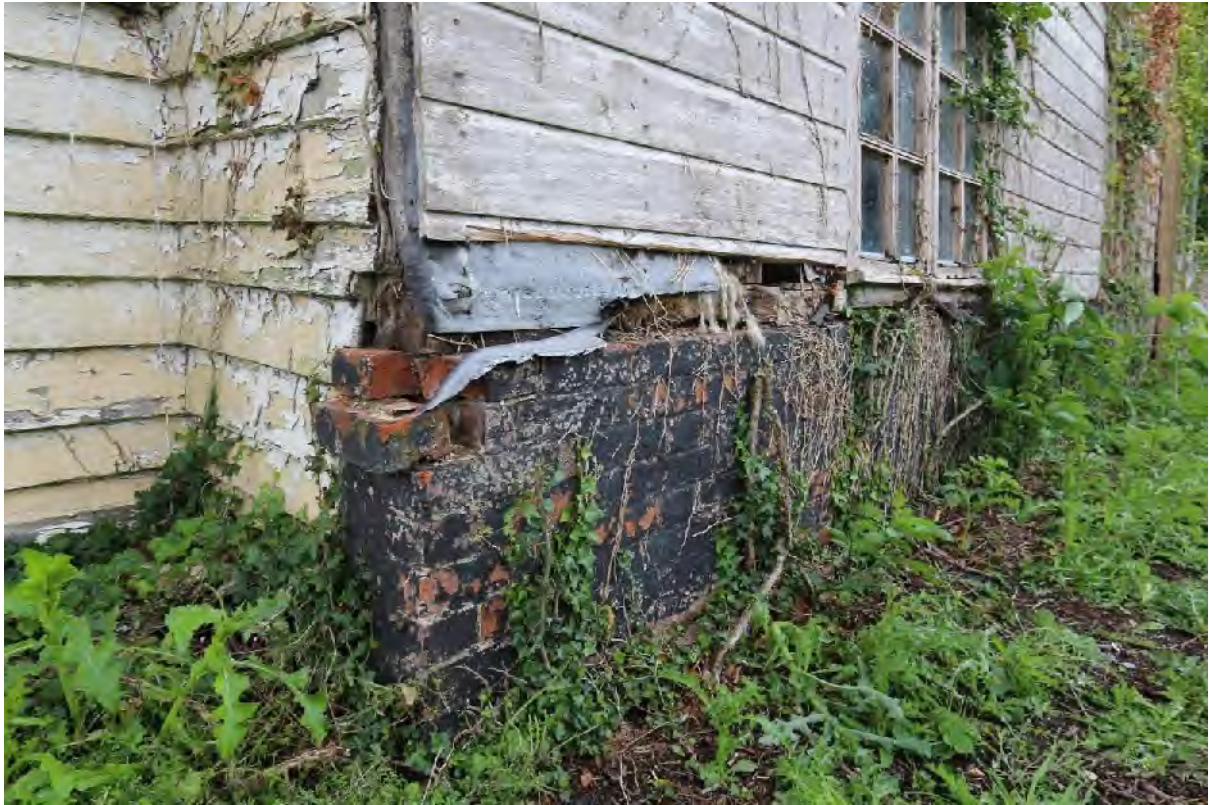
Plate 9 Rebuilt dwarf wall and ship lap boards to south elevation
