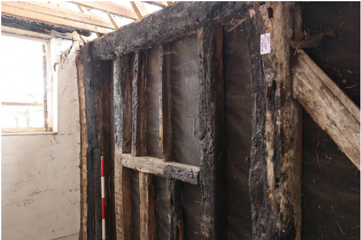
Plate 78 Southern wall to (F2), showing former window and burning
