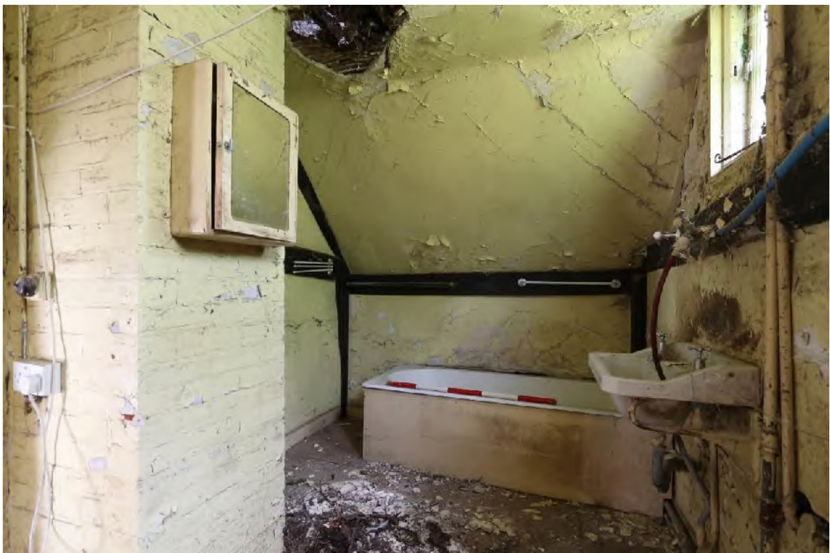
Plate 36 Bathroom (F7) looking west
