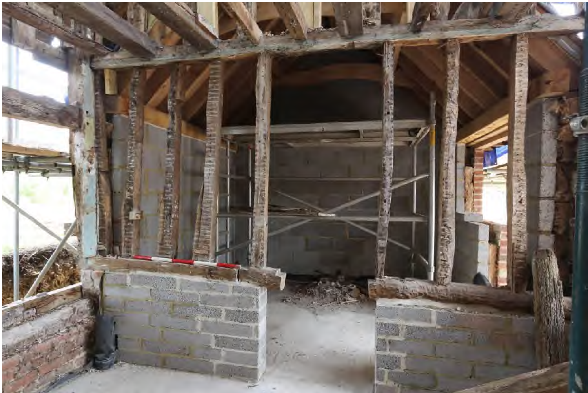
Plate 64 Northern end wall of (G4)
