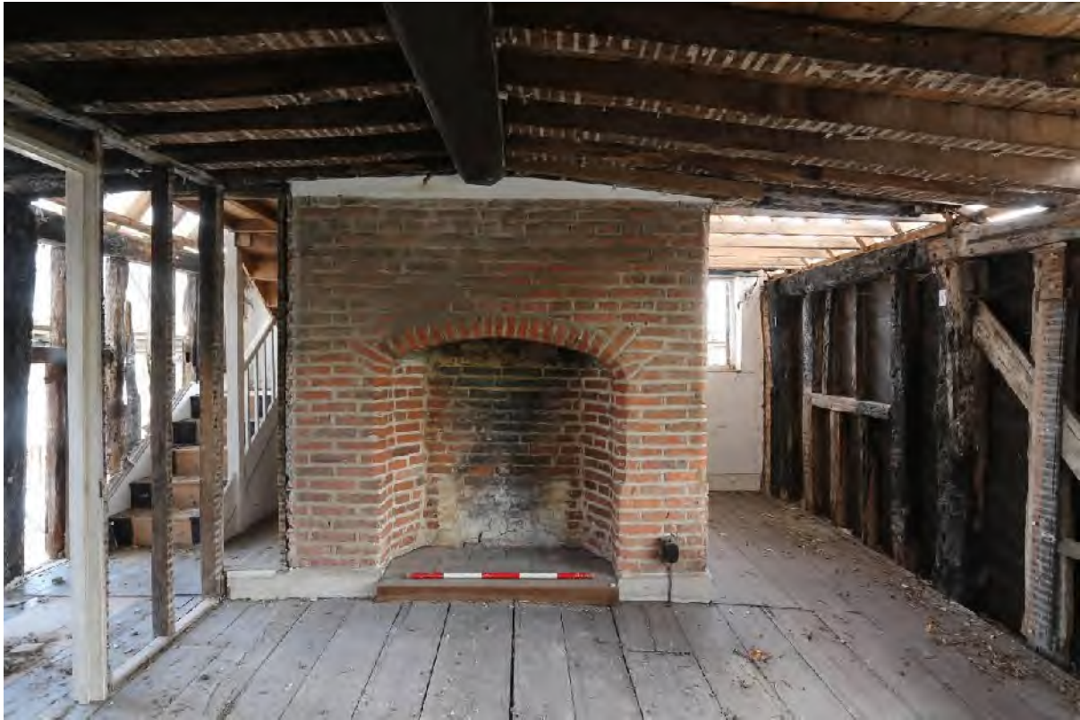
Plate 75 Brick fireplace in (F2) looking east
