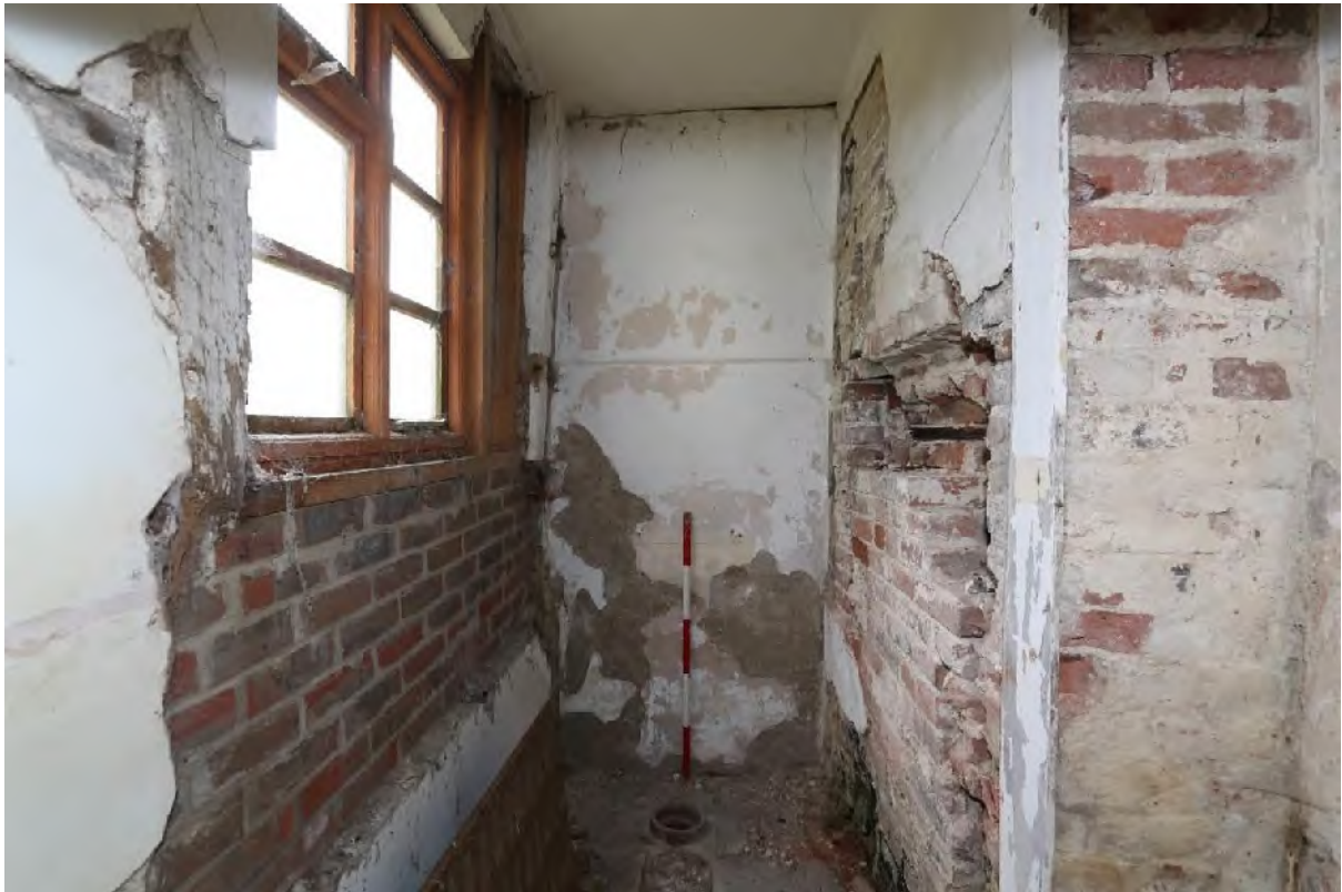
Plate 20 Former toilet (G2B), showing cut away posts (left), looking east
