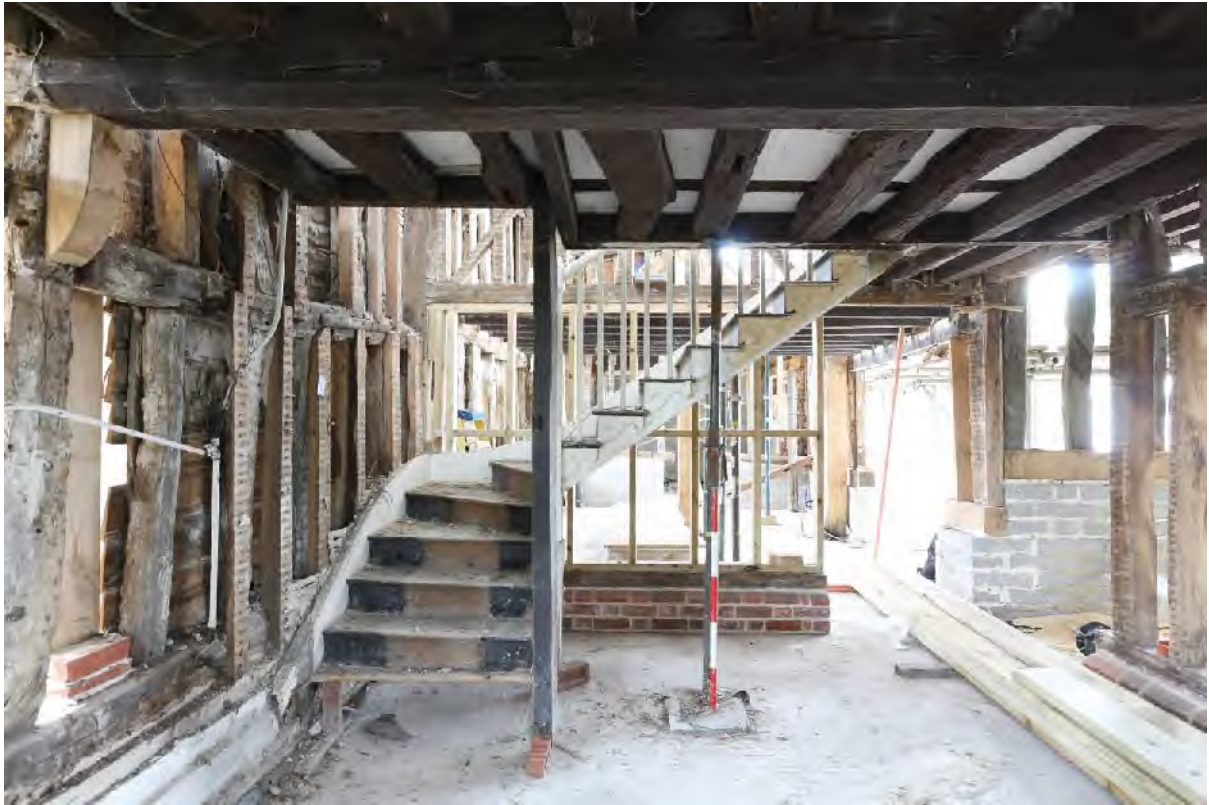
Plate 55 Inserted stair and rebuilt northern wall to (G1)
