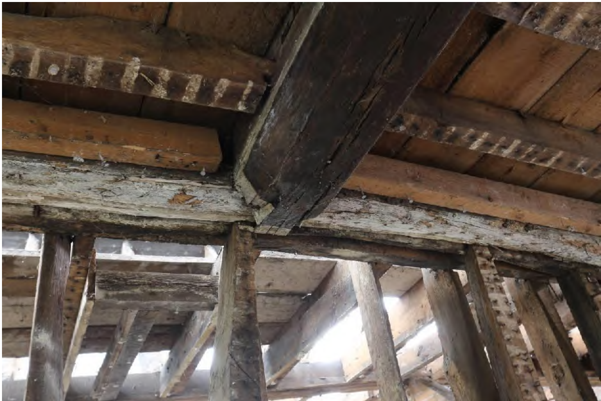
Plate 74 Inserted, higher, tie-beam carrying bridging beam in (F2)
