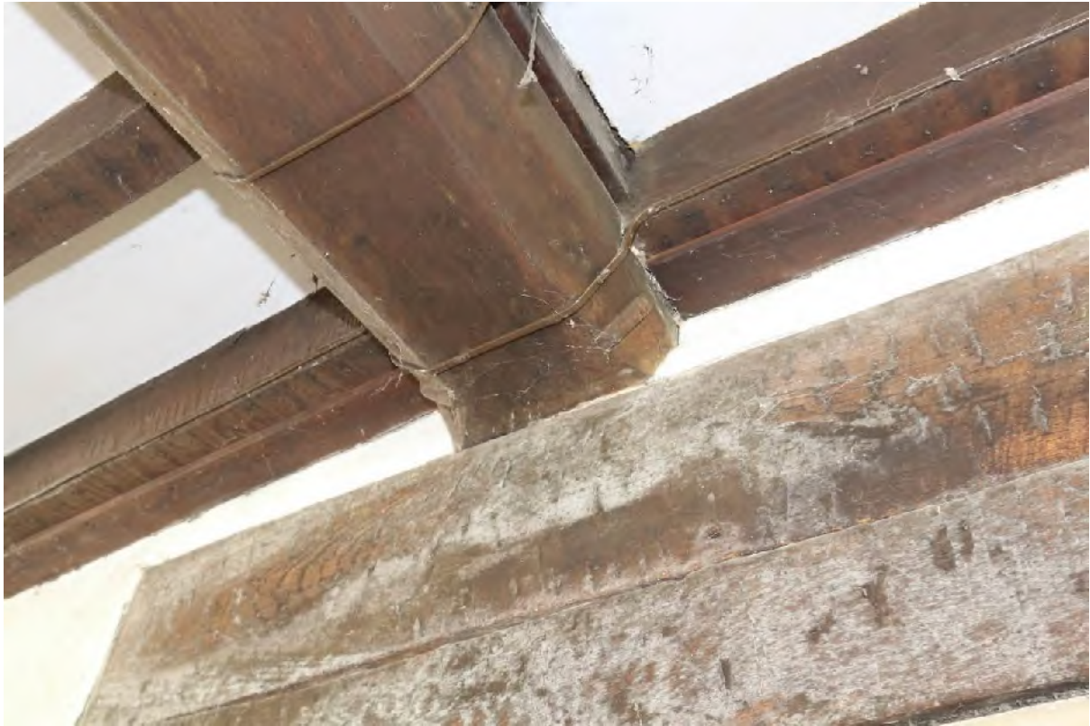
Plate 19 Detail of chamfer stop (G2)
