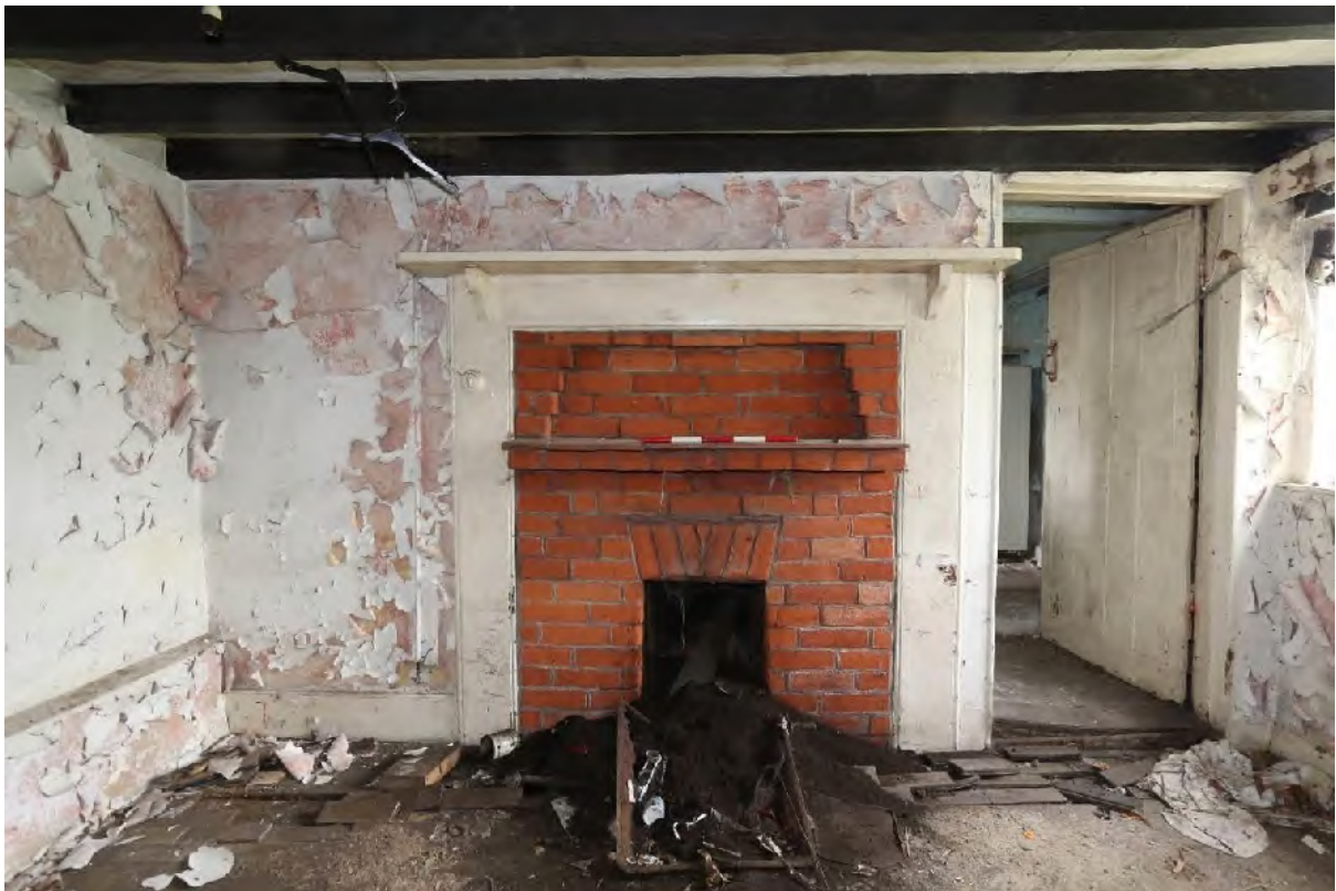
Plate 22 Room (G3) looking north
