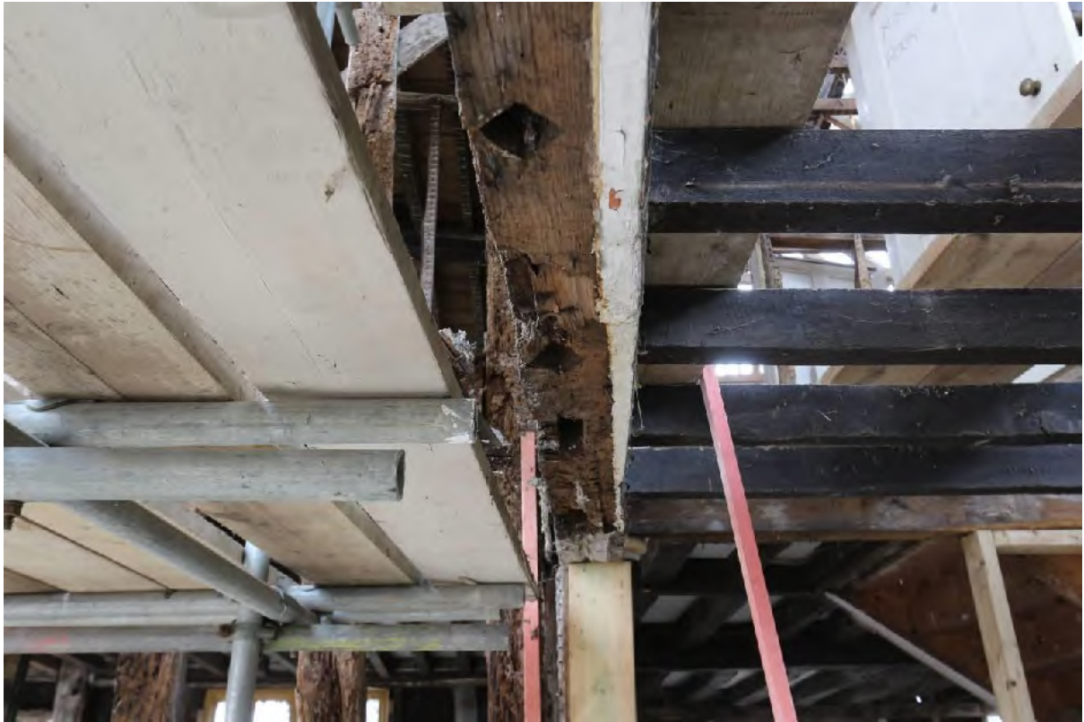
Plate 61 Evidence of diamond mullion window, east wall of (G3)
