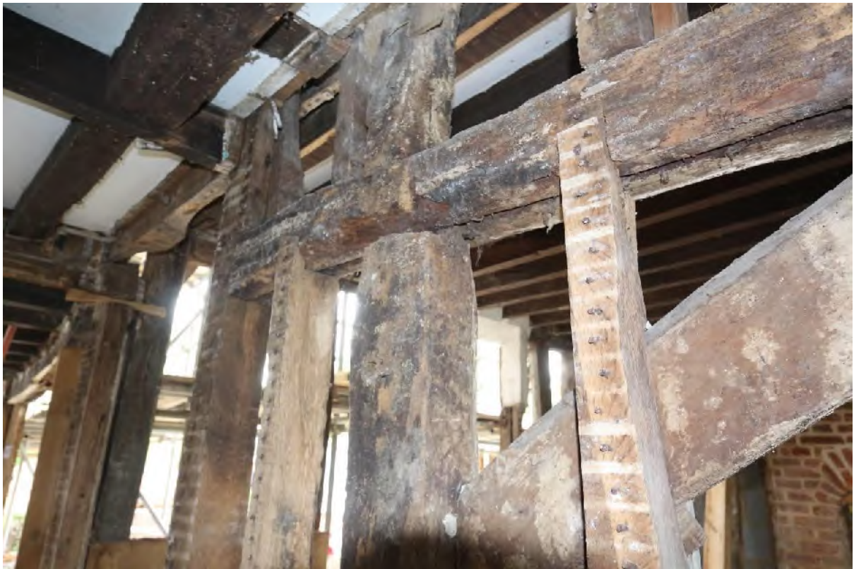
Plate 52 Wattle trench in soffit of mid rail (east wall to G1)
