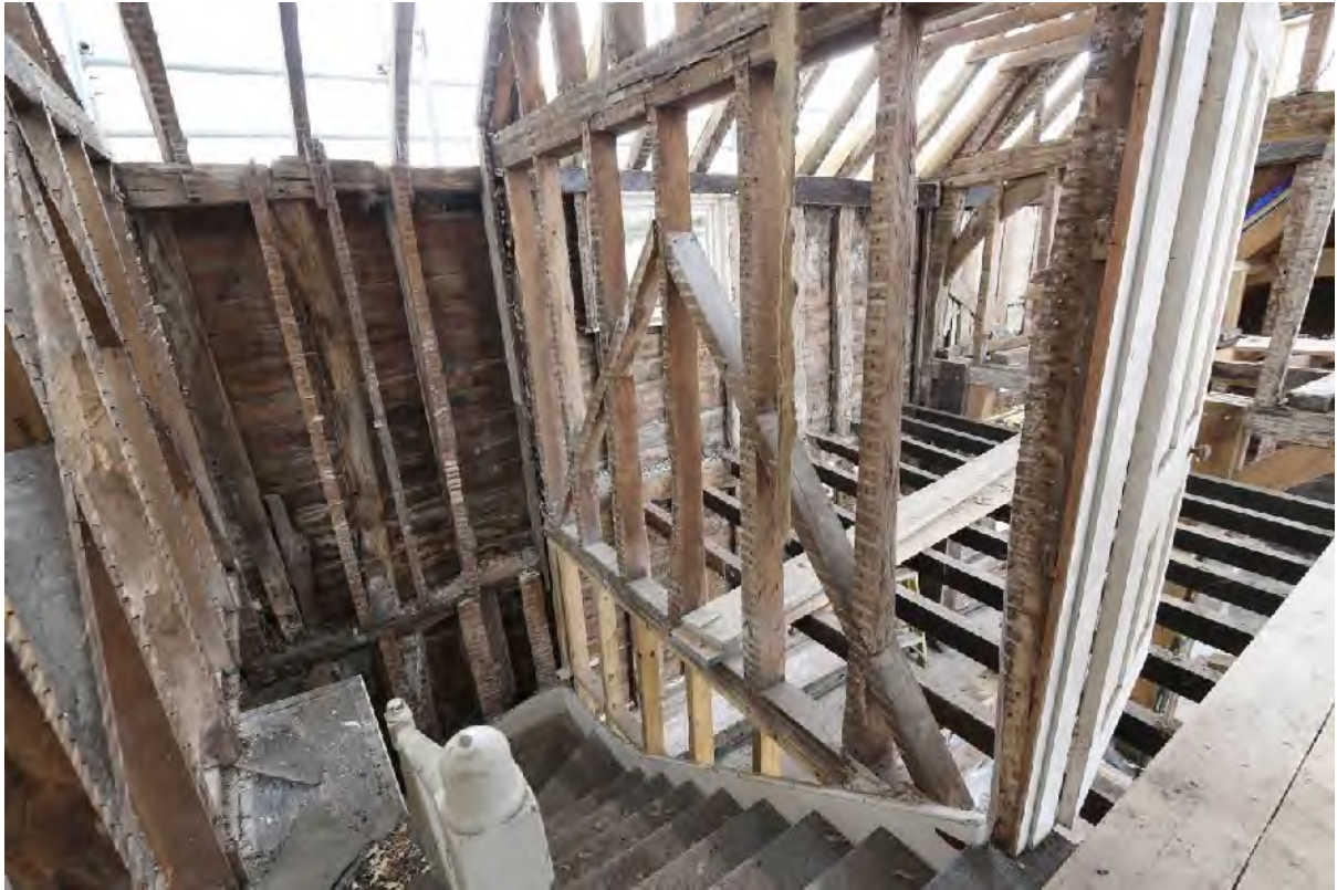
Plate 69 Primary braced wall frame to stairwell
