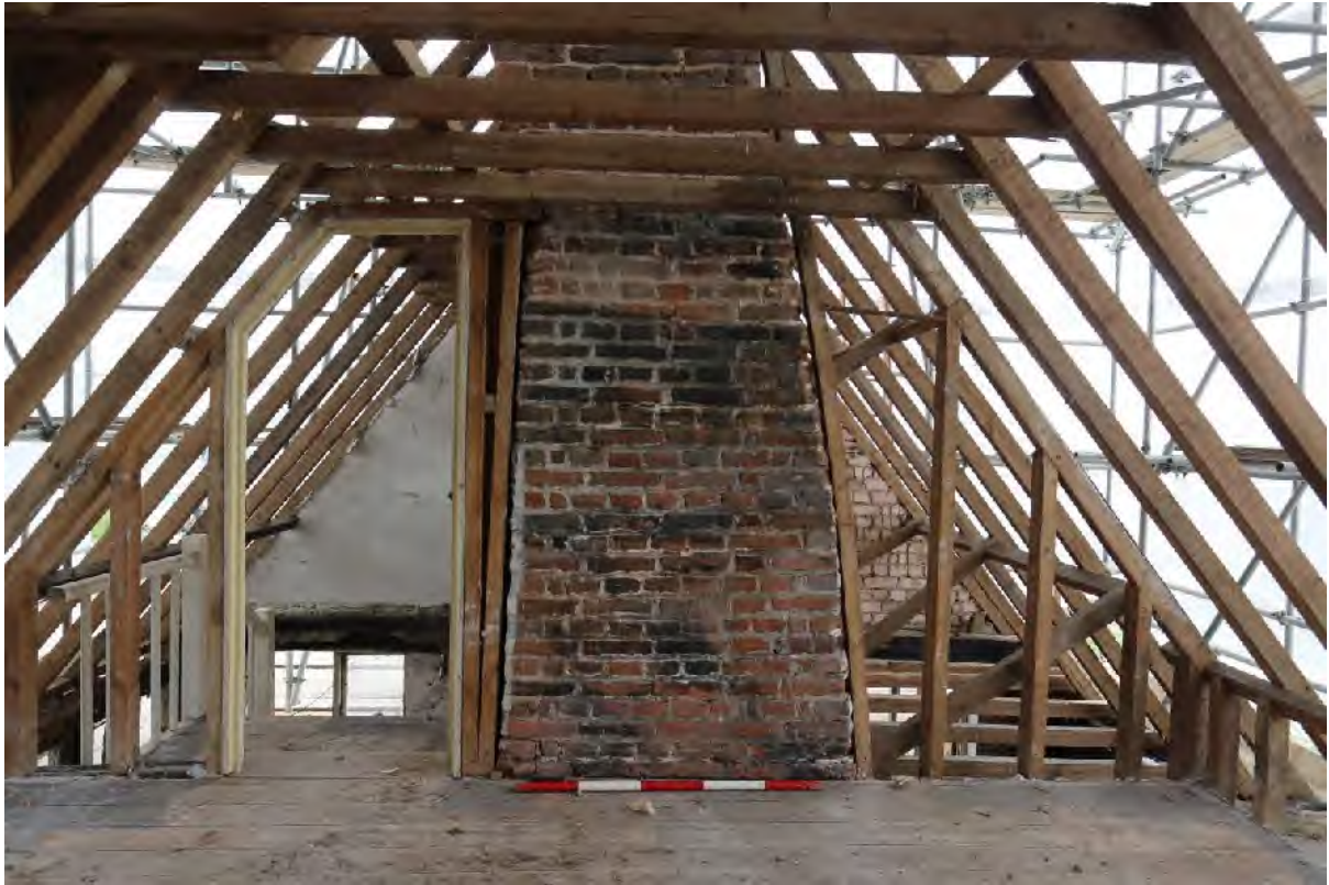
Plate 99 Attic room and brick stack, looking east
