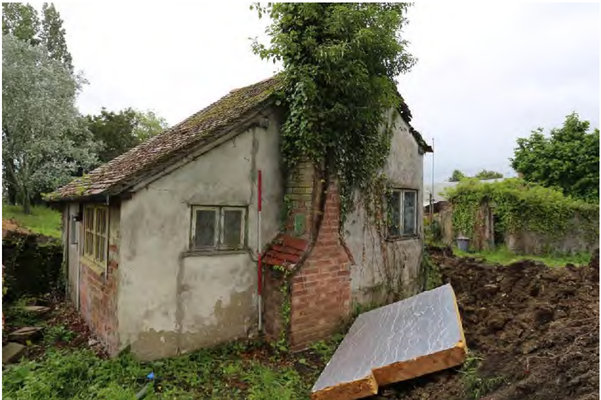
Plate 44 Bothy, looking east
