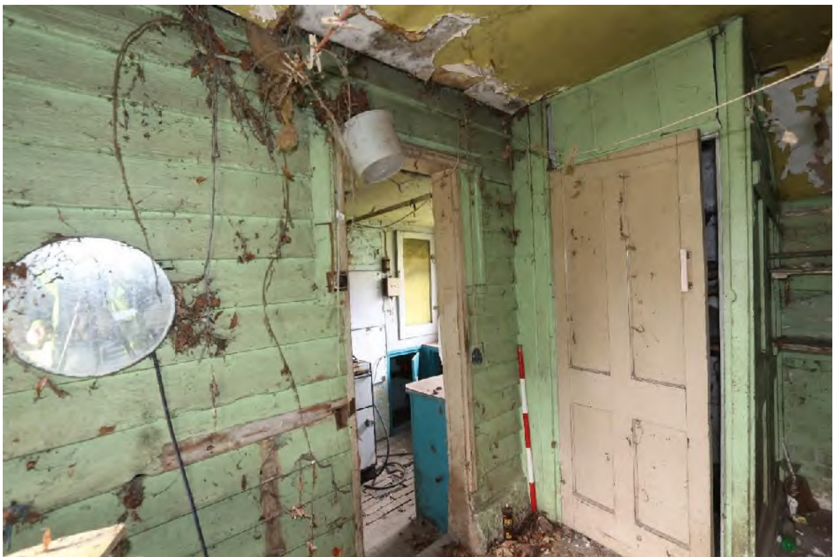
Plate 28 Utility room (G5), showing 'trapped' weatherboard, looking south-west
