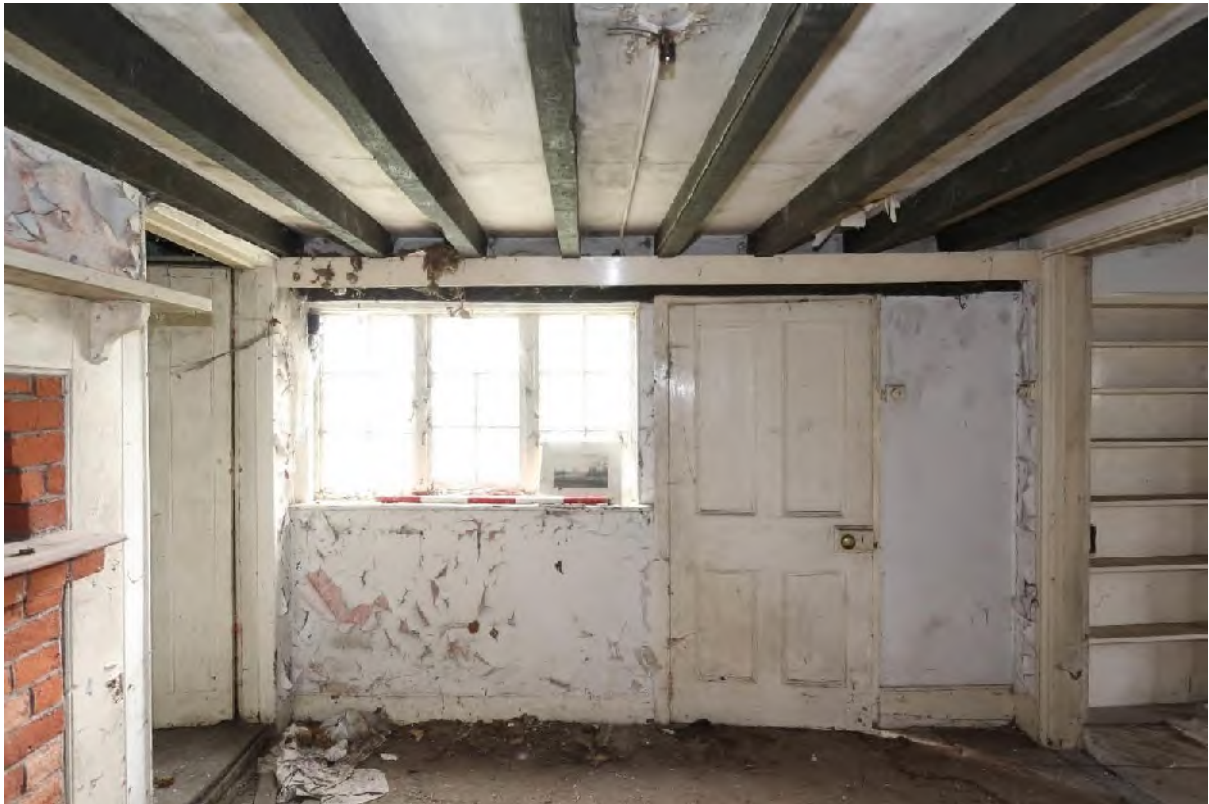
Plate 24 Room (G3) looking east and detailing first floor joists (G3)
