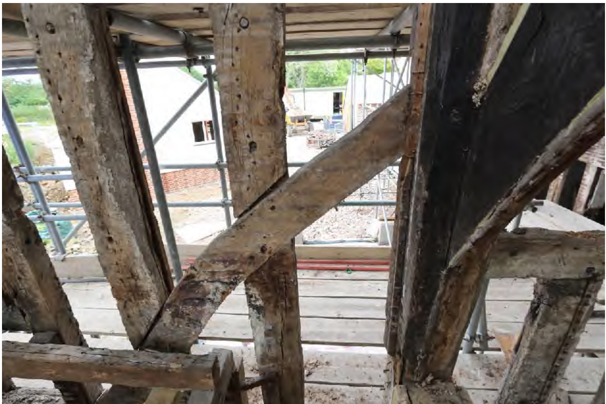
Plate 88 Eastern tension brace in (F7)
