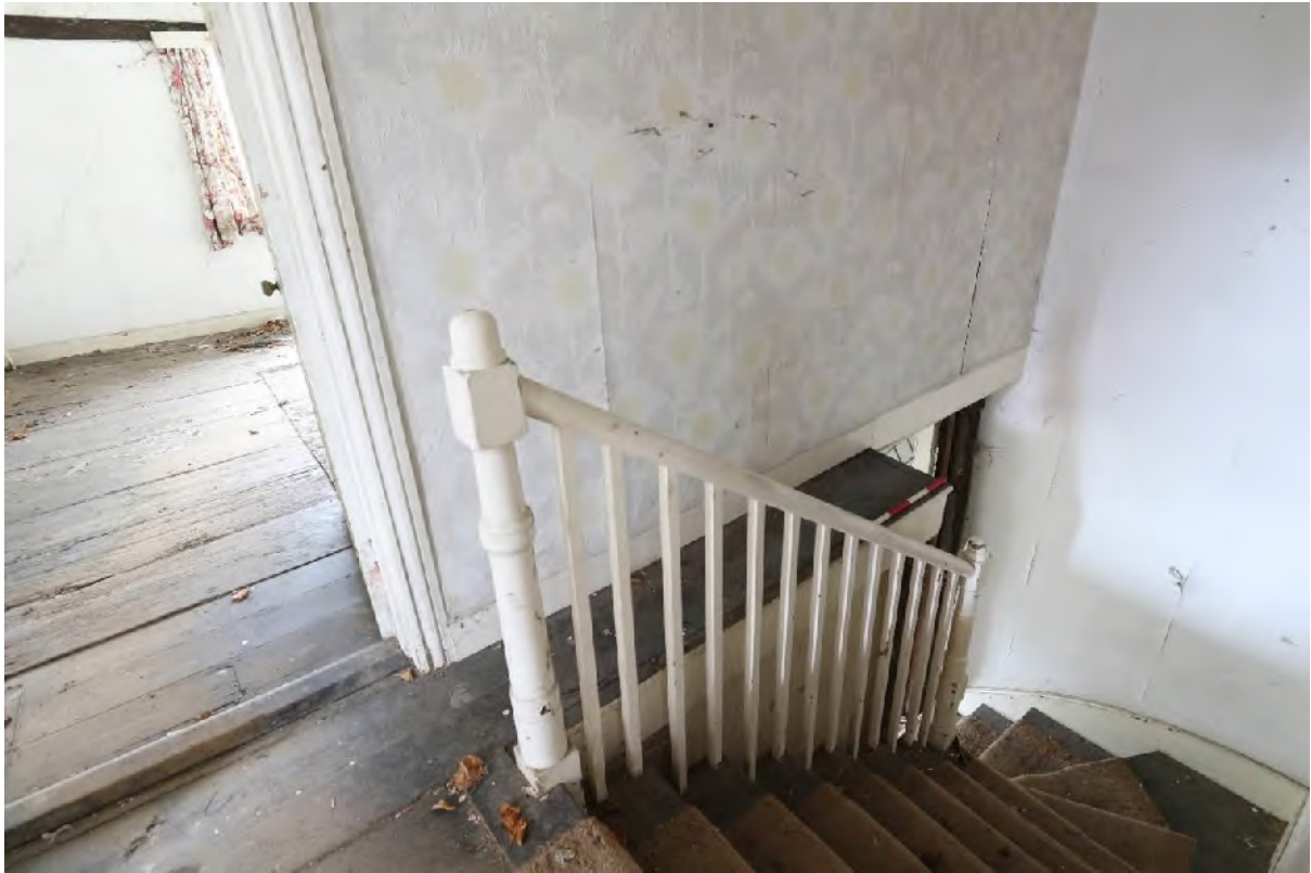
Plate 29 Stair and banister and floorboards in (F1)
