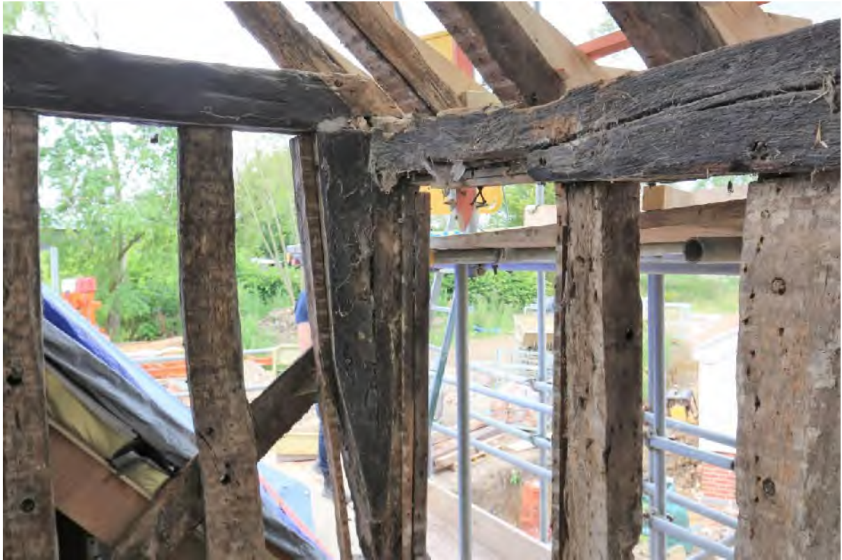
Plate 89 External brace and former window opening, south of north-eastern storey post
