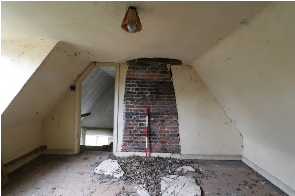
Plate 40 Attic room (A1) looking east
