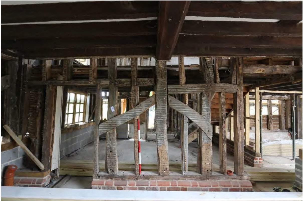
Plate 58 Western wall to (G2) showing downward tension braces and joggled rails
