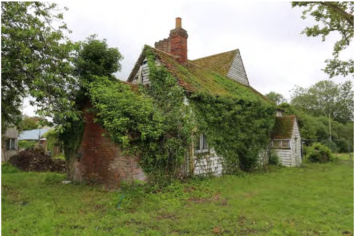
Plate 6 Western elevation, looking south-east
