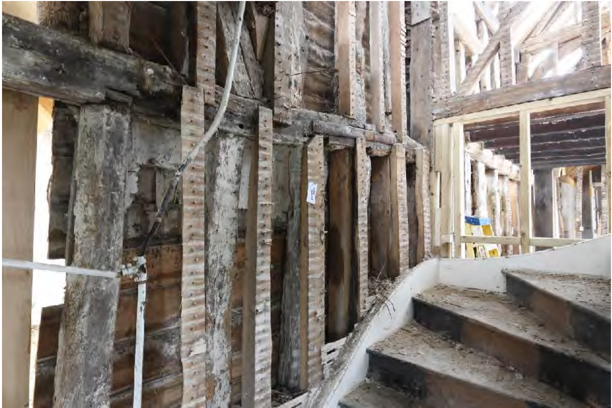
Plate 53 Remnant of wattle and plaster to west side of stair
