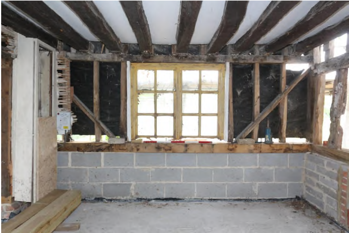
Plate 49 Room (G1) rebuilt southern primary braced wall
