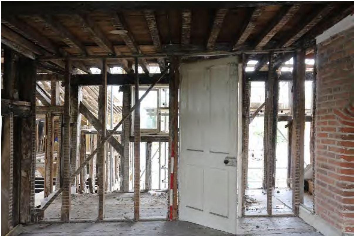
Plate 76 Northern primary braced stud wall to (F2)
