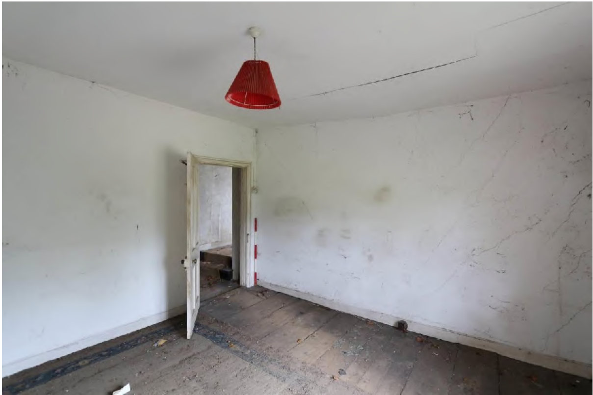
Plate 32 Bedroom (F1) looking north-east
