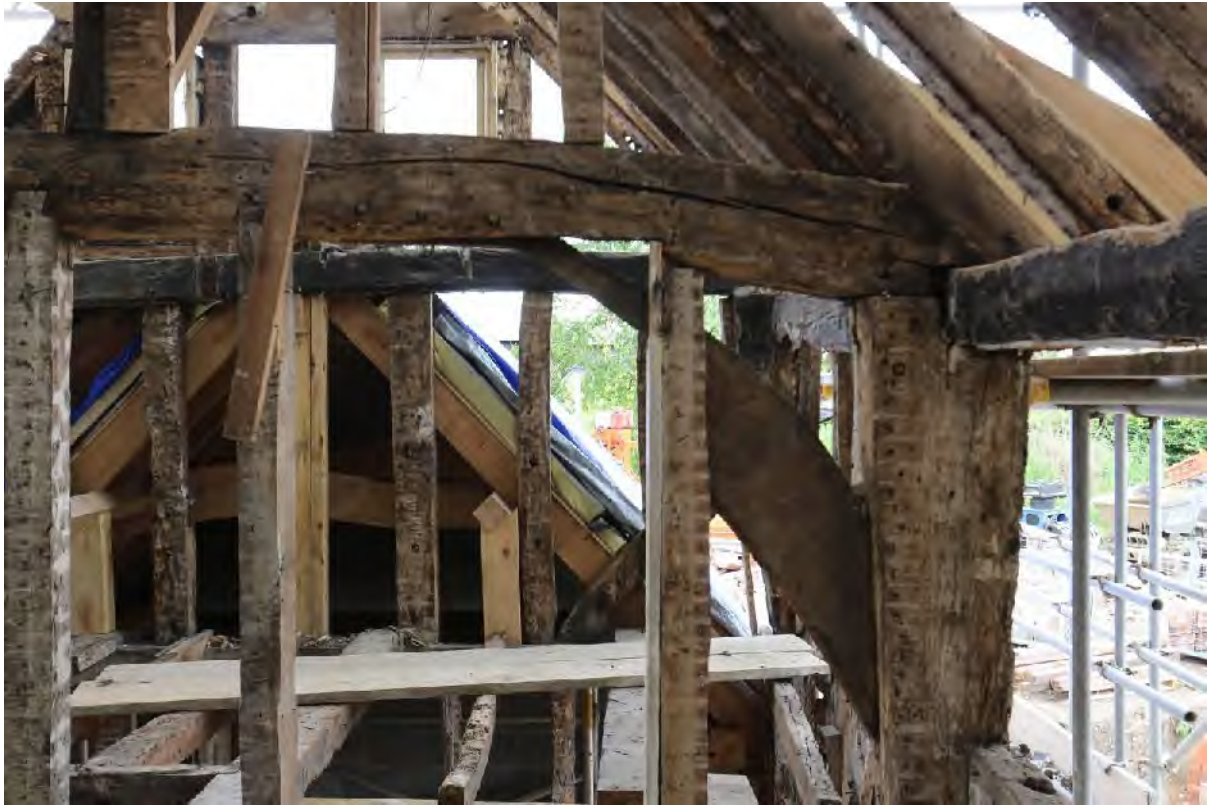
Plate 85 Eastern arch brace cut away to form door opening
