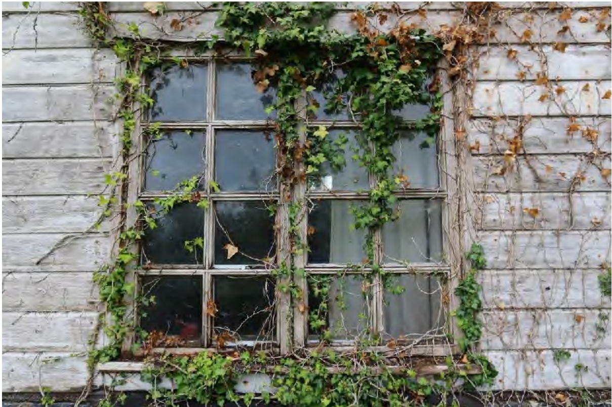
Plate 10 Typical casement in south elevation
