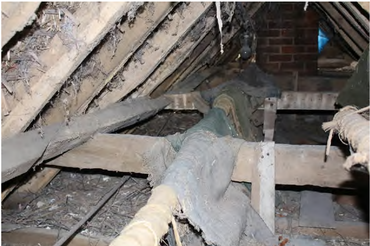
Plate 42 Detail of side purlin roof (middle to northern bays), looking north
