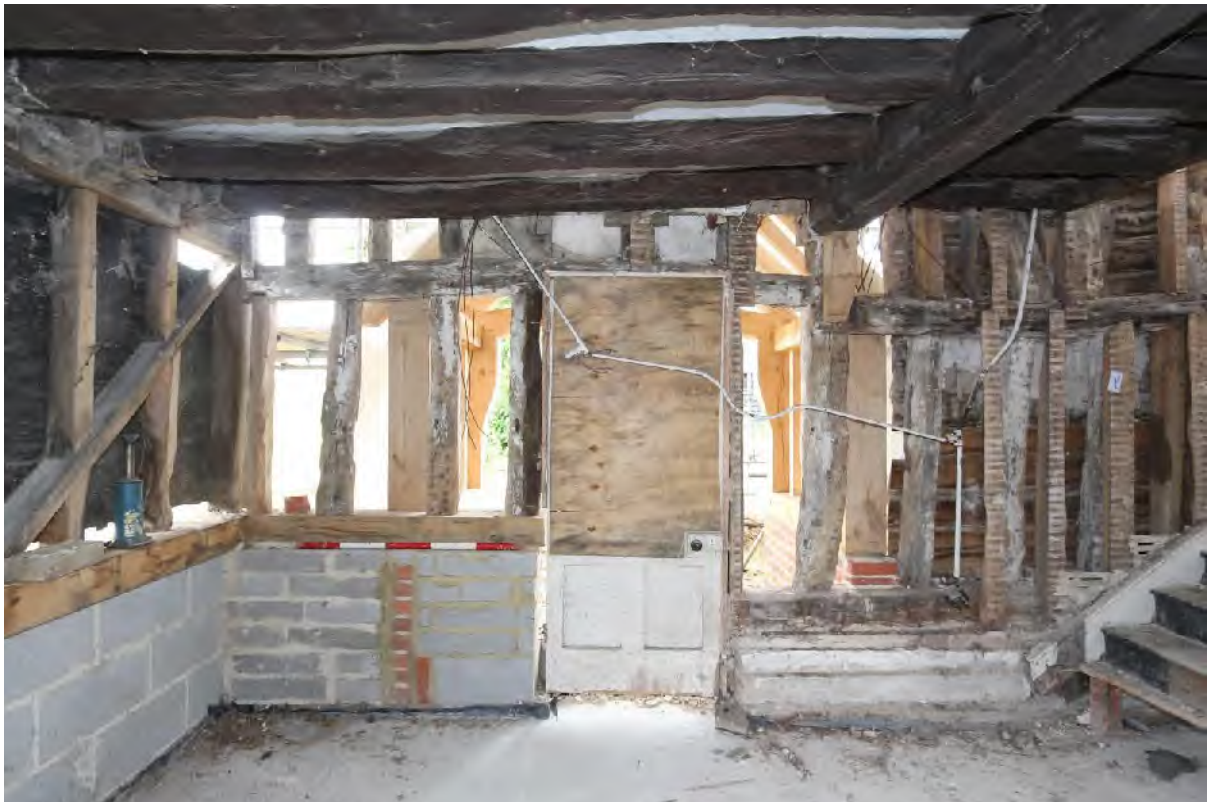
Plate 50 Room (G1), western flank wall
