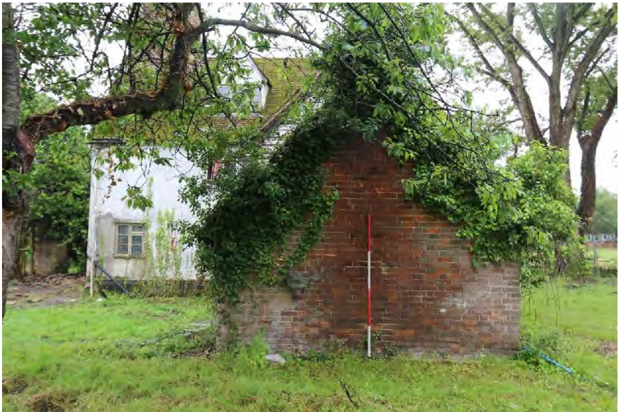
Plate 4 Northern elevation, extension, looking south
