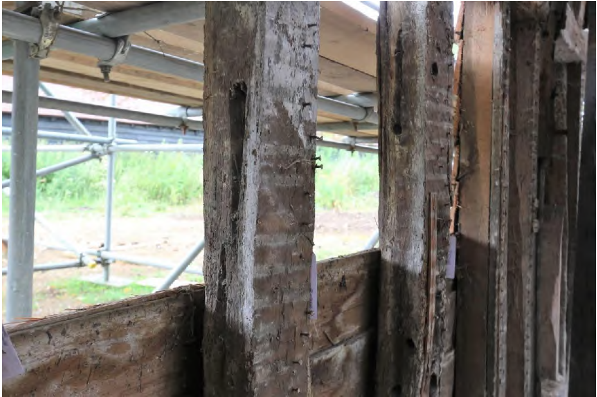
Plate 51 Wattle features cut into opposing faces of wall studding
