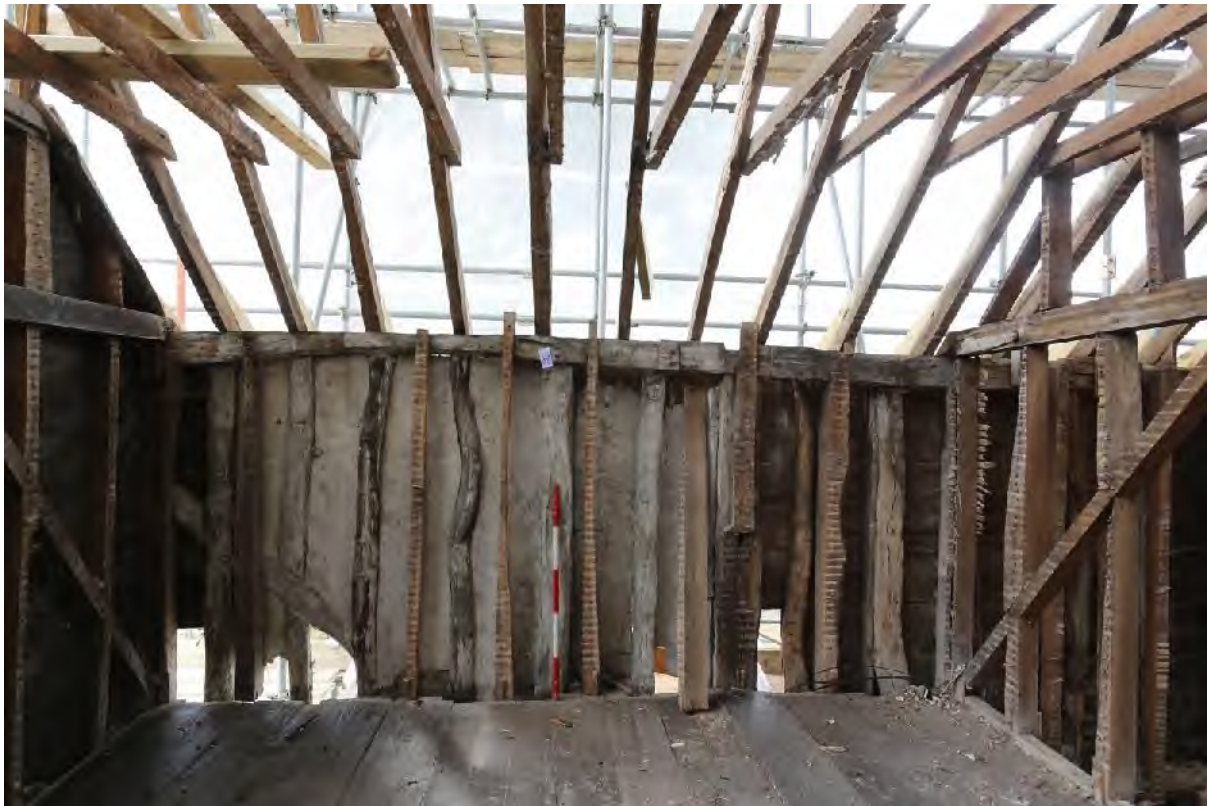
Plate 70 Western wall to (F1) showing tension brace and off-centre storey post
