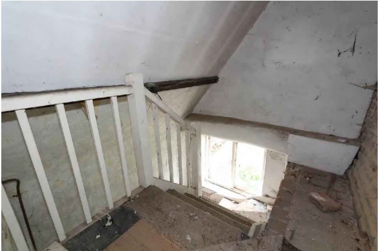
Plate 39 Attic stair looking east
