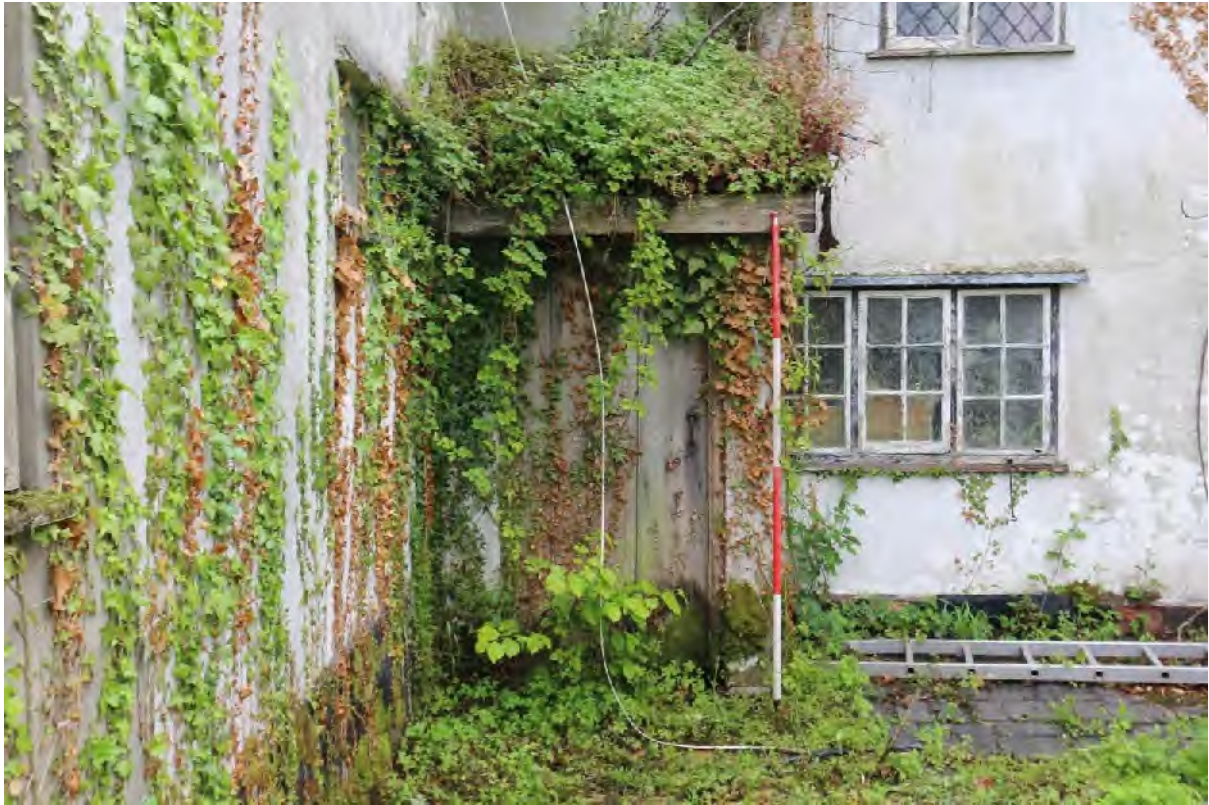
Plate 11 Lean-to porch and 19 th century casement, eastern elevation, looking west
