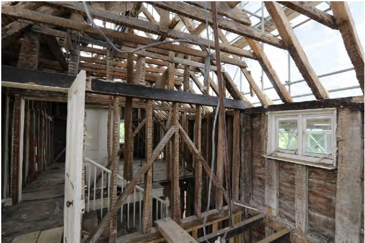
Plate 86 Primary braced south wall to (F6)
