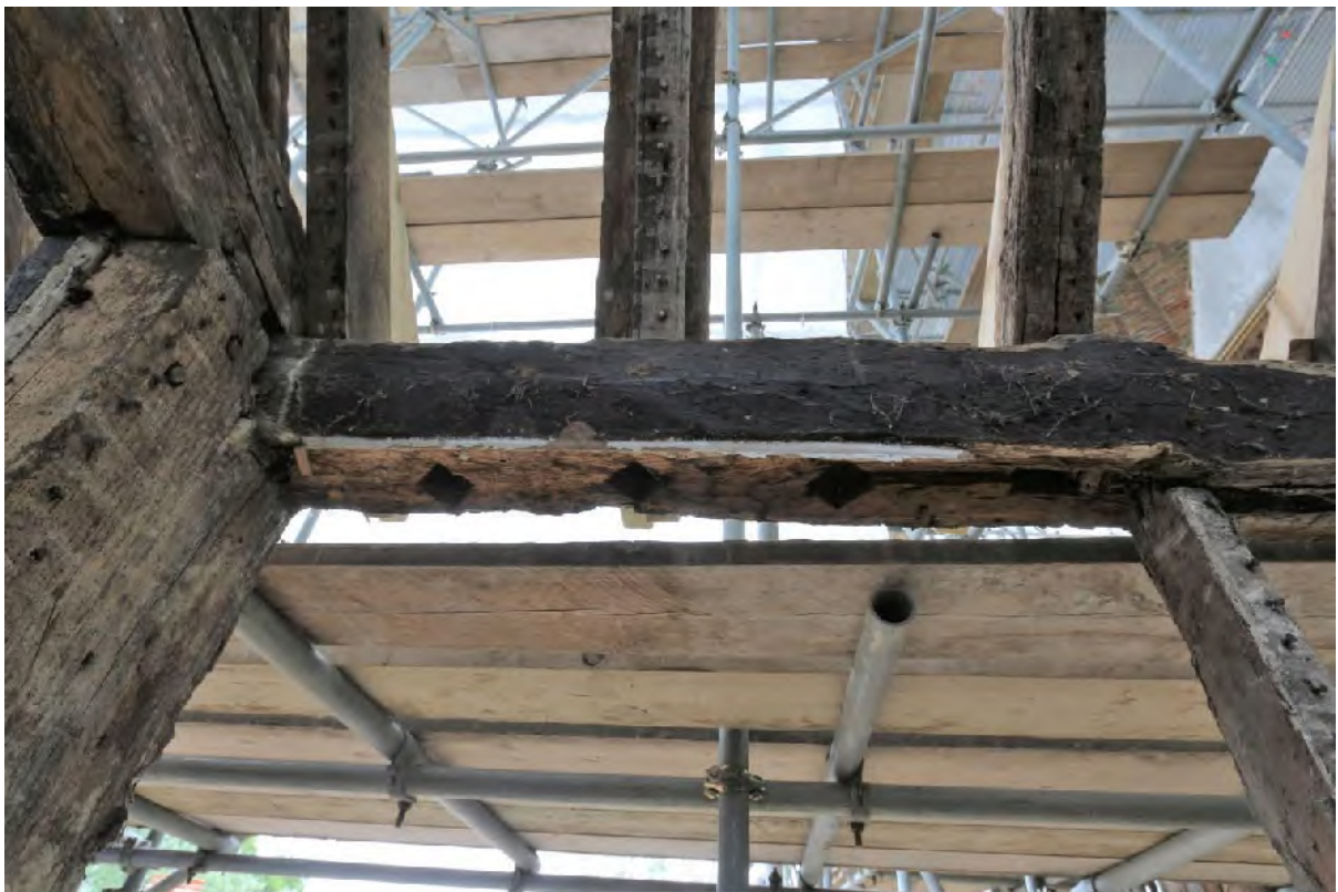
Plate 82 Evidence of diamond mullion window in east wall of (F5)
