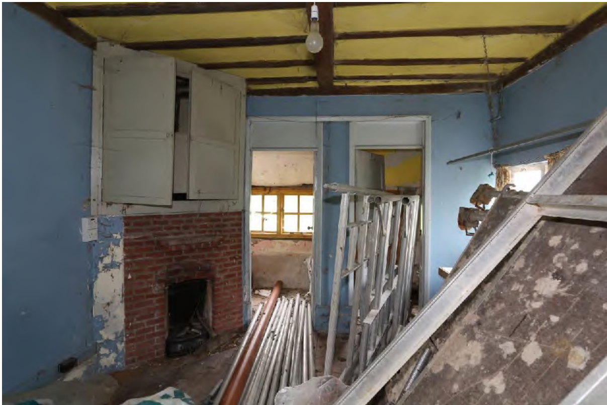
Plate 46 Bothy (B1) looking north-west
