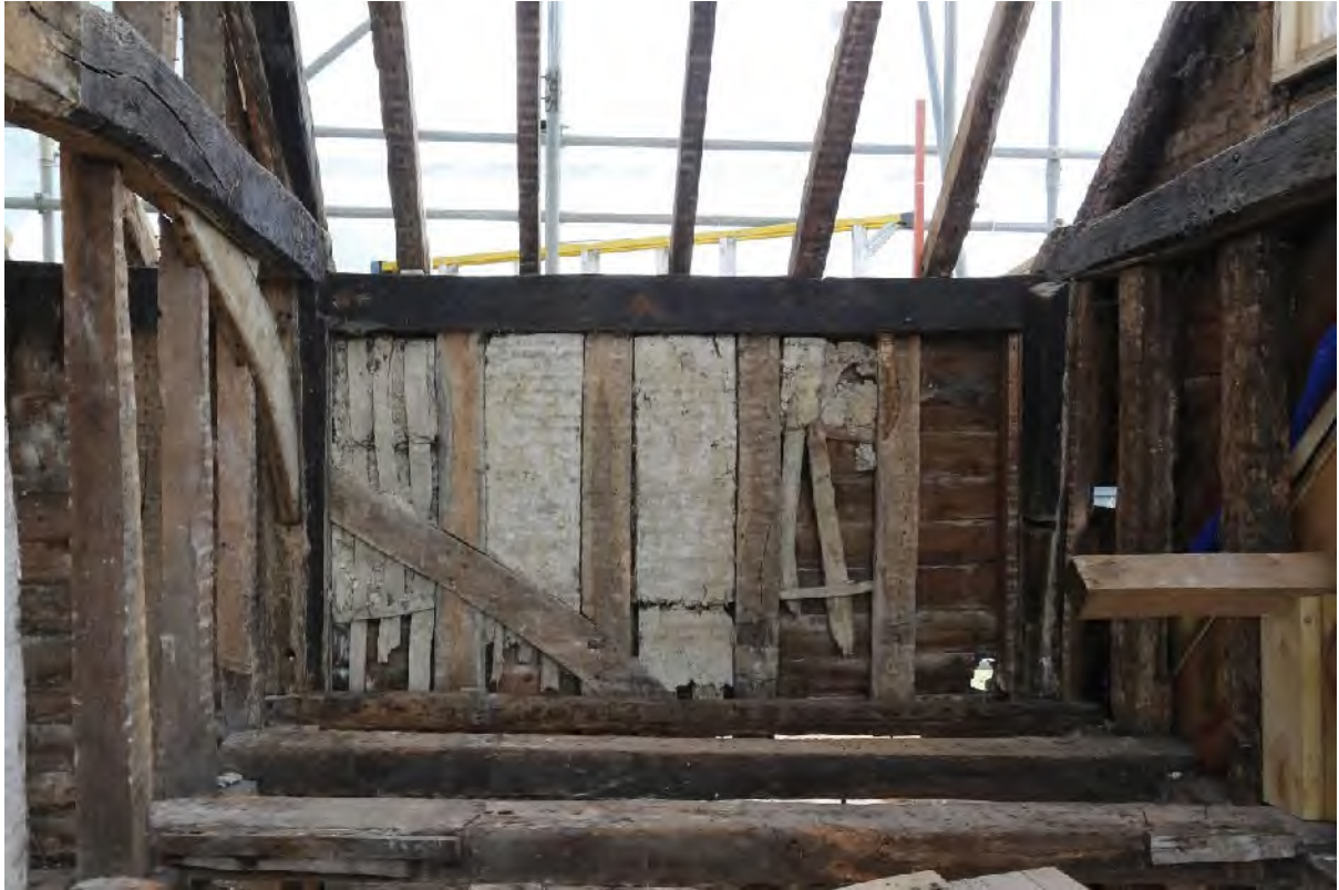
Plate 87 Western wall of (F7) showing arch brace and internal tension brace
