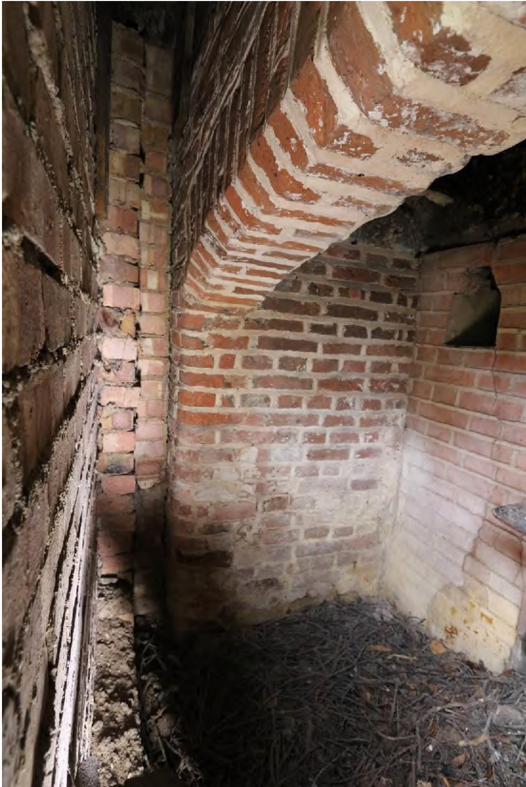
Plate 7 Inglenook fireplace behind Fletton blocking wall (left), east elevation
