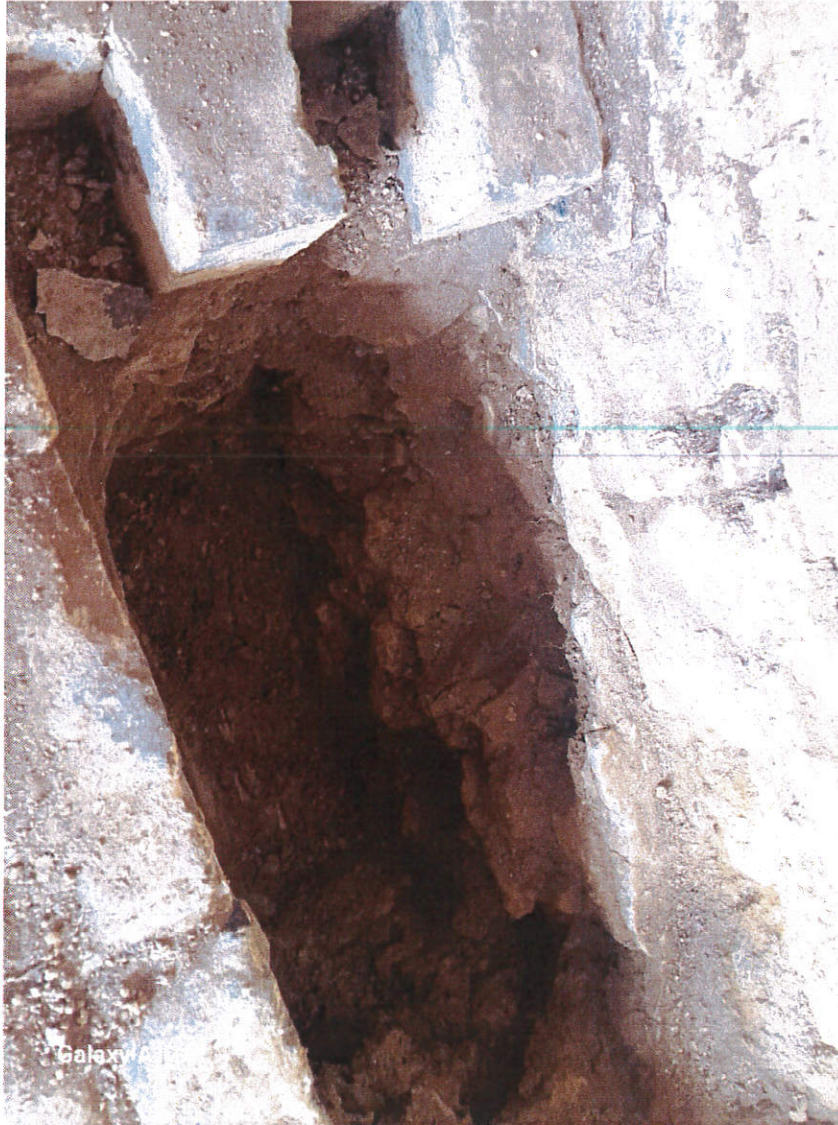
Trial Pit Showing Fractured Limestone.
