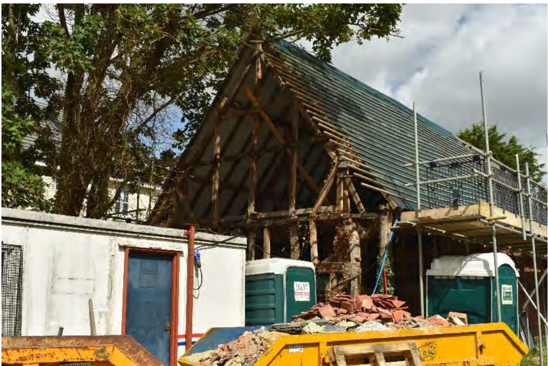
20 Framing of southern gable
