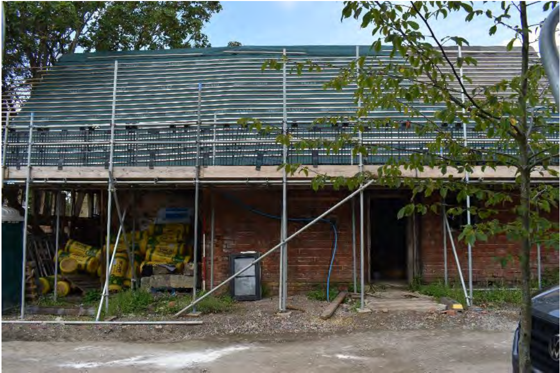
19 East elevation, August 2023
