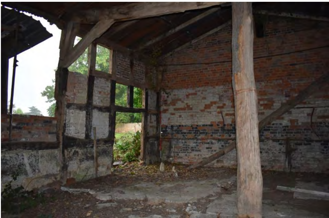
10 Interior of the barn, with concreted floor and partly painted walls and timber framing
