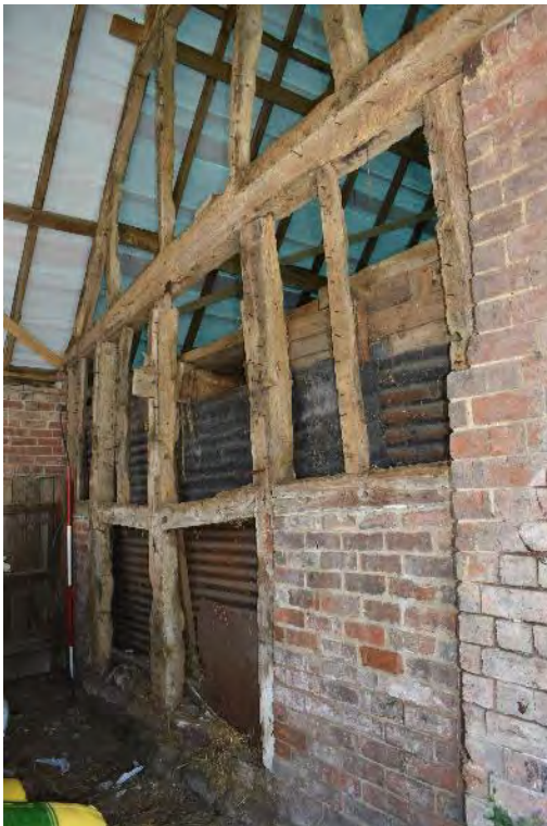
33 Cross wall in 2023, boarding etc removed
