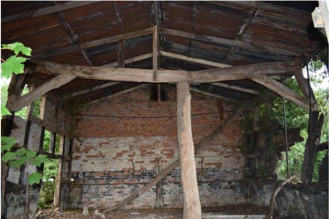
11 Brick gable wall with mull pitching window near apex
