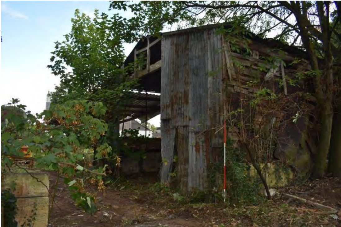
9 Former internal bay division, subsequently covered with corrugated iron sheeting
