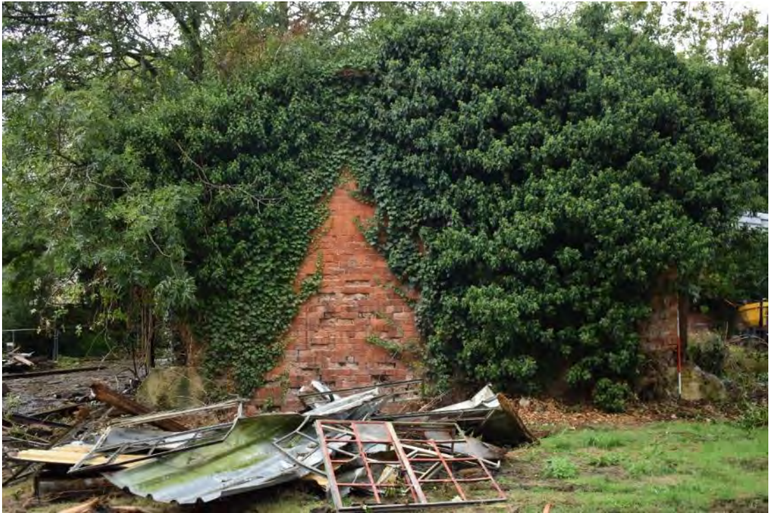
5 Brick gable, overgrown with ivy
