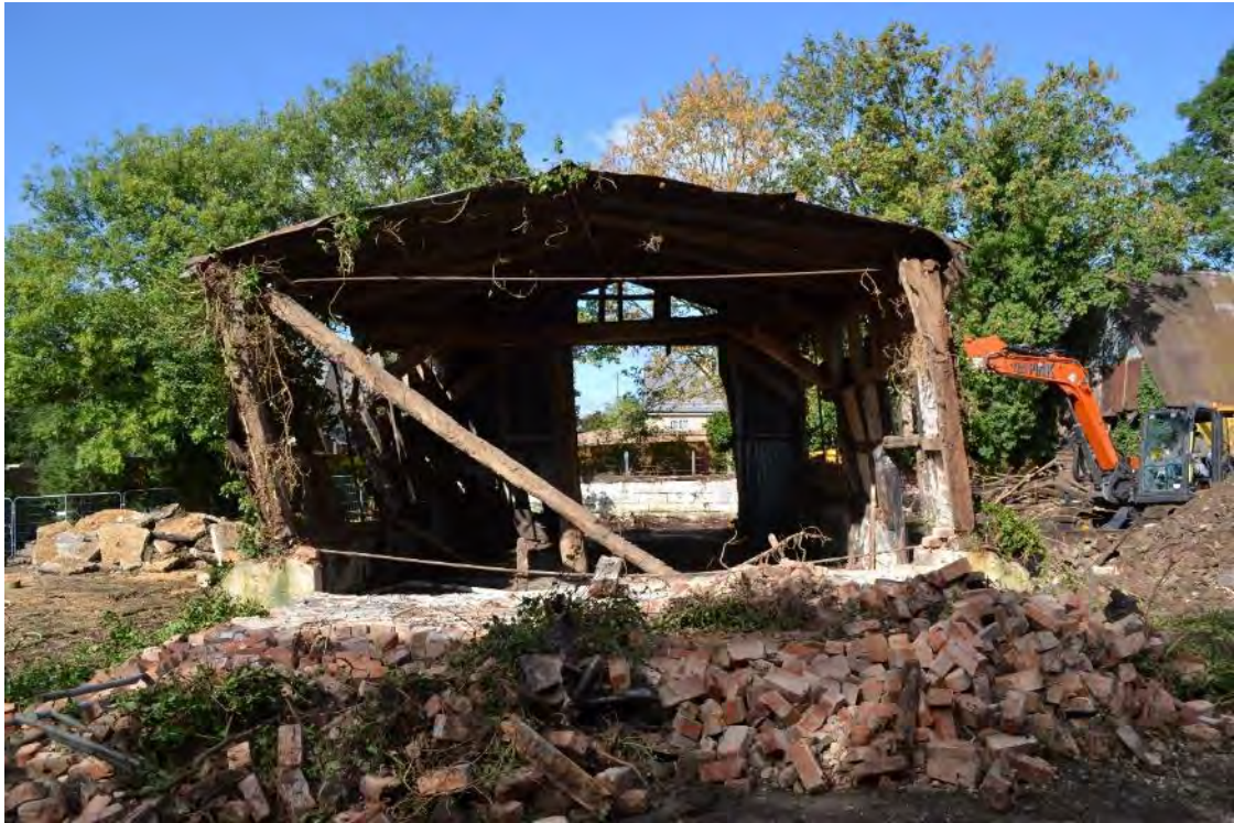
44 Start of demolition of barn
