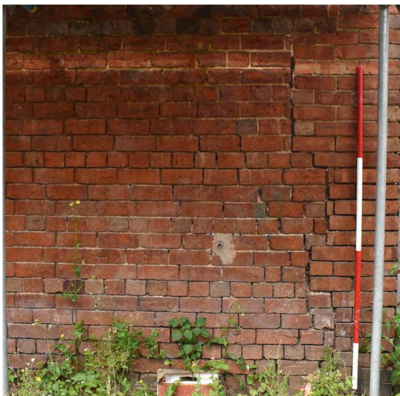
25 Change of brickwork at north-east corner
