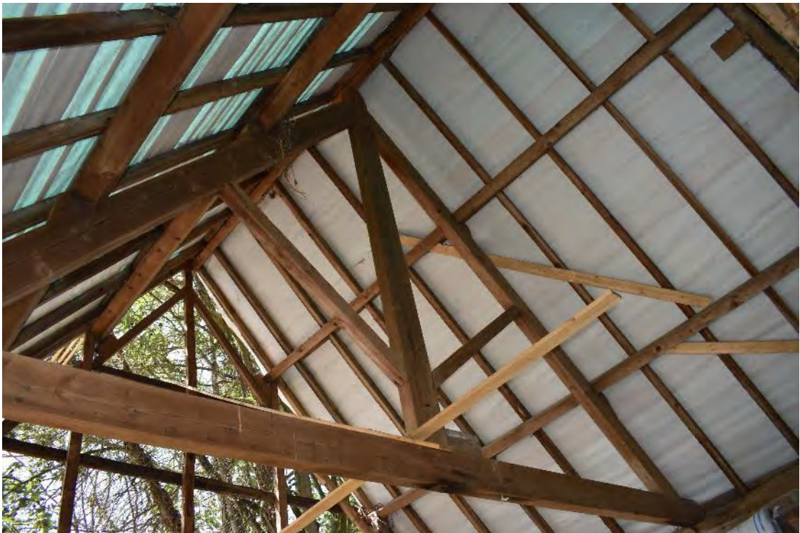
37 Machine-cut, bolted king-post truss with new purlins and rafters
