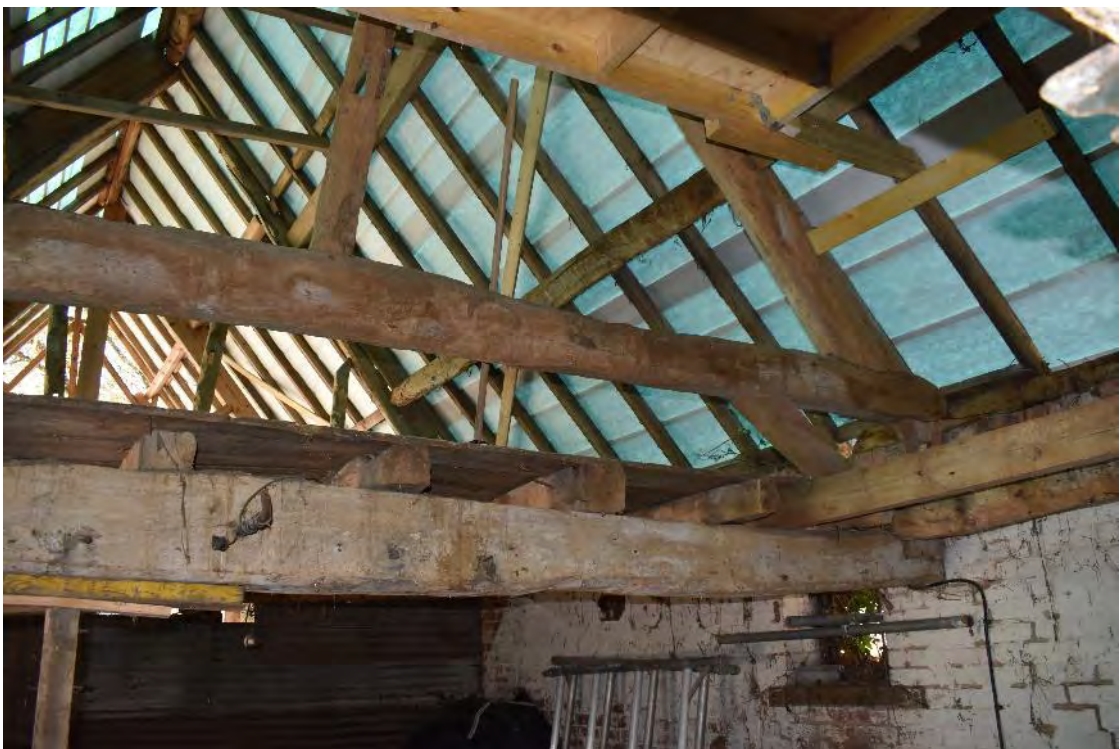
41 Central roof truss above floored level in southern part of room
