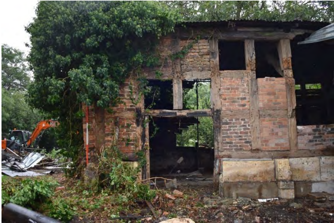
3 Box framing on north-east side of barn
