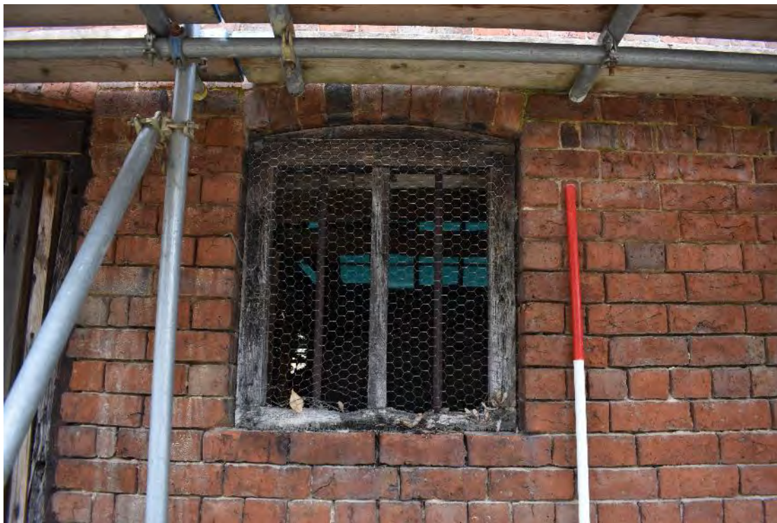
24 Window on east wall
