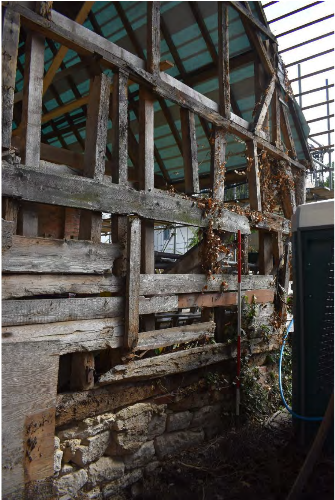
21 Southern gable with weatherboarding and stone plinth
