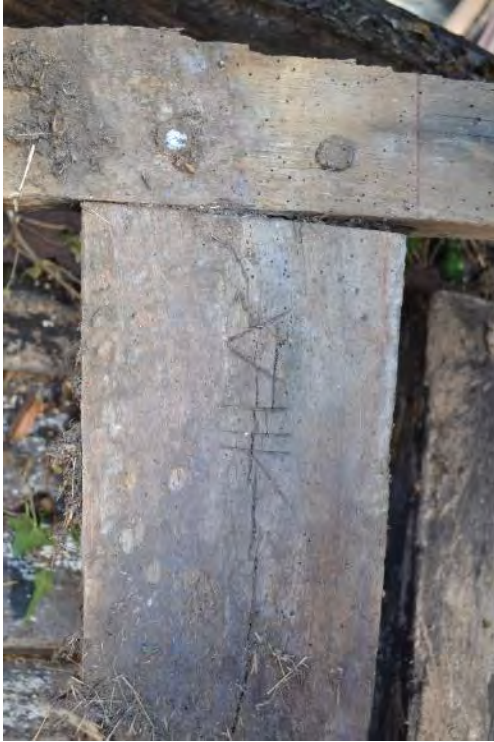
46 Carpenter's mark on timber of demolished barn
