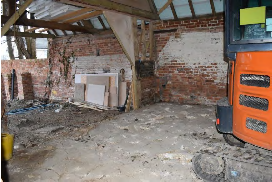
50 Stripped-out interior of Building L, concrete broken up
