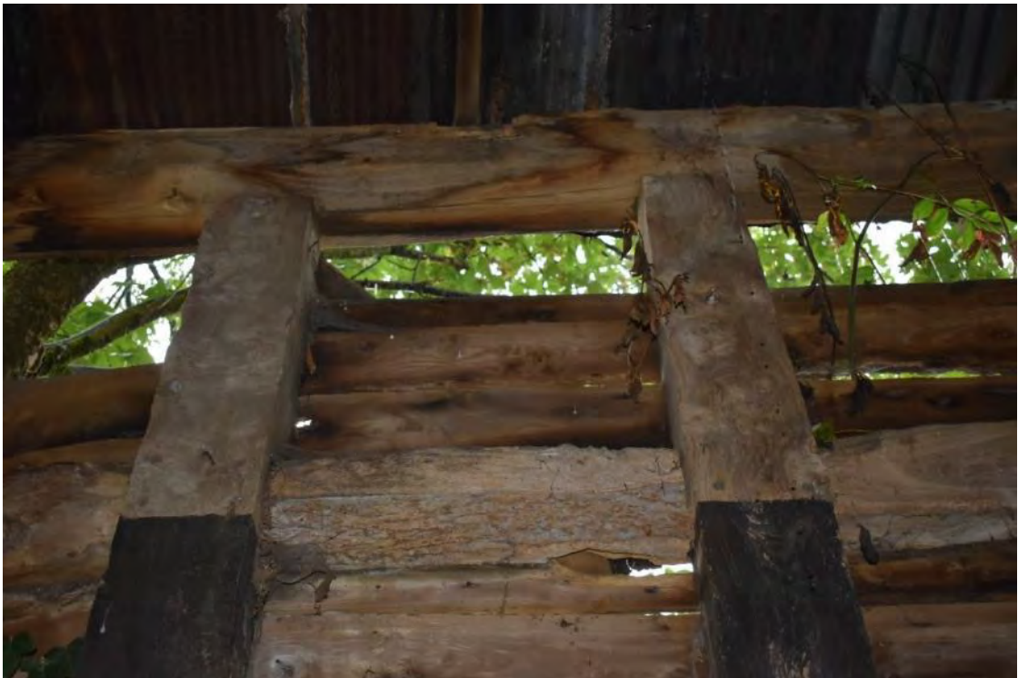
14 Underside of framing with bark below timber
