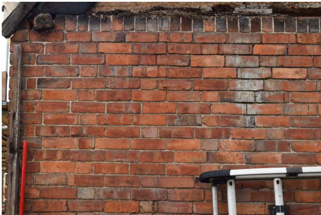
26 Flemish Garden Wall Bond brickwork in north gable
