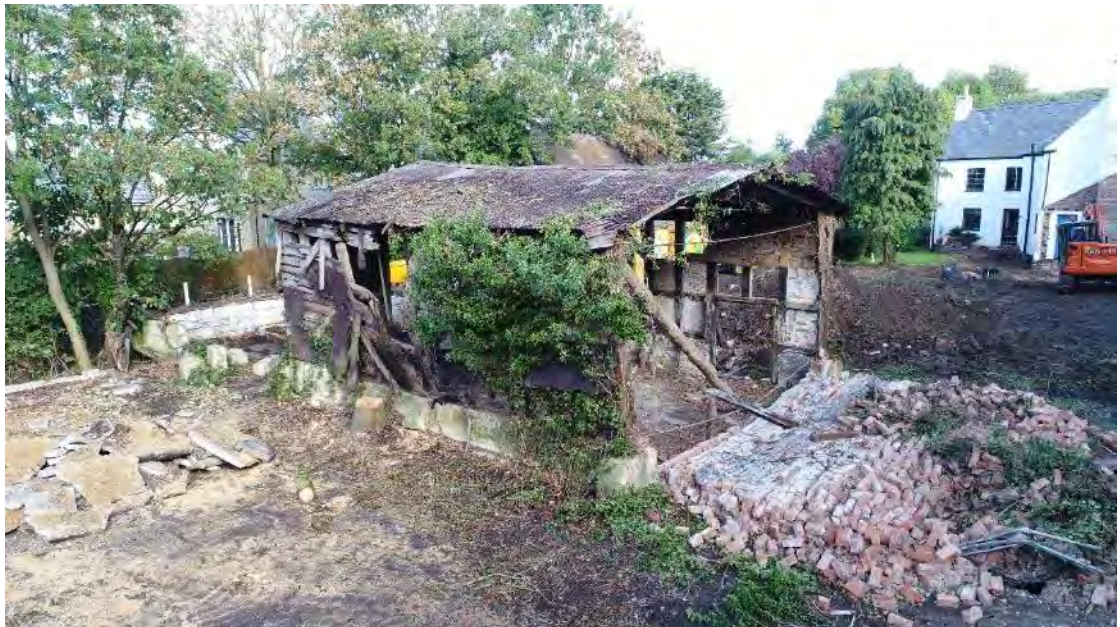
43 Drone shot of Barn prior to demolition
