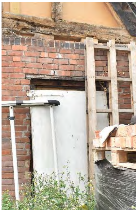
27 Inserted door on north gable wall
