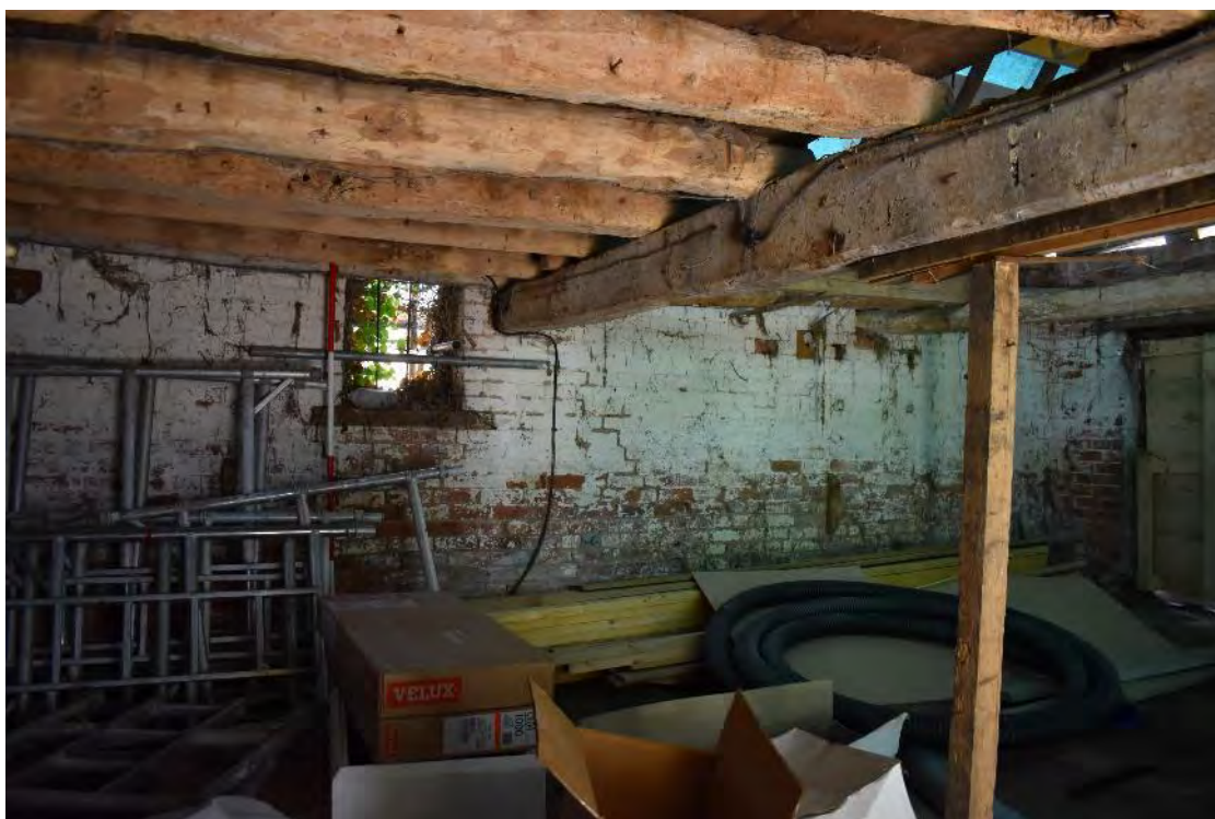
39 Chamfered girder and floor joists
