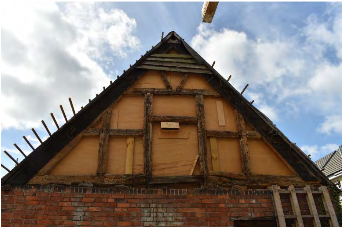
29 Timber framing in upper part of north gable
