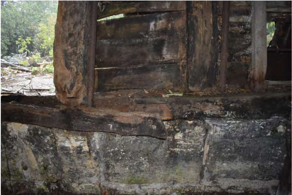
13 Half-jointed sill beam with face pegs
