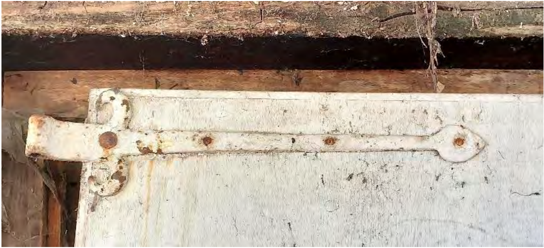
28 Old strap hinge on later north door
