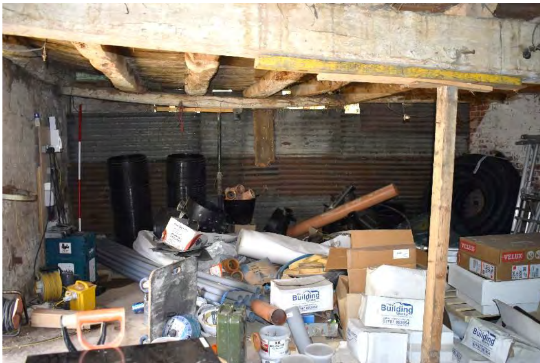
38 Corrugated iron covered wall at south end
