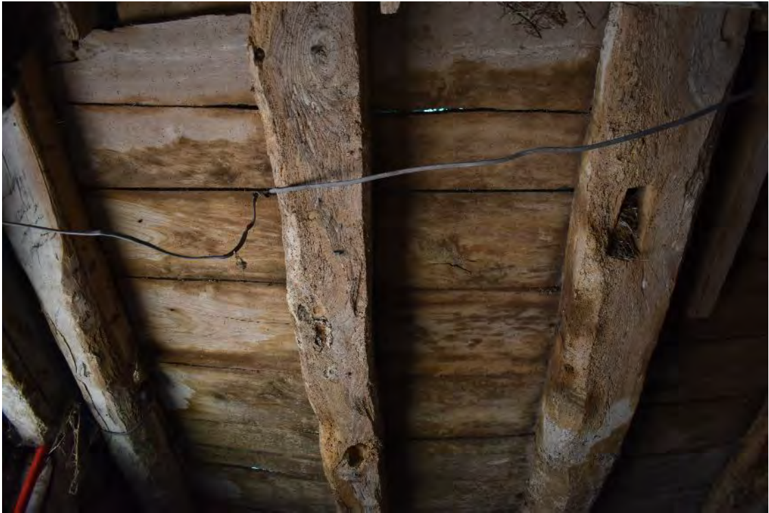
40 Old floorboards and re-used timbers for joists
