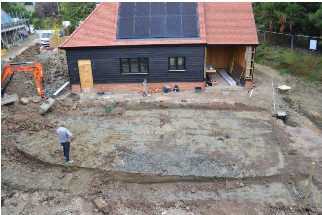
49 Area stripped to natural clay for attenuation tank, looking north-east
