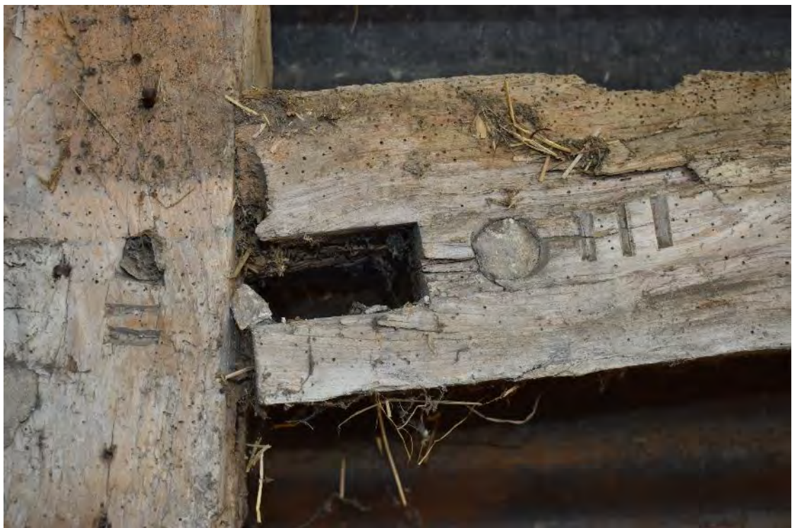
35 Carpentry marks III, infilled hole and open mortise
