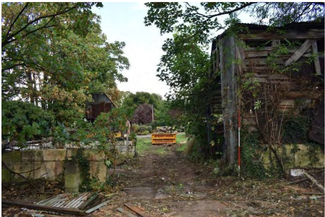
8 Bay of former threshing floor
