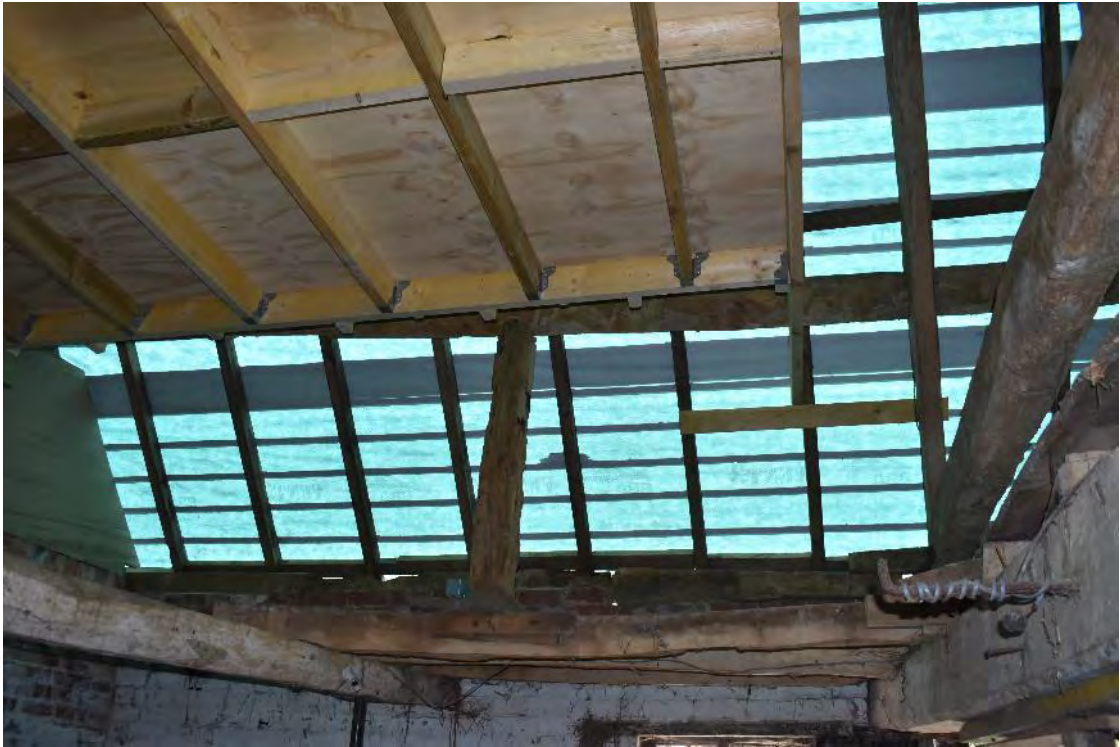
42 Modern bat roost above formerly floored area in north part of room, old timbers below
