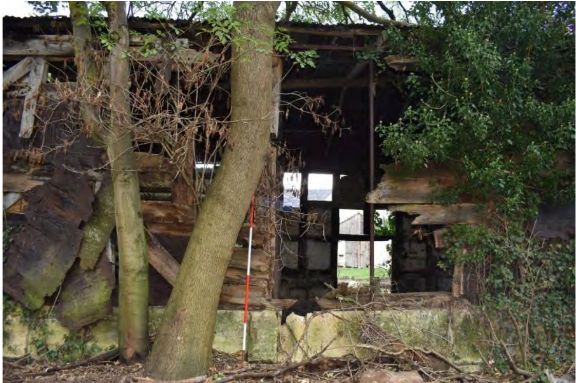
7 South-west side of the building with timber framing replaced by iron pile
