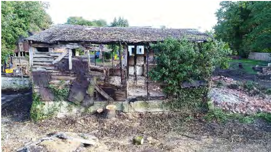
4 Weatherboarded south-west side of barn after removal of trees
