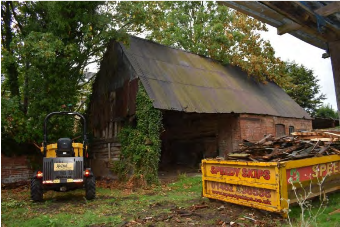
17 Building L, southern gable, September 2022
