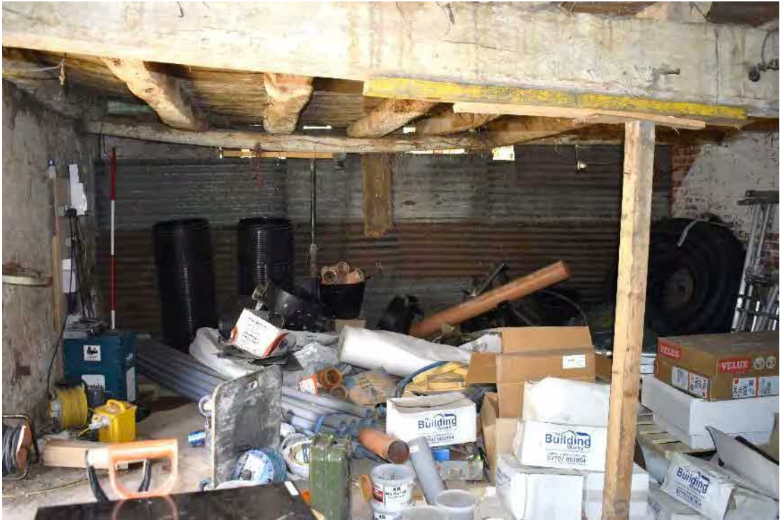
38 Corrugated iron covered wall at south end
