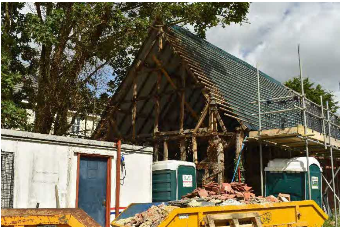
20 Framing of southern gable
