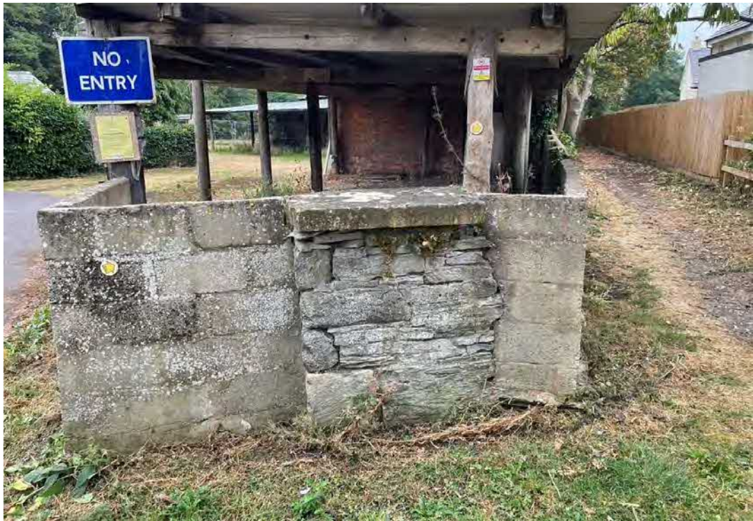
54 Section of stone walling of former building or boundary wall at north end of site, surrounded by breeze blocks of Building M, looking south
