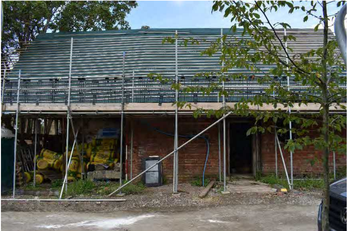
19 East elevation, August 2023
