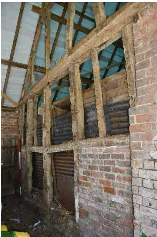
33 Cross wall in 2023, boarding etc removed
