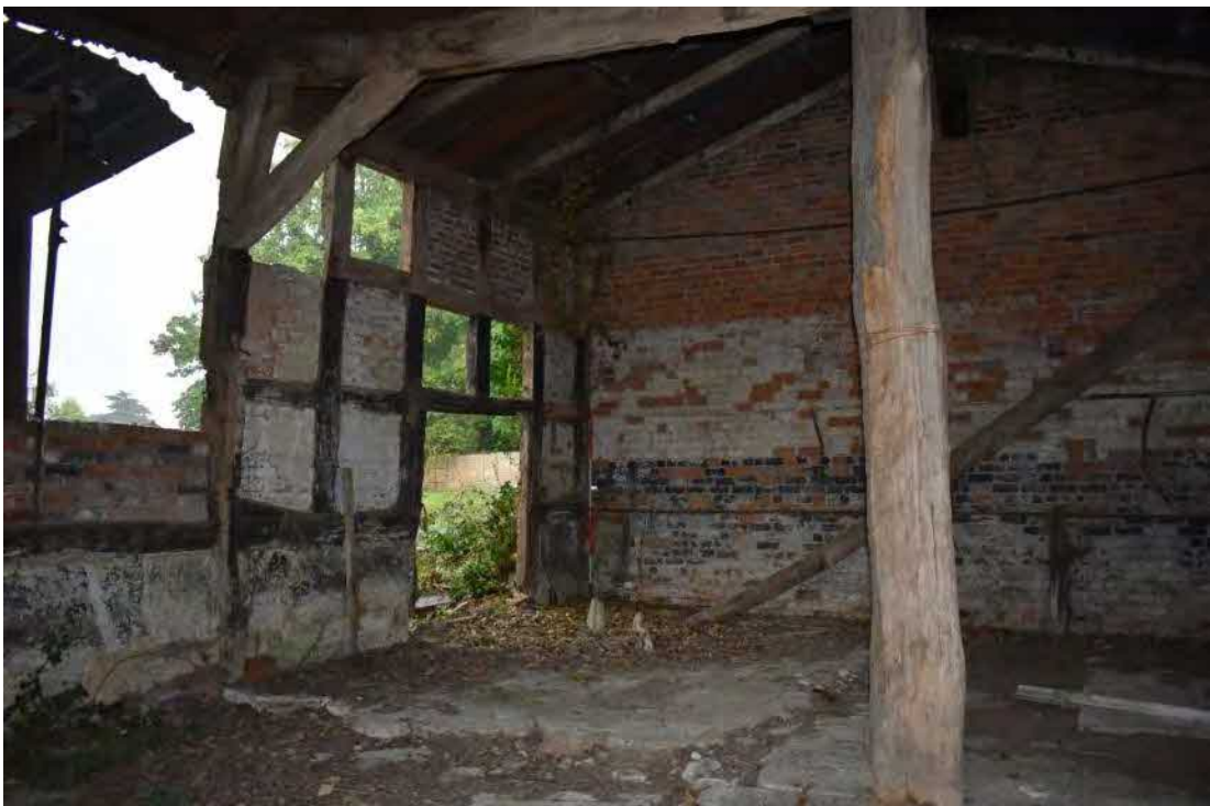
10 Interior of the barn, with concreted floor and partly painted walls and timber framing
