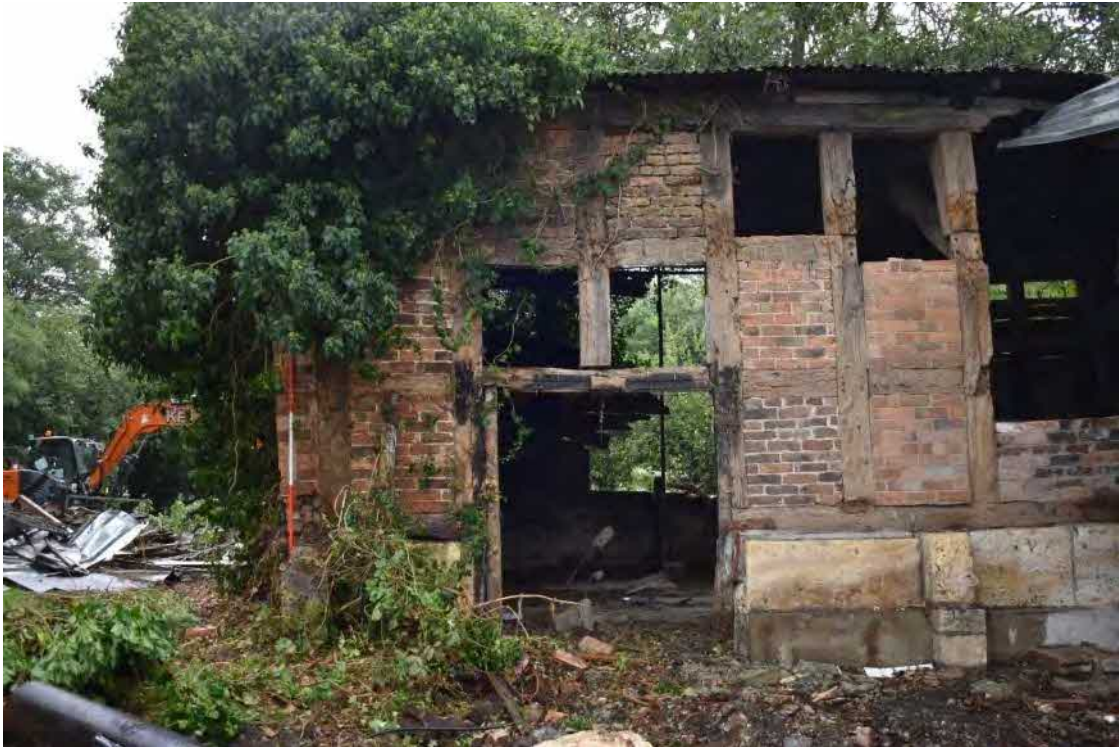
3 Box framing on north-east side of barn
