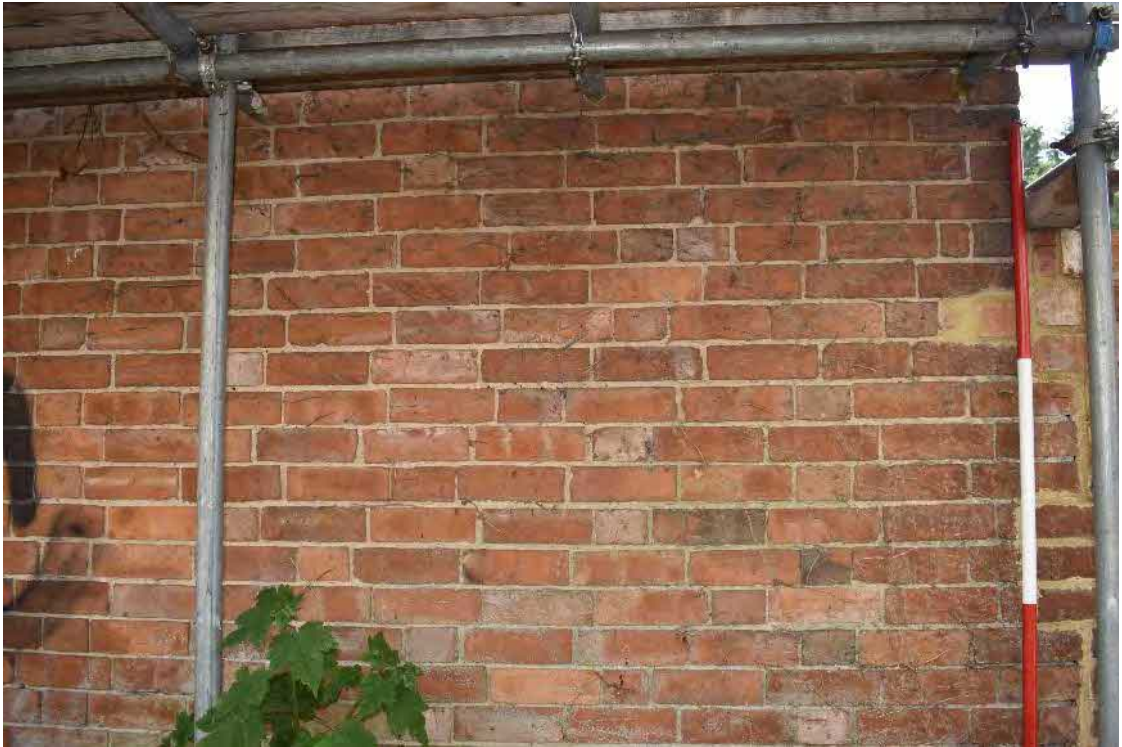
30 Brickwork of west wall, largely Flemish Garden Wall Bond
