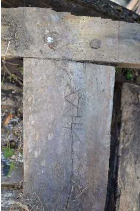
46 Carpenter's mark on timber of demolished barn
