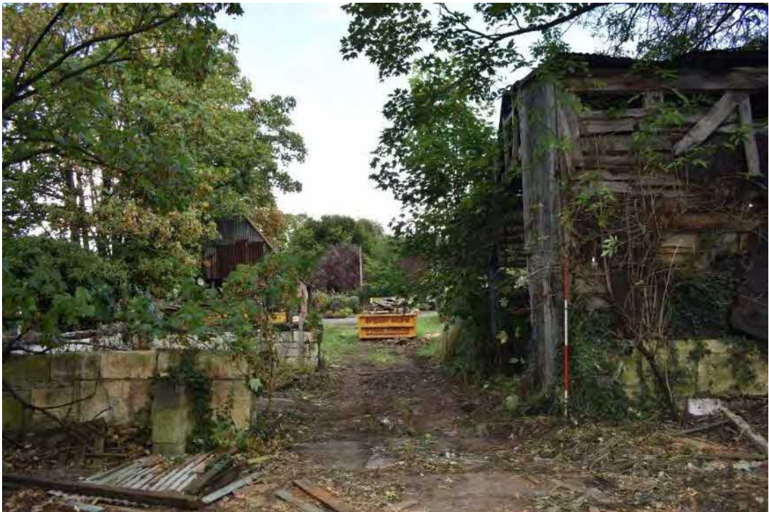
8 Bay of former threshing floor
