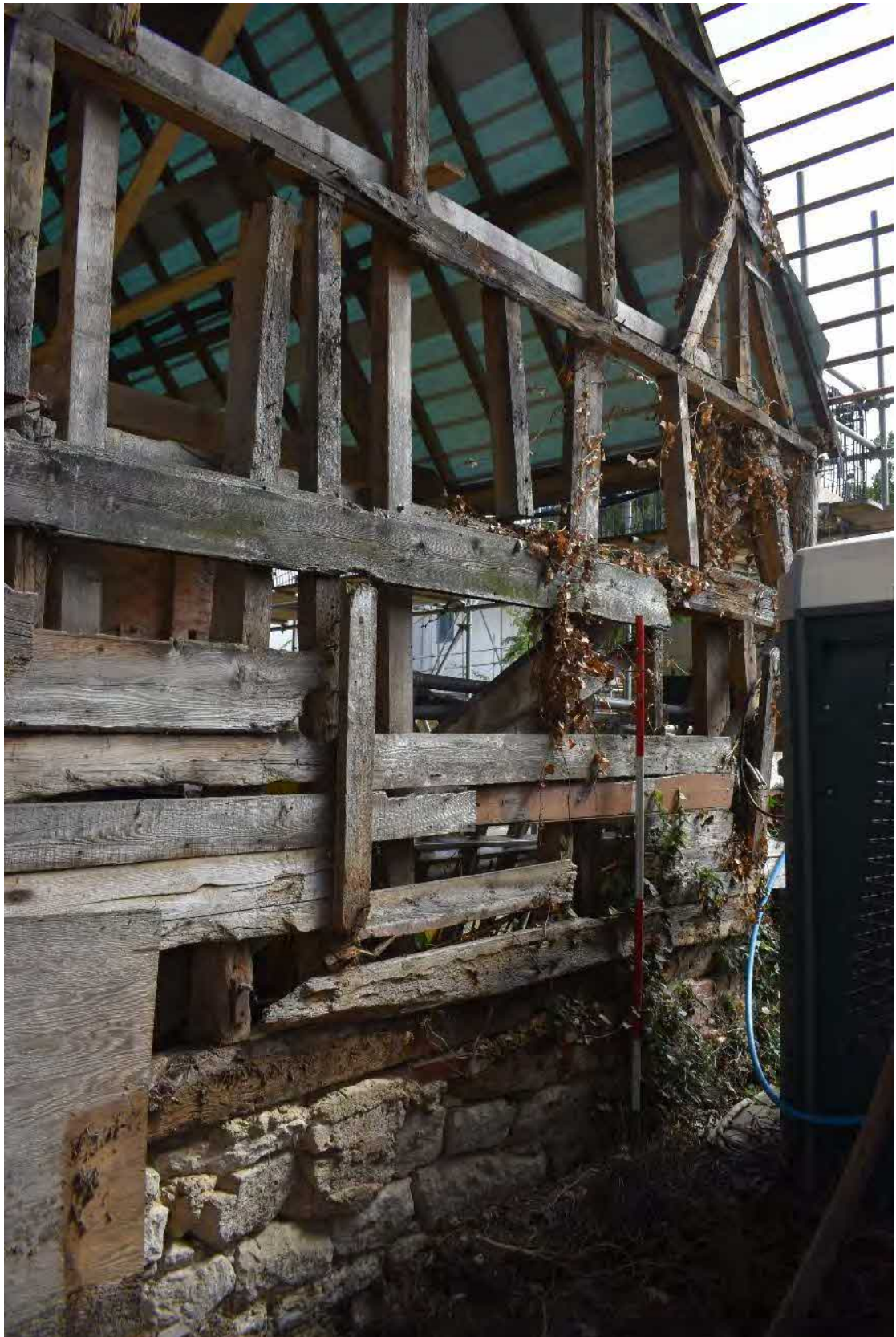
21 Southern gable with weatherboarding and stone plinth
