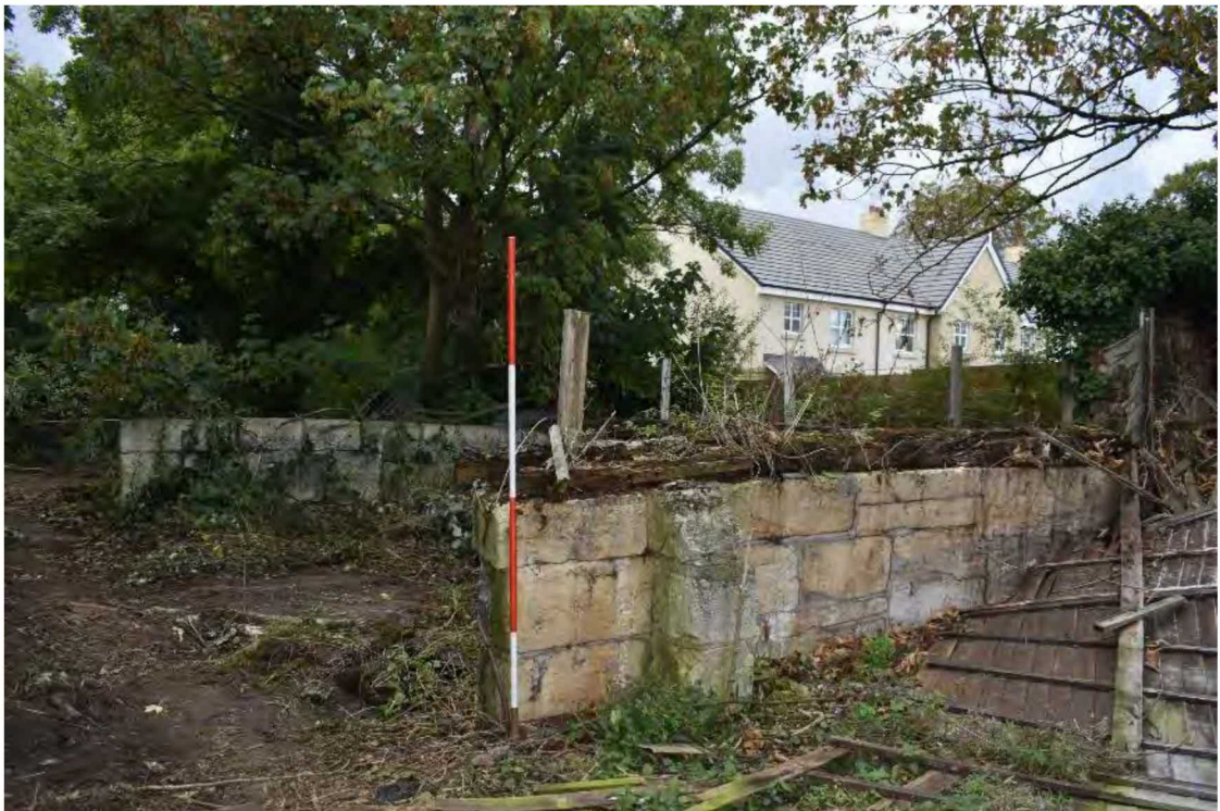
2 Stone plinth of western part of building, without superstructure
