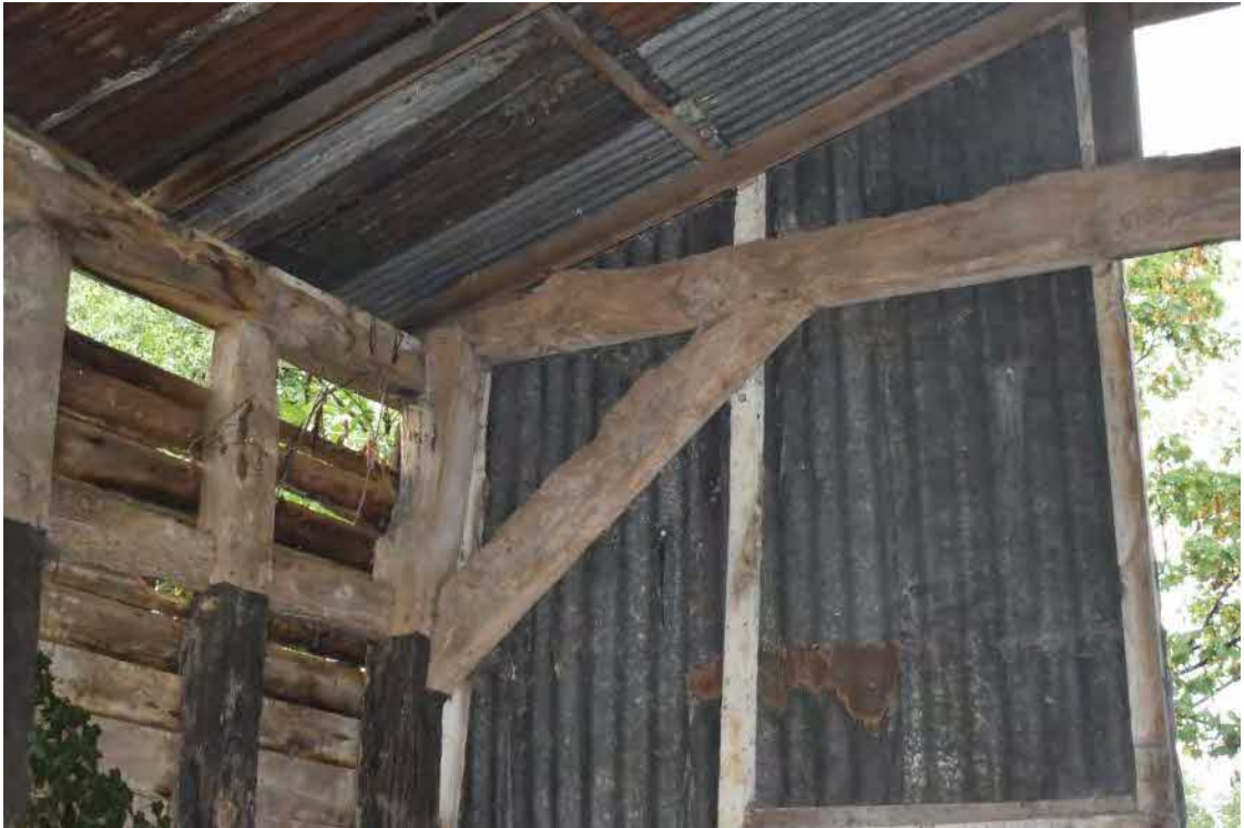
15 Detail of brace with mortise and tenon joints, triple pegged
