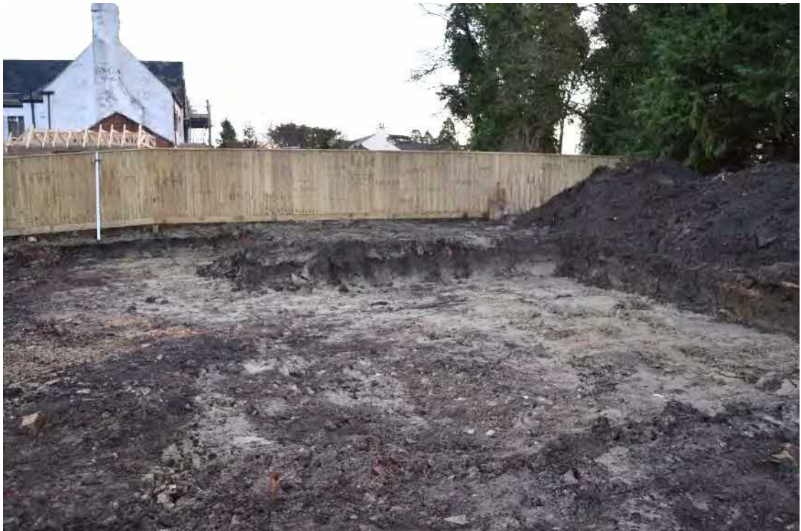
47 Area stripped for first house plot to south of farmhouse
