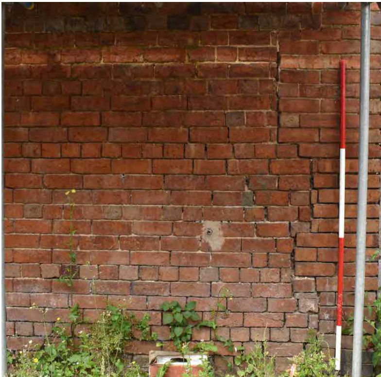
25 Change of brickwork at north-east corner
