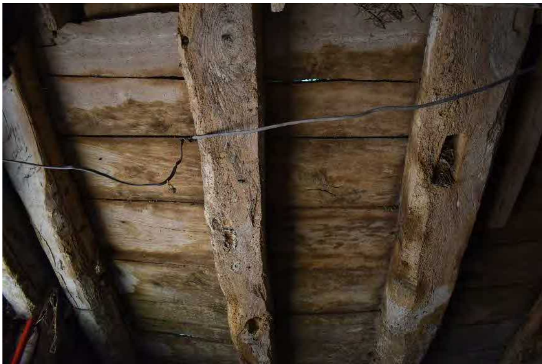
40 Old floorboards and re-used timbers for joists
