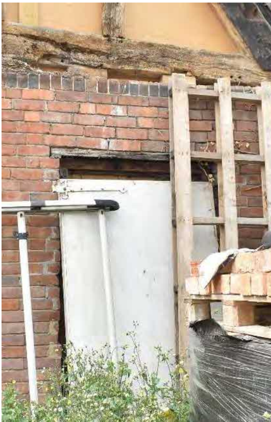
27 Inserted door on north gable wall
