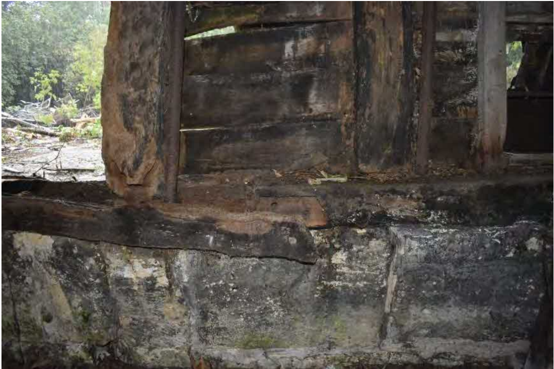
13 Half-jointed sill beam with face pegs
