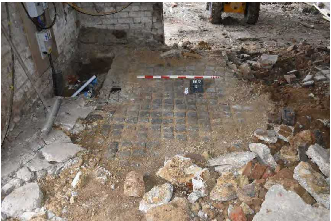
51 Brick 'setts' below concrete
