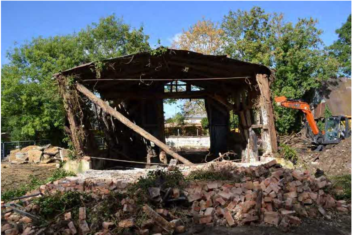
44 Start of demolition of barn
