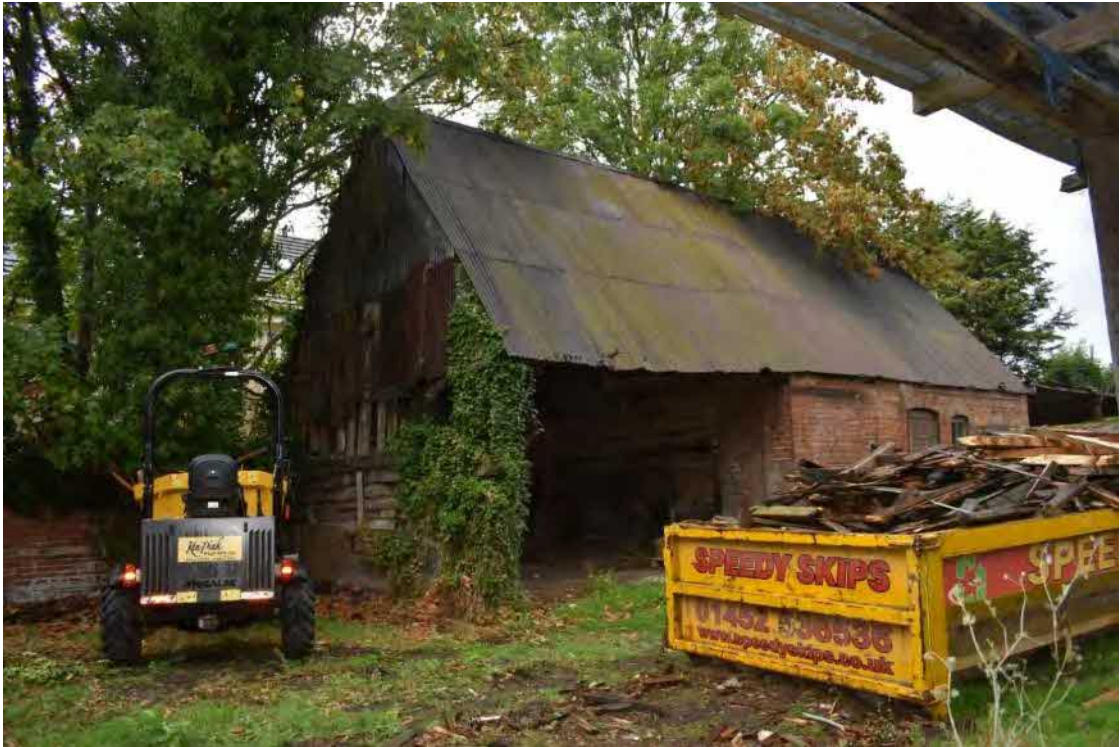
17 Building L, southern gable, September 2022
