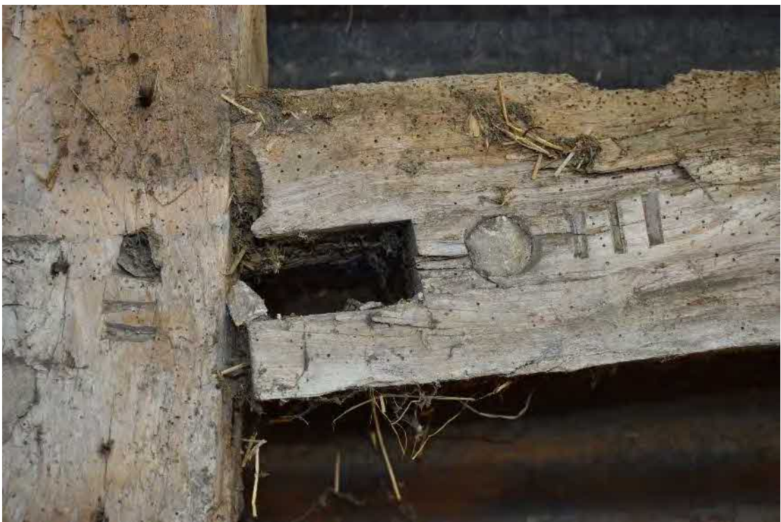
35 Carpentry marks III, infilled peg hole and open mortise
