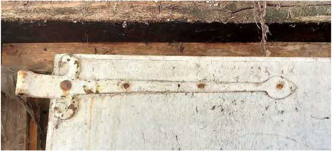
28 Old strap hinge on later north door
