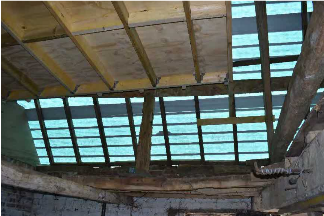
42 Modern bat roost above formerly floored area in north part of room, old timbers below
