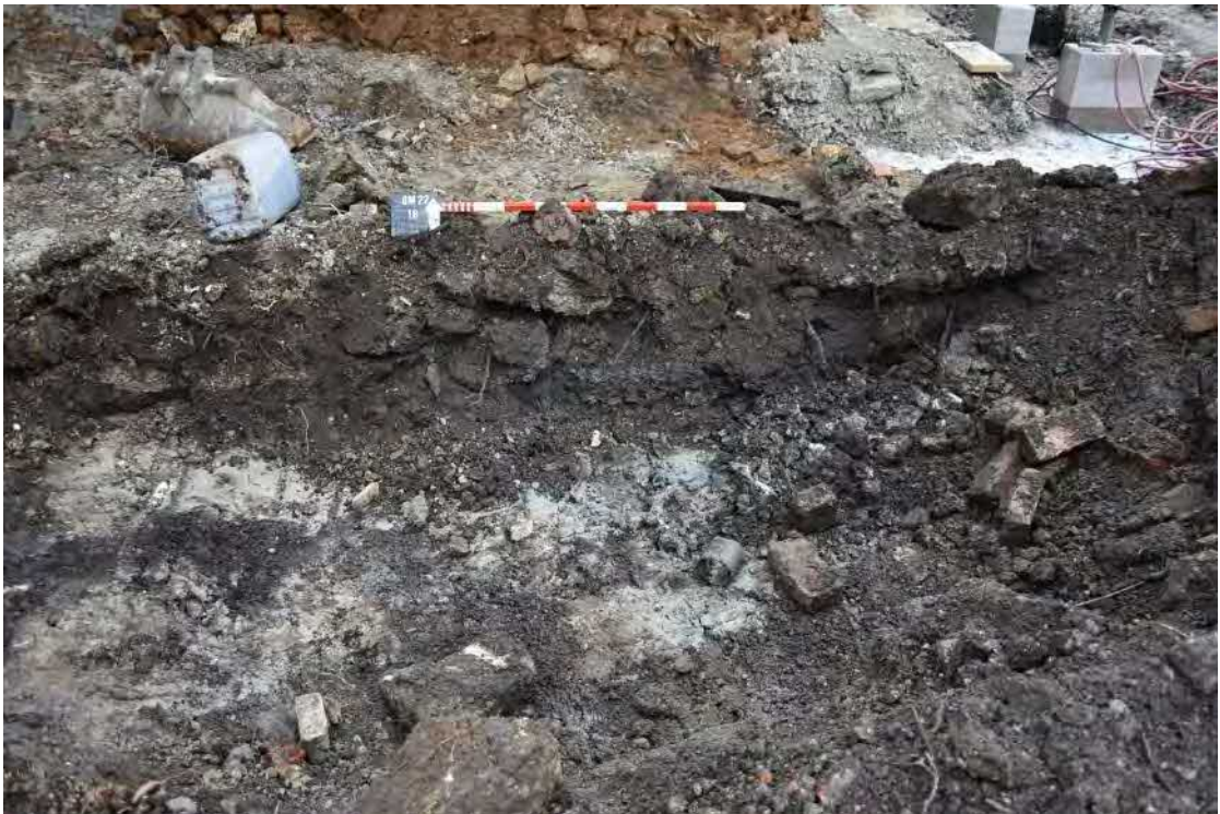
53 Trench excavated through contaminated ground to the south of Building L
