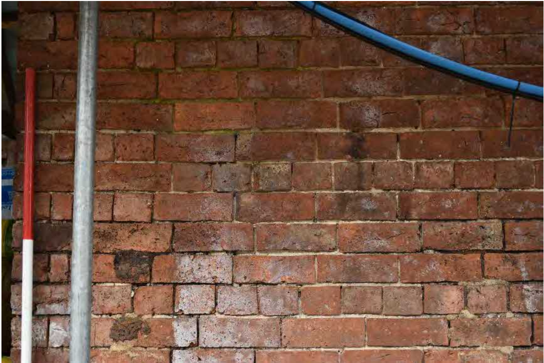
22 Detail of English Garden Wall Bond brickwork of east wall
