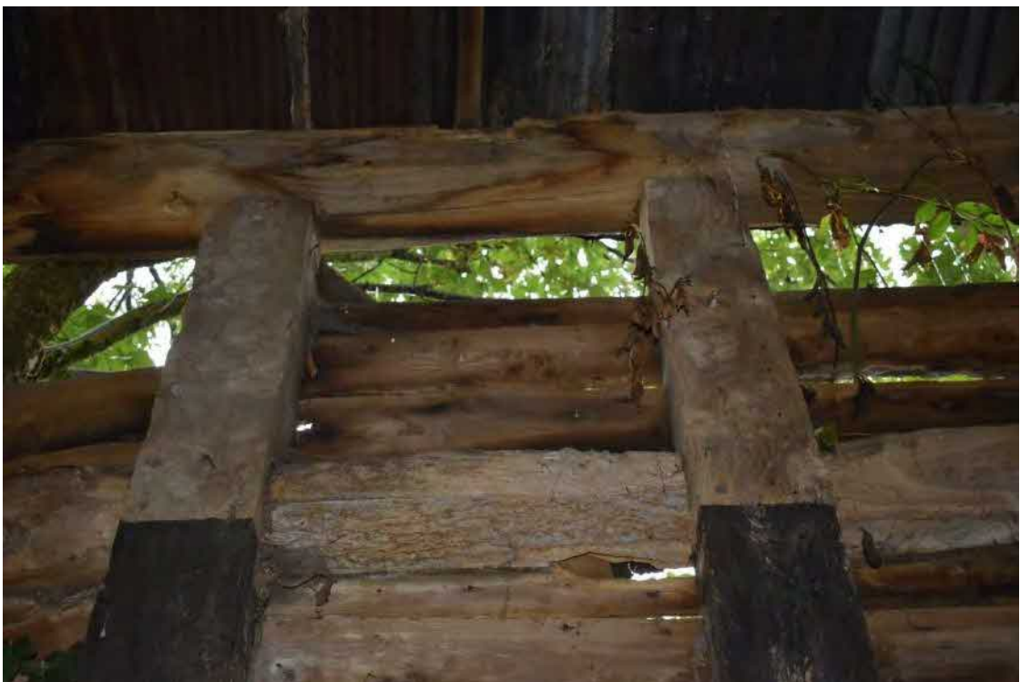
14 Underside of framing with bark below timber
