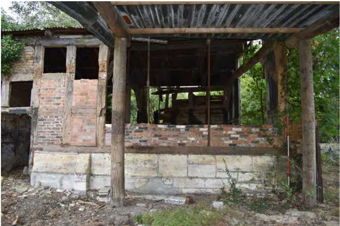
6 Area where timber framing has been replaced by iron poles and brickwork
