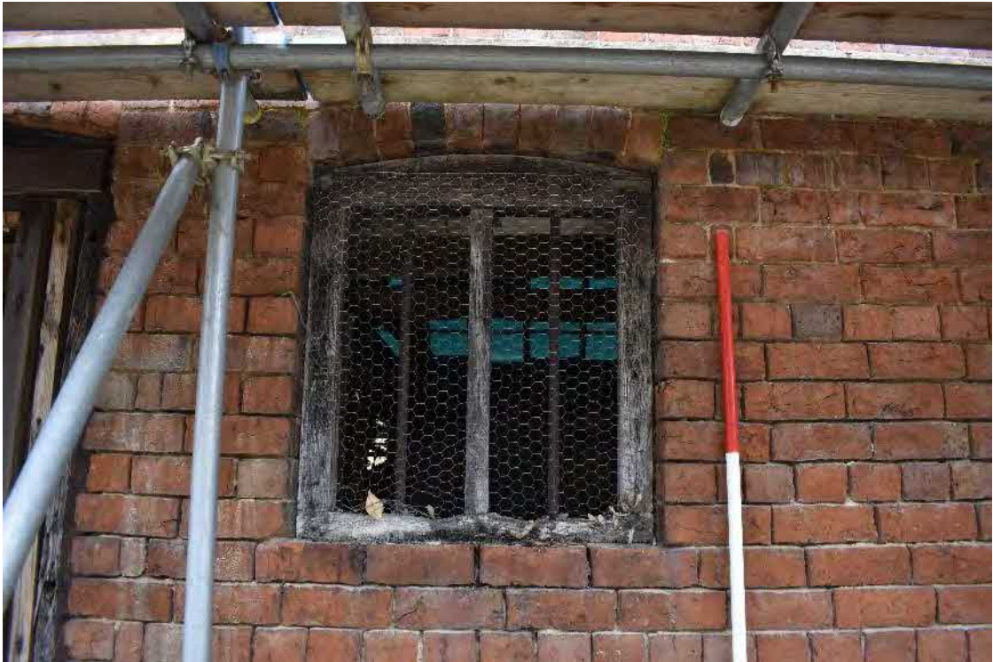
24 Window on east wall
