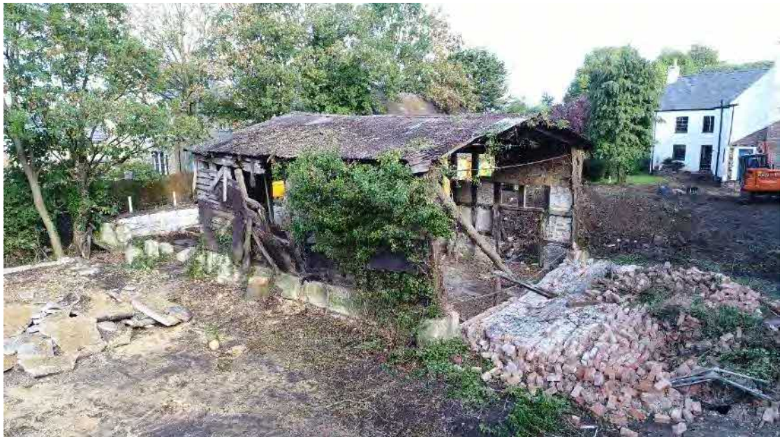
43 Drone shot of Barn prior to demolition
