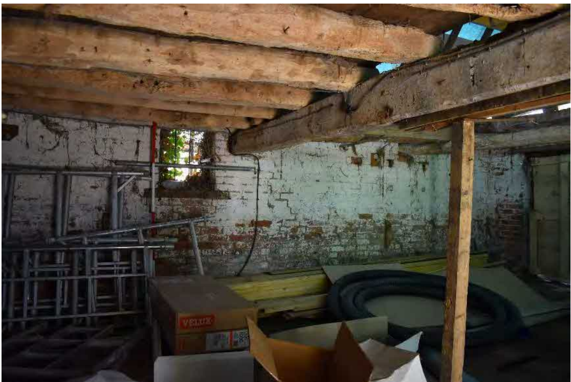
39 Chamfered girder and floor joists
