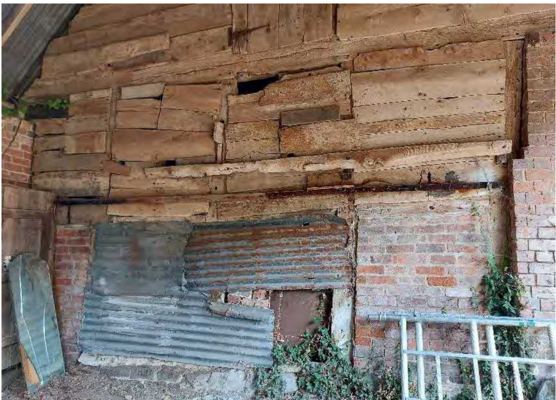
18 Internal wall with rough board and brick infill
