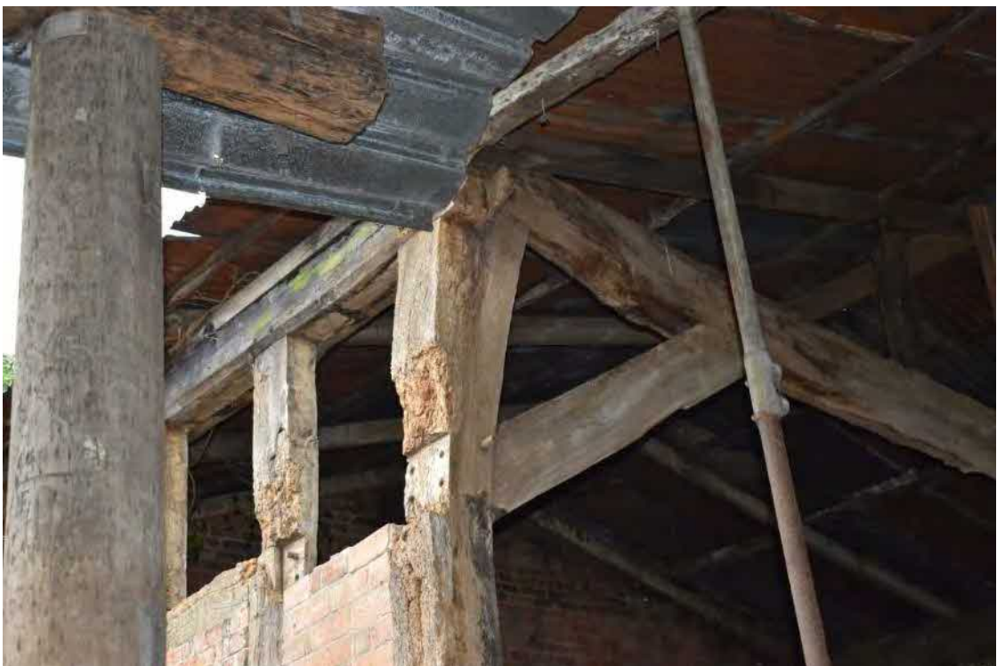
12 Timber framing with detail of halved joint, formerly face pegged
