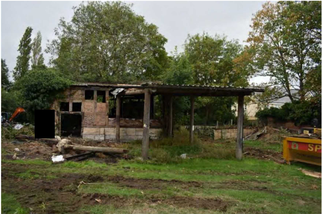
1 Timber-framed barn, north-east side, with pole barn in front
