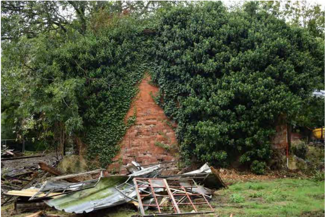
5 Brick gable, overgrown with ivy
