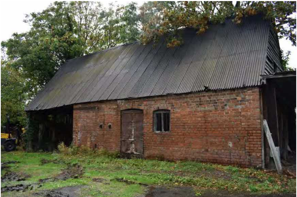
16 Front of Building L with weatherboarded north gable, September 2022
