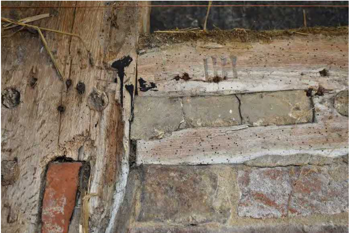
36 Carpentry marks IIII, mortises infilled with brick and mortar
