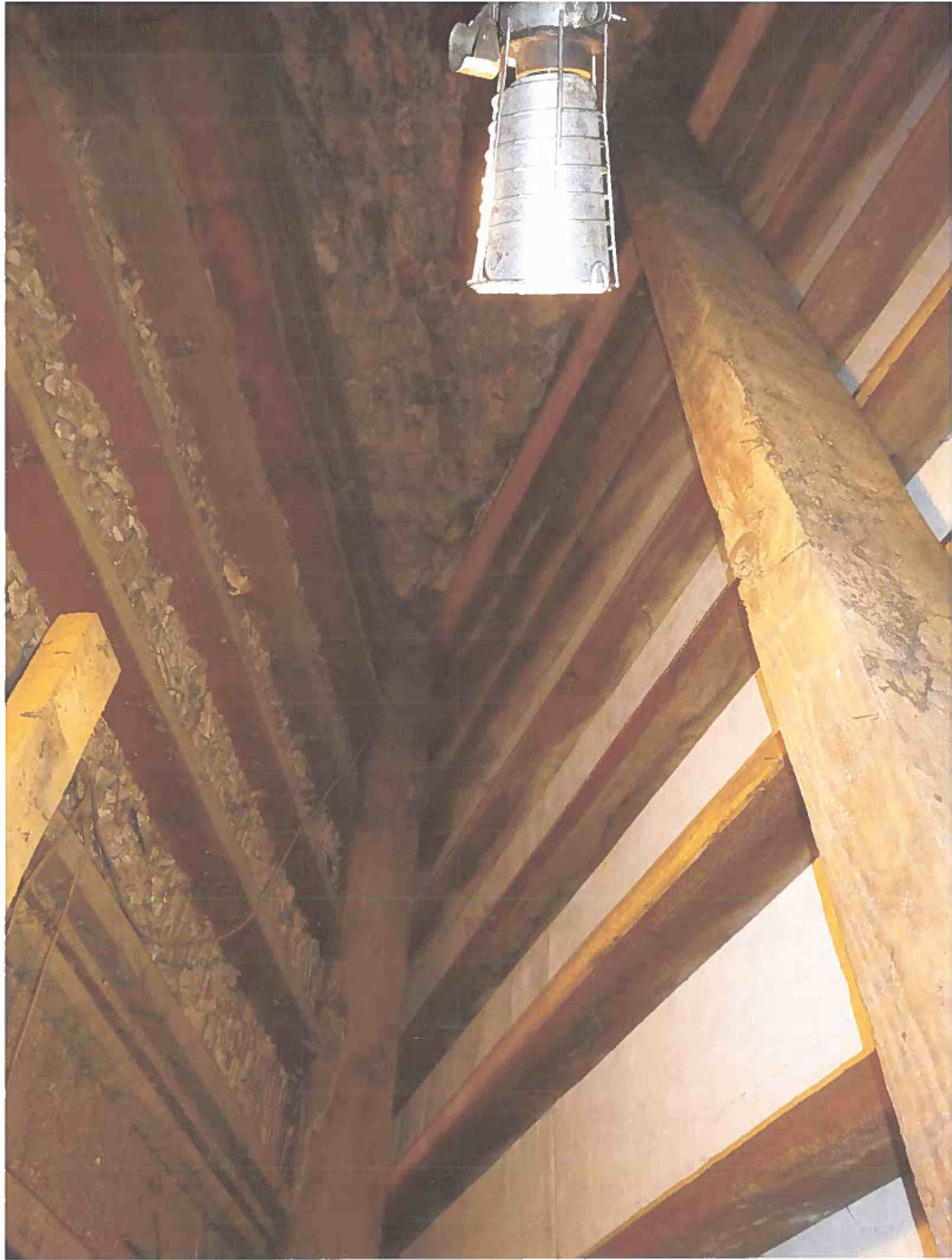
FIG 1. 30° PITCH ROOF, 2 PURLINS, REPLACED RAFTERS
