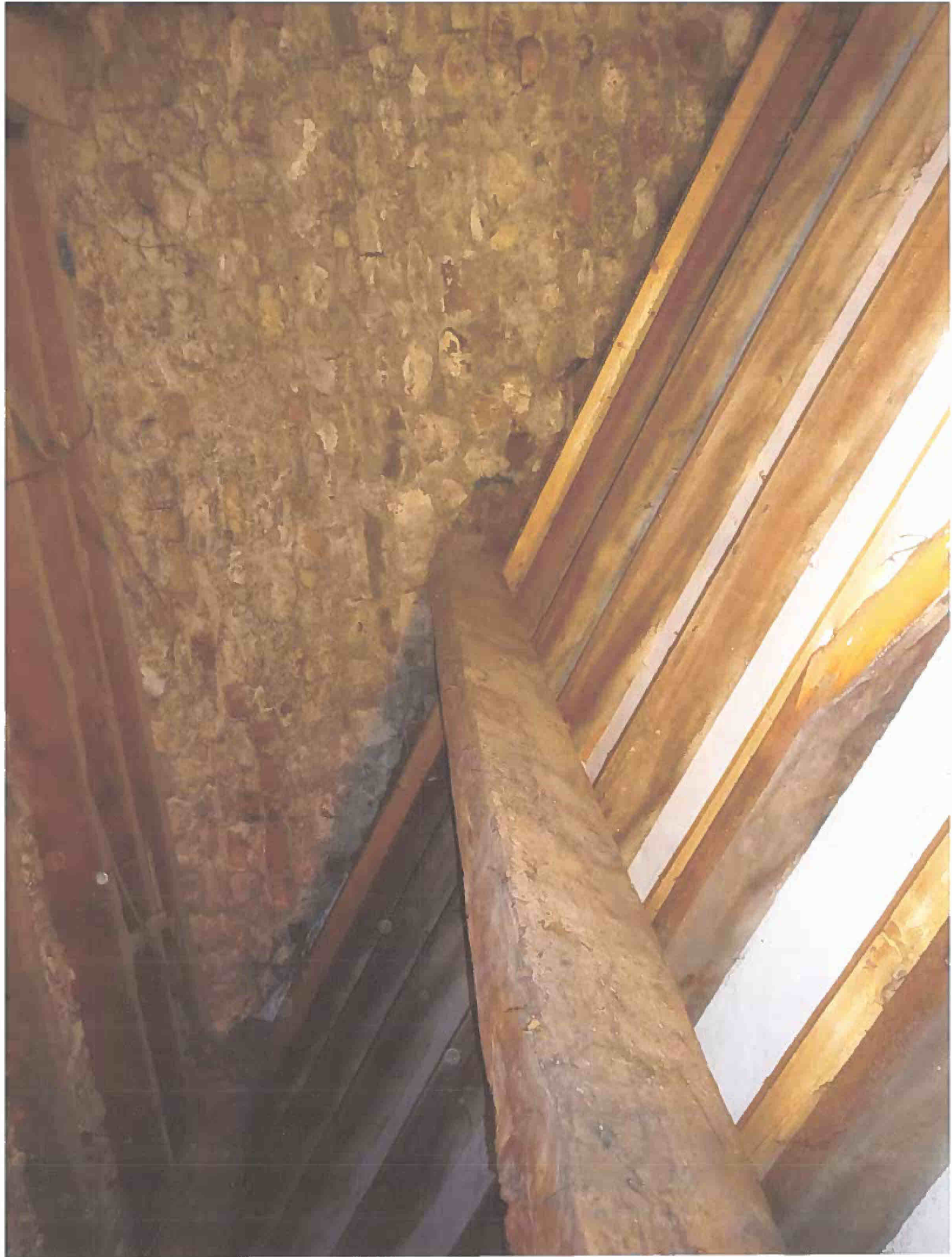
FIG 2. PRIMARY SUPPORT PURLINS 'BUILT IN' REPLACED RAFTERS
