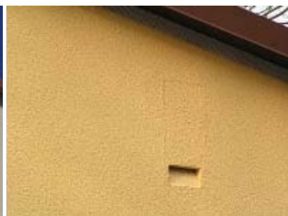
Schwegler 1FR Bat Tube, to be integrated into building wall, and either bricked in or rendered. Self cleaning. Dimensions: 47.5 x 20 x 12cm.
