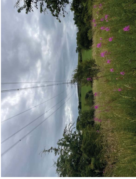
Plate 10: (looking south) Overhead lines crossing eastern section of site.
