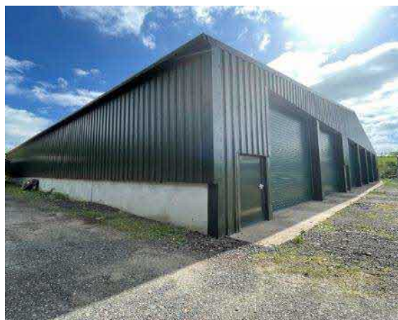
Photo 19: NW aspect of the shed
