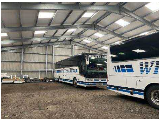
Photo 18: Internal view of shed
