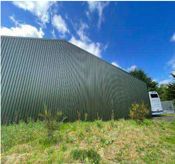
Photo 20: Back of shed
