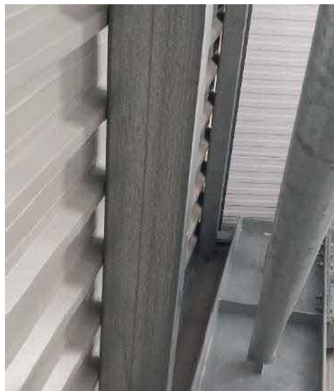
Photo 21: External light see at the top of the wall sheets
