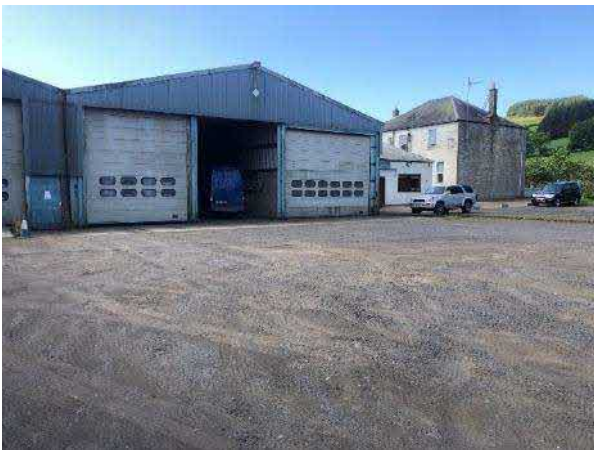
Photo 13: Offsite old bus shelters and office building (J3.6).
