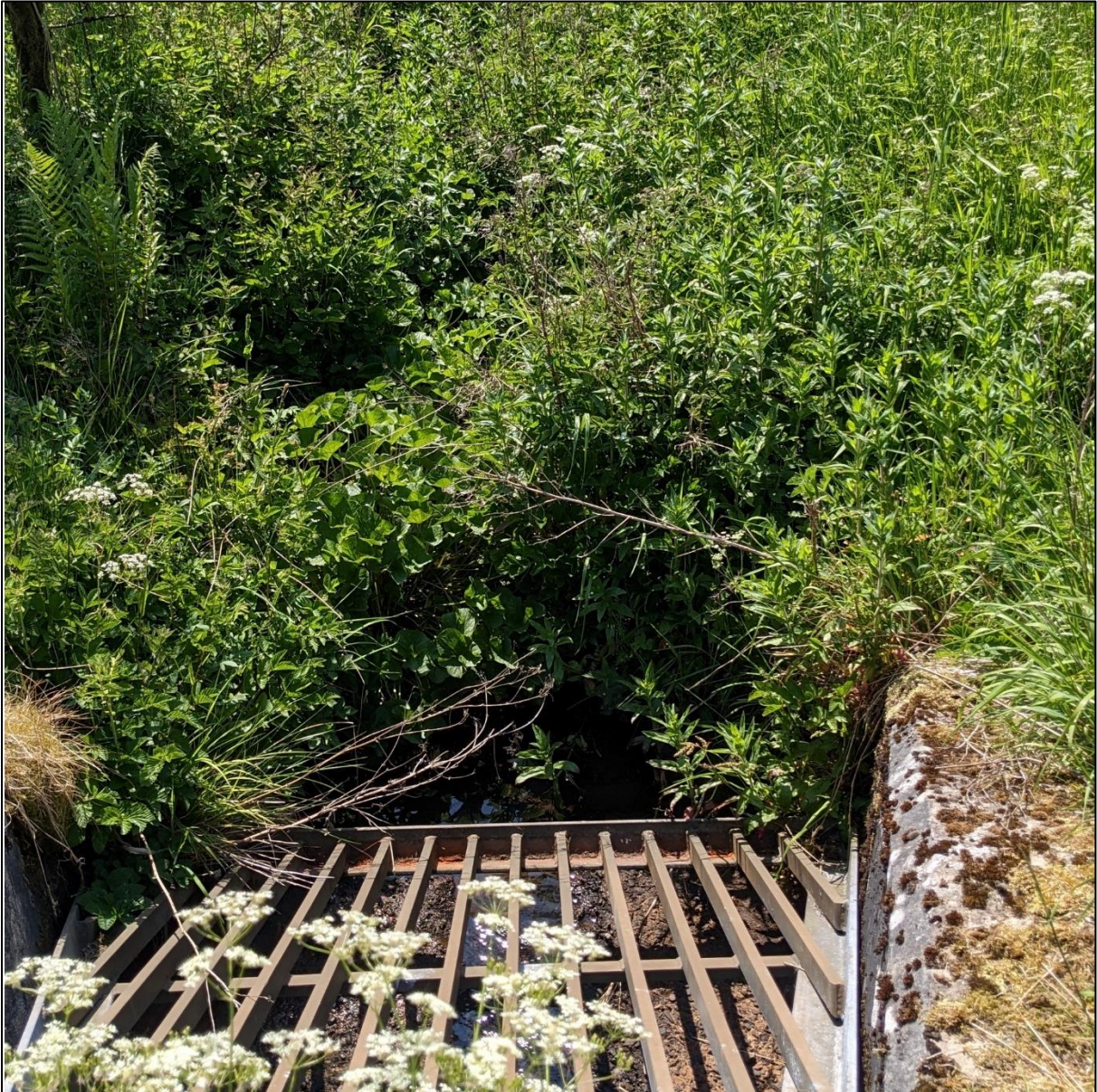
Photo 4: Unnamed Drain Flowing from Culvert Outlet into Site
