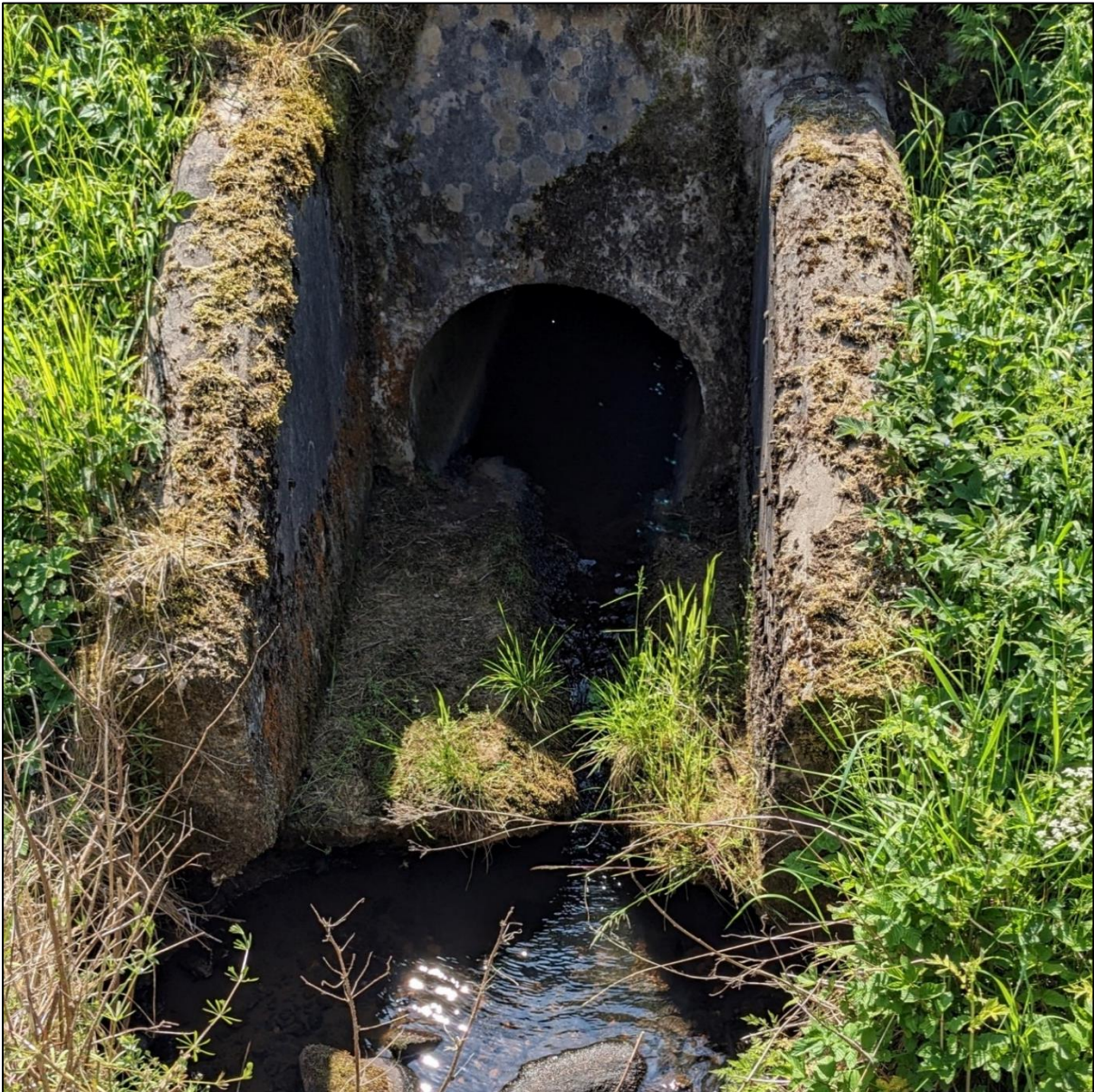
Photo 3: Culvert Inlet Under Road Immediately Upstream of Site
