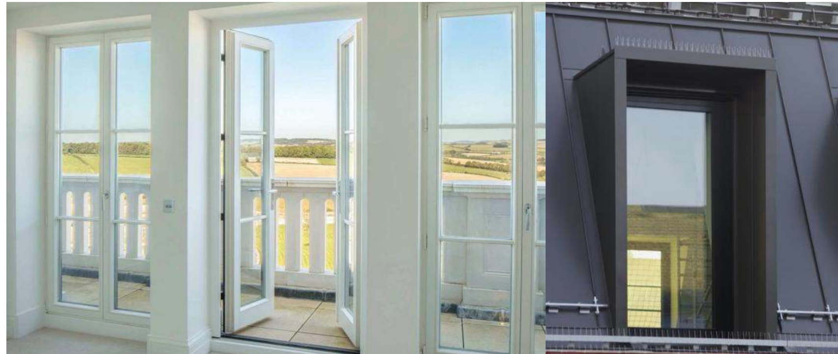
Above: French doors to terrace with precast stone balustrade
