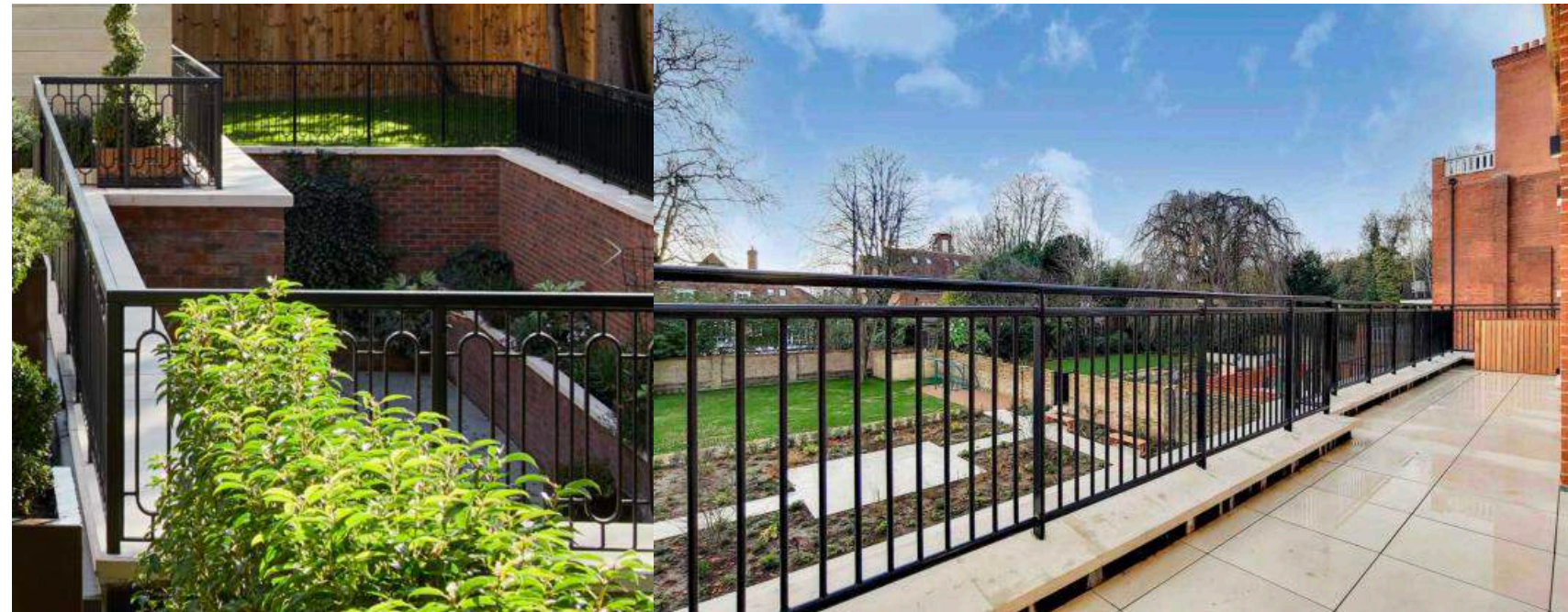
Above: Metal balustrade on low parapet to edge of terrace.
