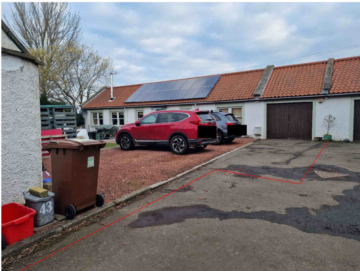
Image 3, showing property of 43 Main St. Image Facing North with approximate boundary line shown in RED.
