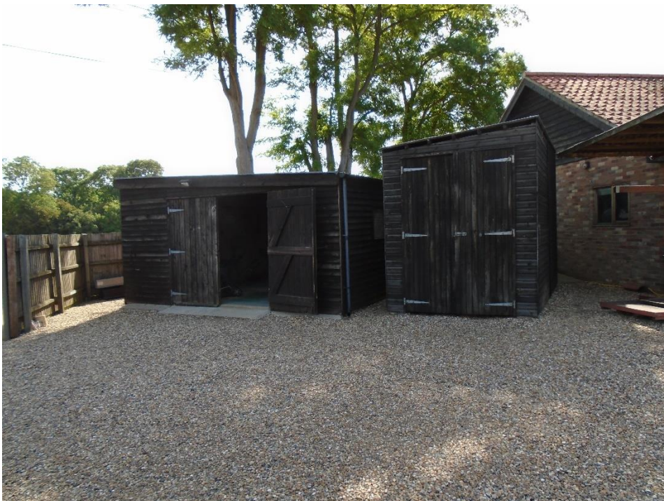
Photograph 4: Timber buildings at Royston Farm.
