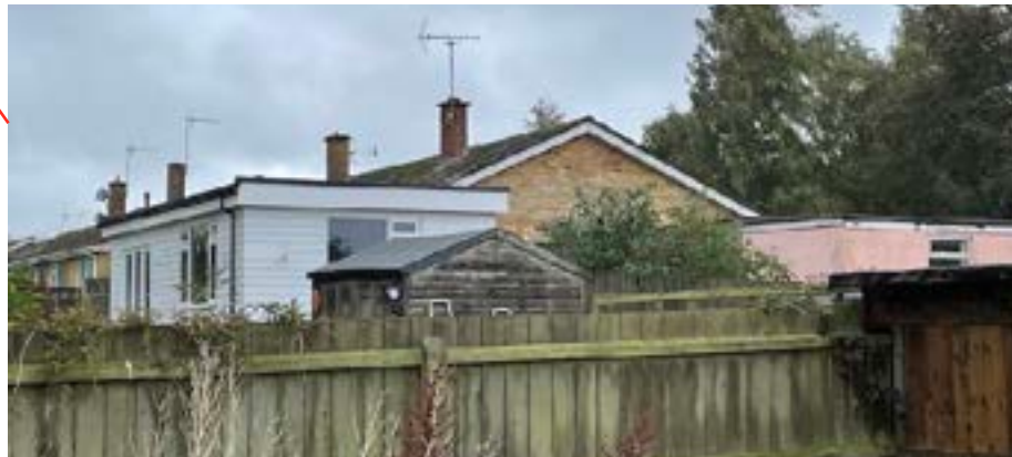
Figure 8 Recent extension to No 31
