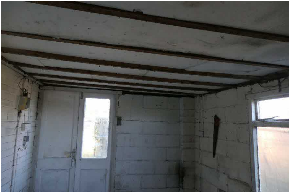
Photo 10, internal view of building two looking west.
