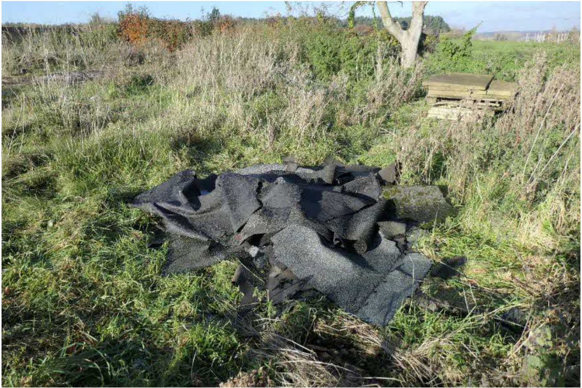
Photo 7, stacked materials on site.
