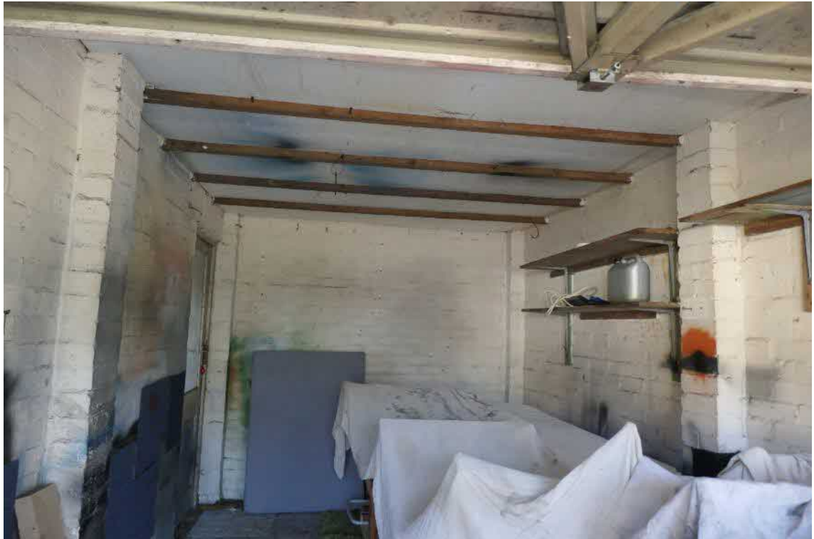
Photo 9, internal view of building one looking east.
