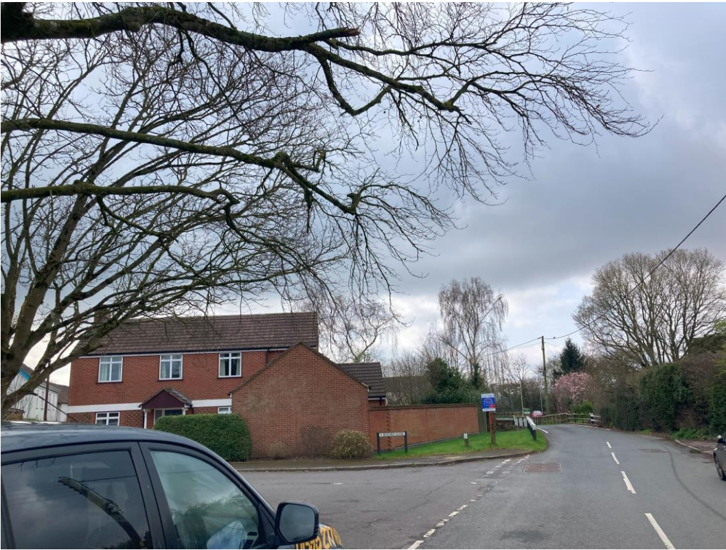
Photo showing crown lifting needed on T2
