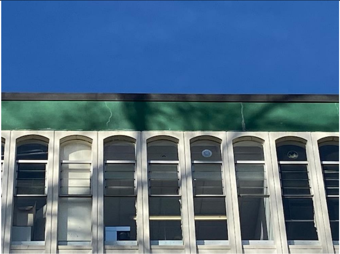
Building 4 – photo showing section of flat roof
