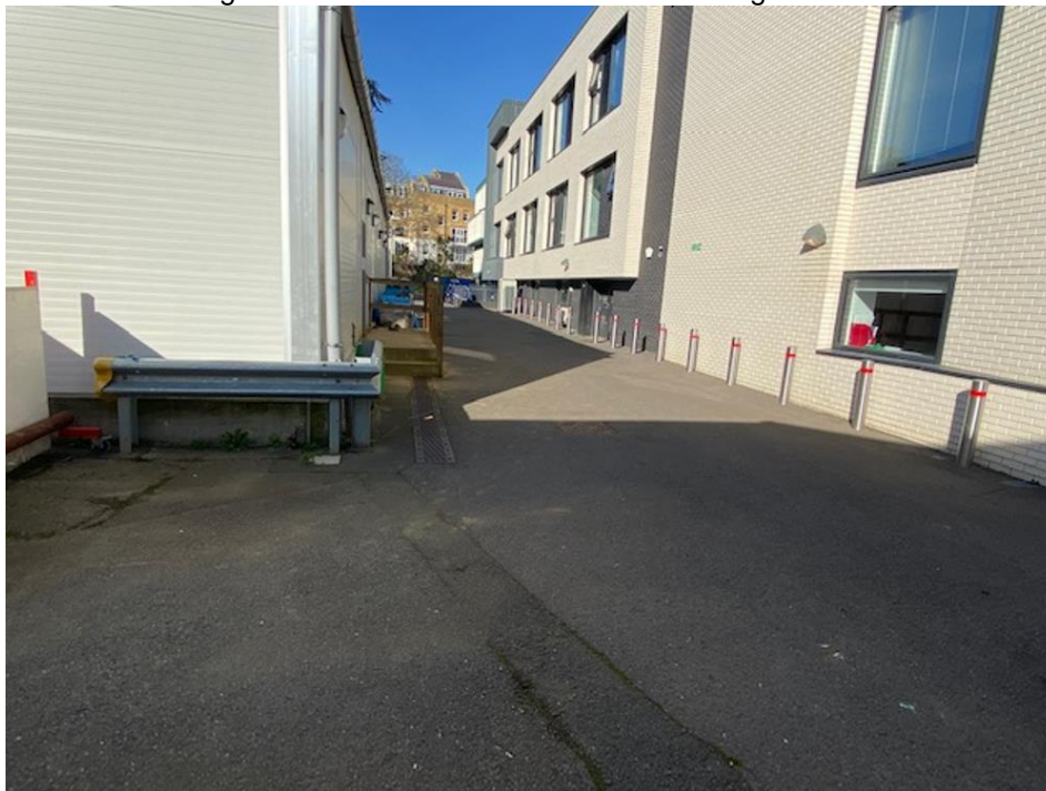
Photo showing hardstanding on site in centre of site
