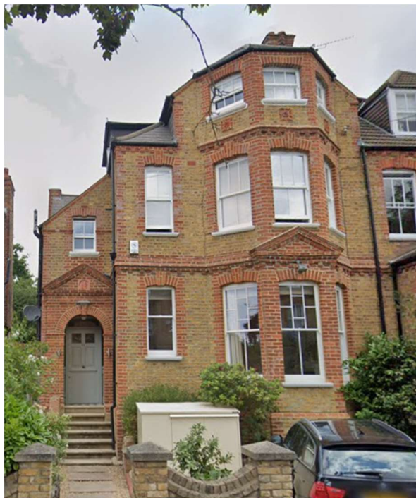
Fig.1- Front elevation of property
