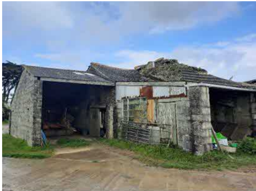
Figure 2: View of the eastern and southern elevations of Barn 2.
