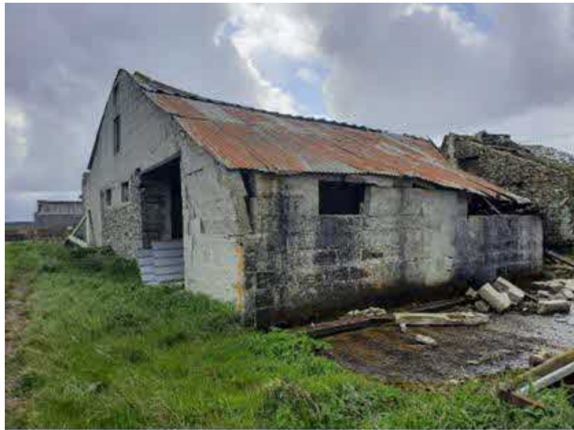
Figure 5: View of part of the block-built section on the northwest elevations of Barn 2.
