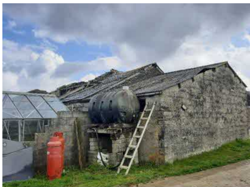
Figure 3: View of the southern and western elevations of Barn 2.
