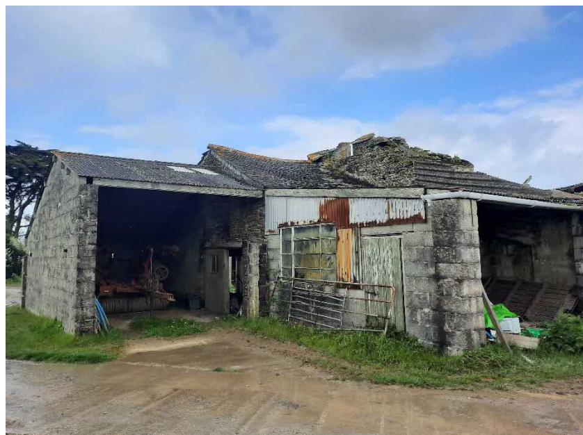
Figure 4: View of the eastern and southern elevations of Barn 2.
