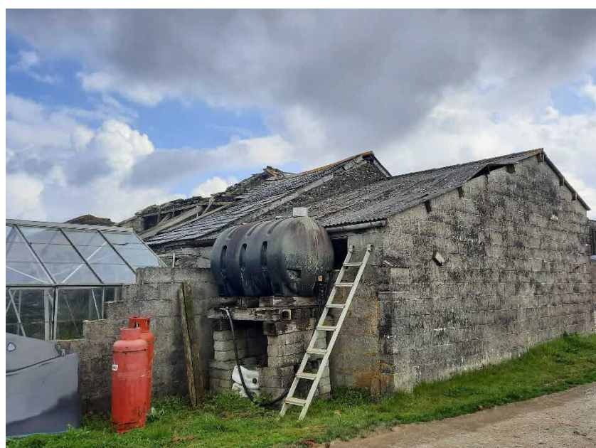
Figure 5: View of the southern and western elevations of Barn 2.
