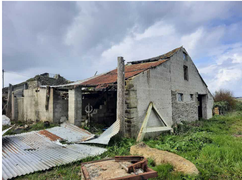
Figure 8: View of part of the block-built dilapidated section on the northeast elevations of Barn 2.
