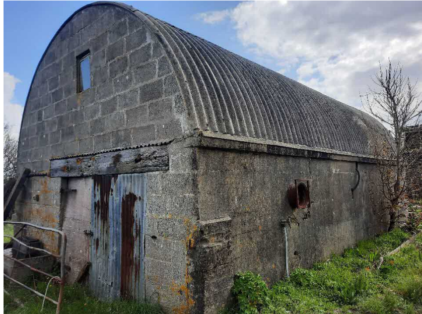
Figure 2: View of the south and western elevations of Barn 1.
