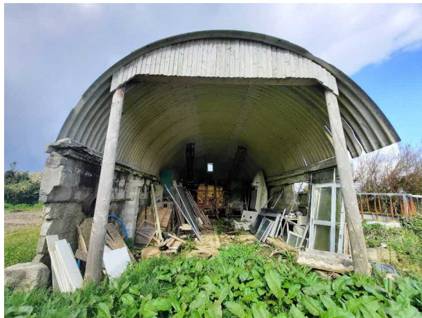
Figure 3: View of the open nature of the eastern elevation of Barn 1.
