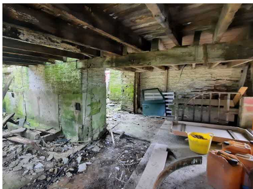
Figure 12: Internal view of part of the block-built section in Barn 2.
