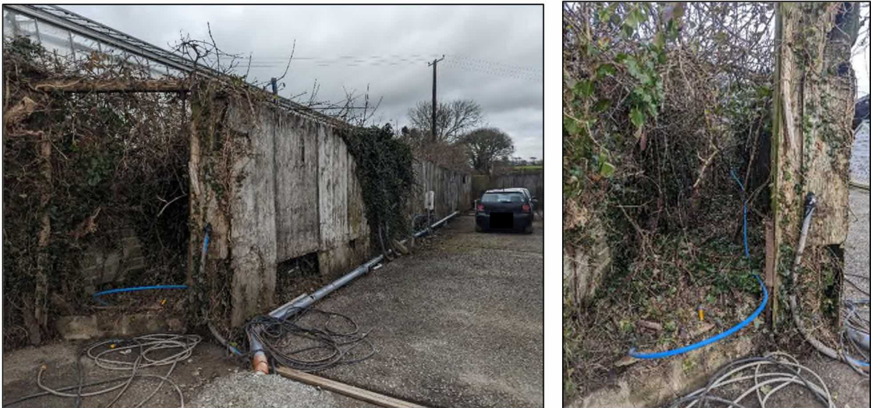
Figure 3: linear scrub habitat formed between wooden panel fence and boundary wall.
