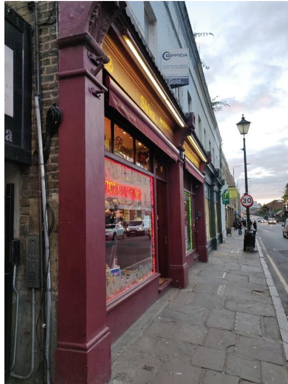
P09- Shiva- LED strip light above fascia signage
