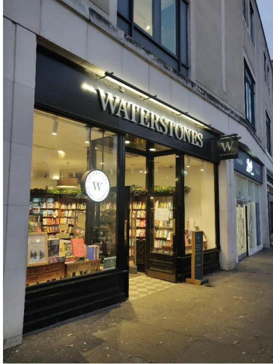
P01- Waterstone – LED strip light above fascia signage and projecting signage
