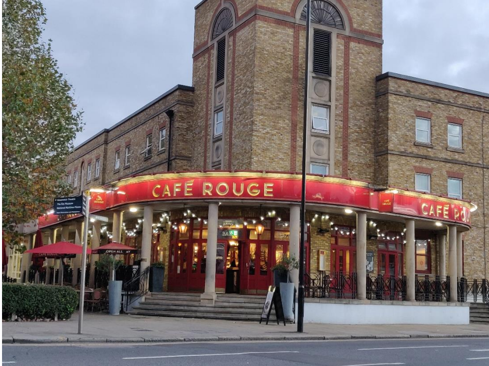
P03- Café Rouge – LED strip light above fascia signage and projecting signage
