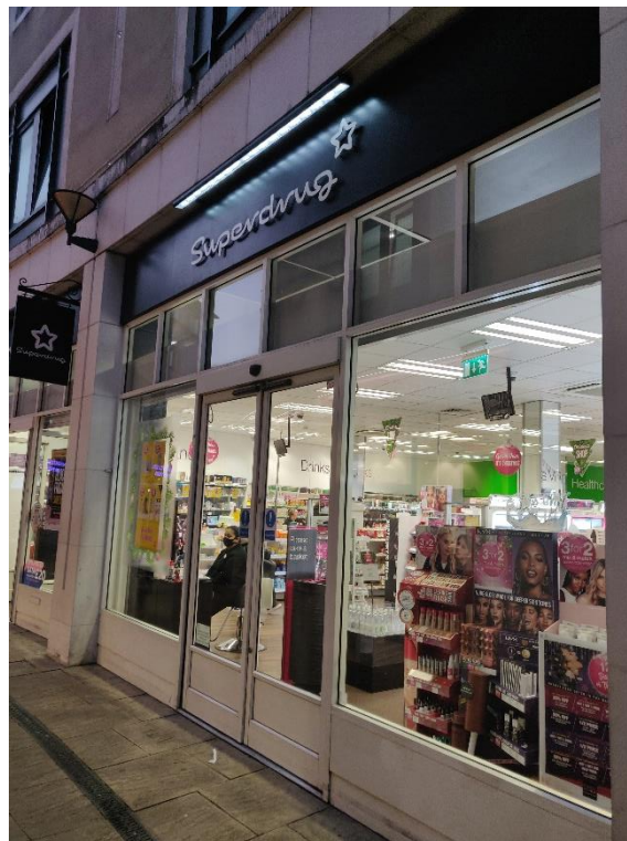
P08- Superdrugs– LED strip light above signage
