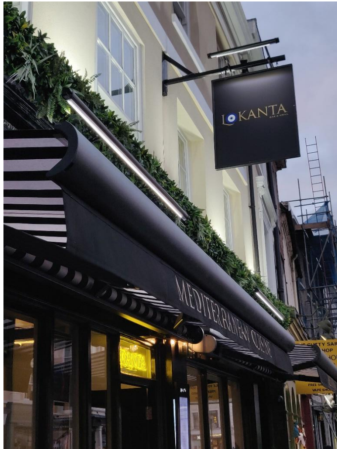
P05- LED strip lights above fascia signage and projection signage
