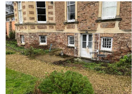
Photo 6. The front elevation which has a shallow lightwell and access into the lower ground floor accommodation.
