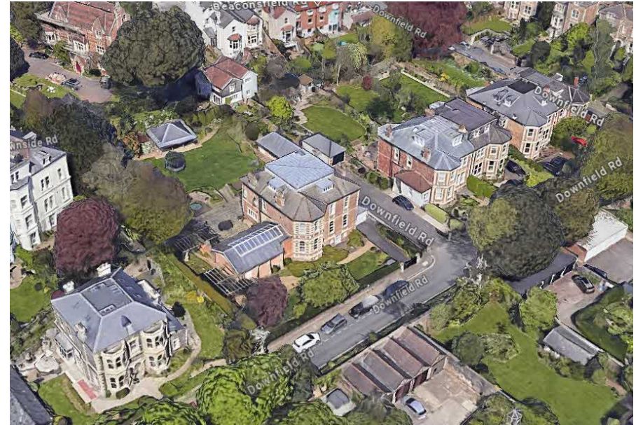
Figure 3. No. 3 Downfield Road seen in context with its modern clerestory roof and southwest side extension (c.1998).
