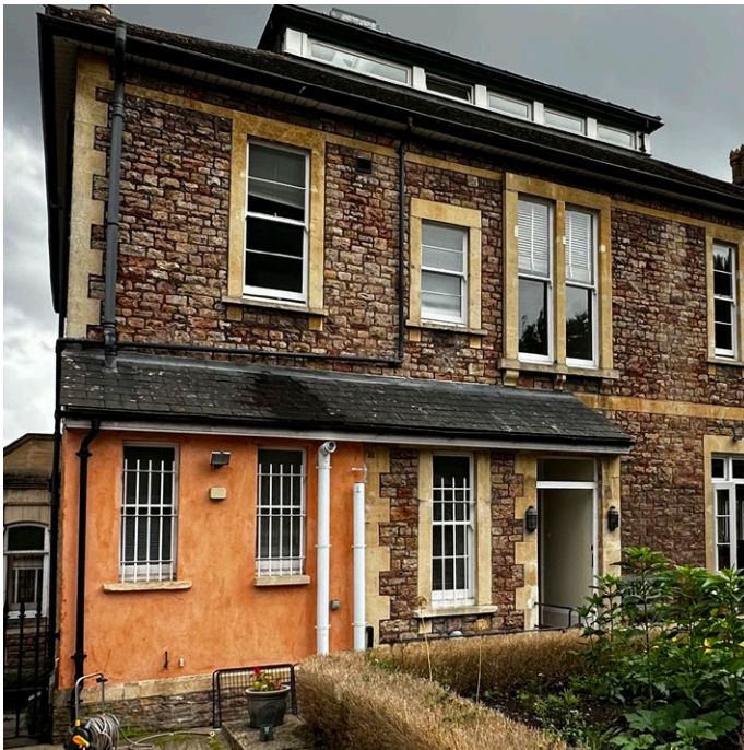
Existing rear extension of differing materials and detail.
