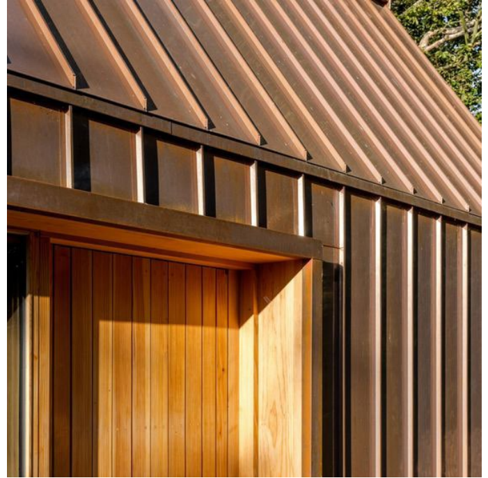
Proposed Copper Standing Seam Cladding. The deep brown non-uniform colour has been selected to reflect the brown stone of the existing house.
