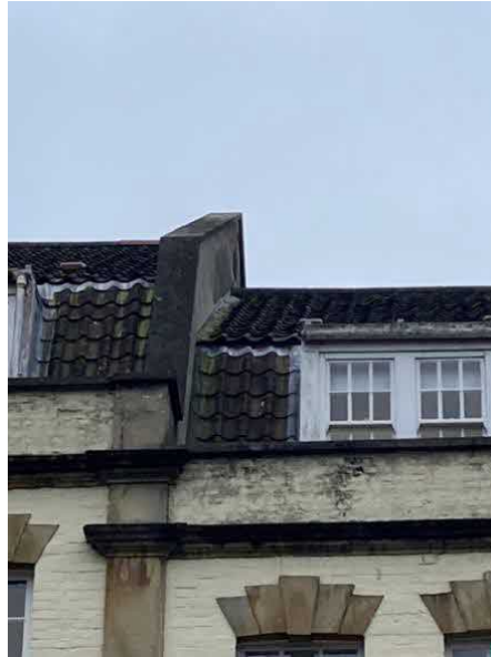
Figure 9 - Party Wall between 9&10 Upper Berkeley Place
