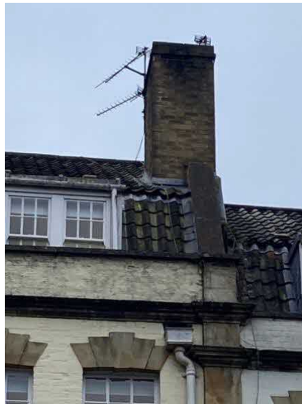
Figure 10 - Chimney to 9 Upper Berkeley Place
