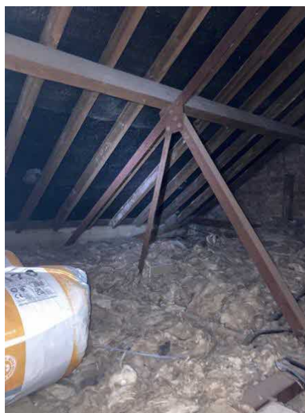
Figure 14 - Roof Void to 9 Upper Berkeley Place
