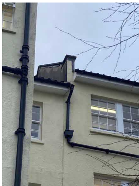
Figure 11- Rear Elevation of 10 Upper Berkeley Place
