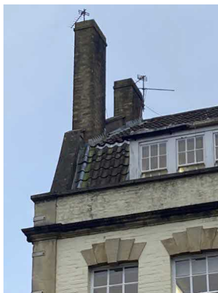
Figure 8 - Chimney to 10 Upper Berkeley Place
