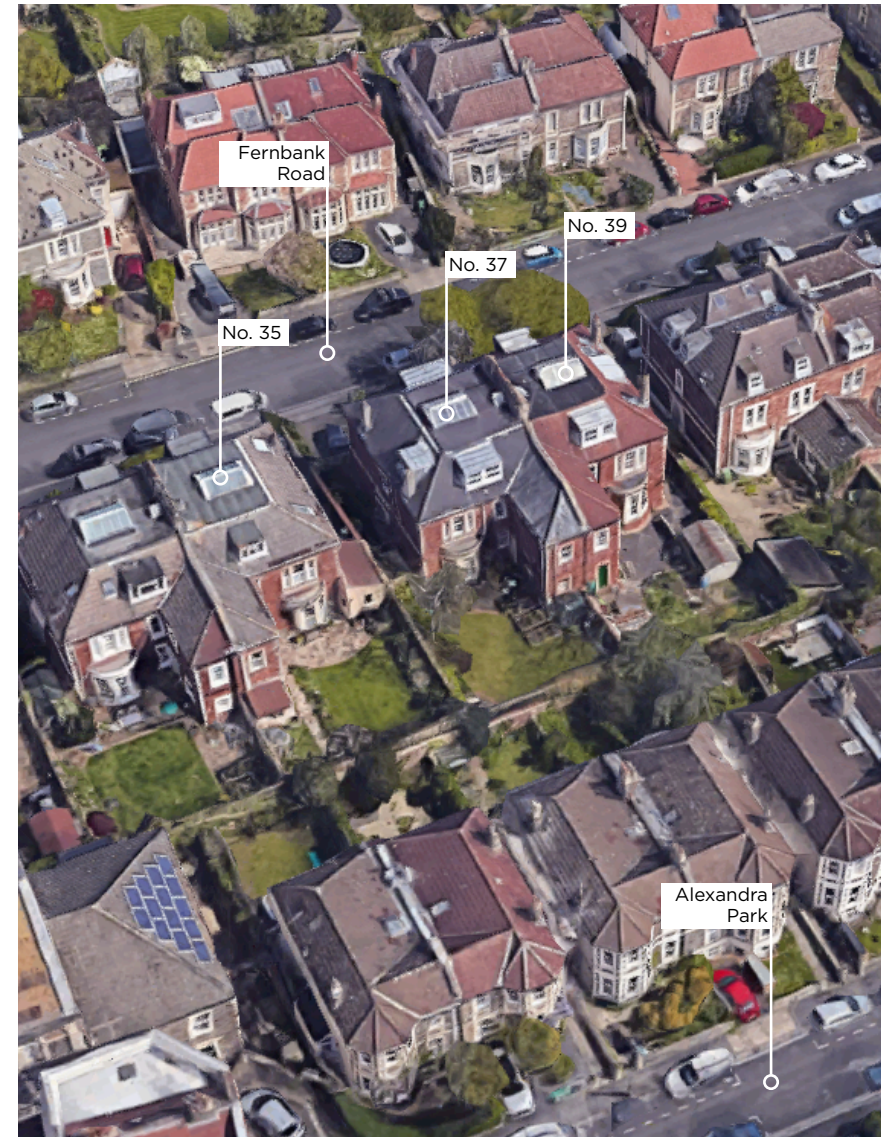
Aerial view of site & context
