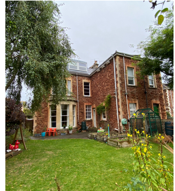
Existing property from rear curtilage
