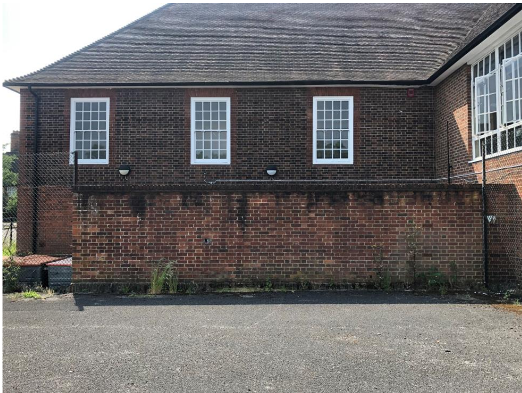
External view of the existing rear wall
