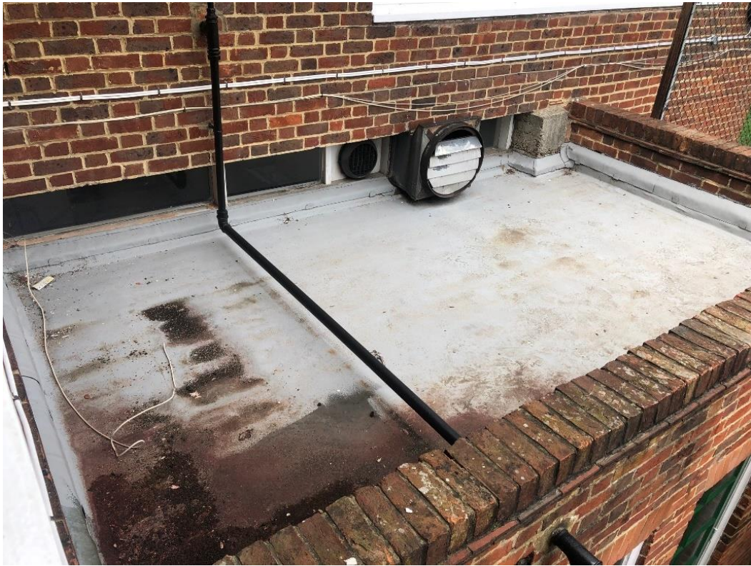
External view of the existing flat roof
