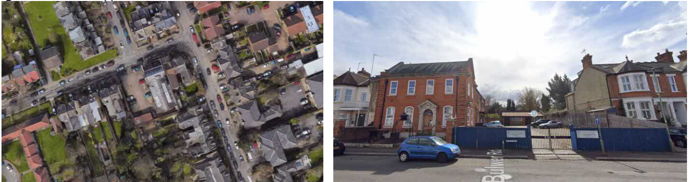
Figure 1. Views of Application Site
